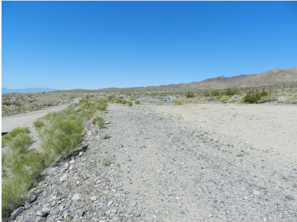
Figure 5. Overview of Cottonwood Springs Siphon. Facing West.
