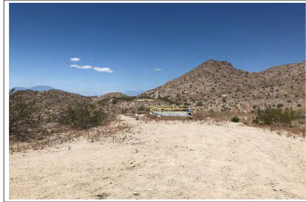
Photograph 6: View to the west of Mecca No. 1 Siphon [Work Area 7].
