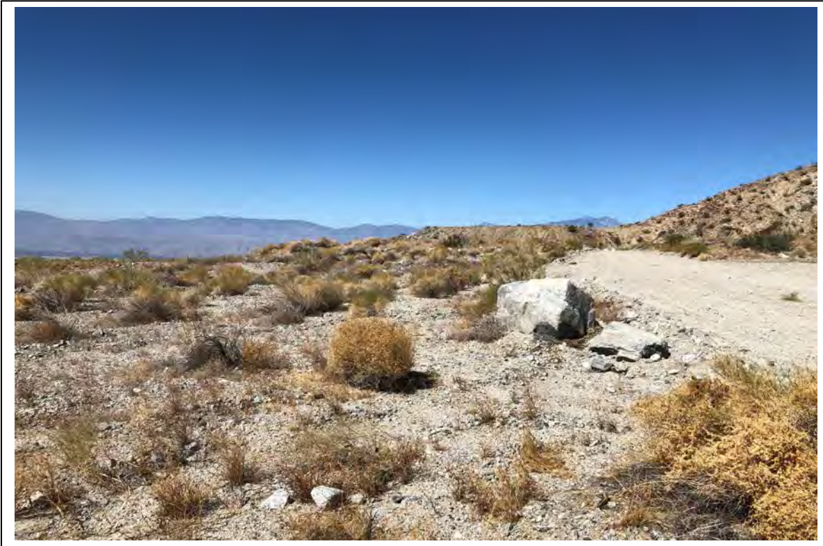
Photograph 15: View to the southwest of West Fan Hill Siphon [Work Area 14].
