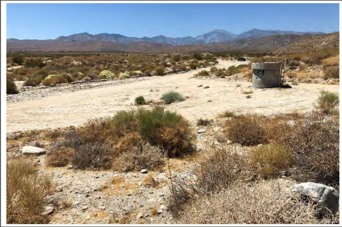
Photograph 21: View to the west of Big Morongo Siphon [Work Area 24].
