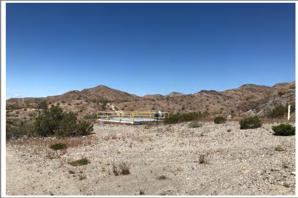
Photograph 1: View to the northwest of East Cottonwood No. 1 Siphon [Work Area 4].
