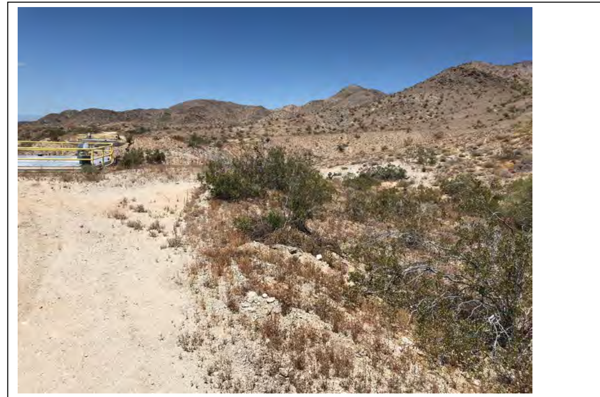
Photograph 12: View to the northwest of Iron Ledge Siphon Work Area 9].
