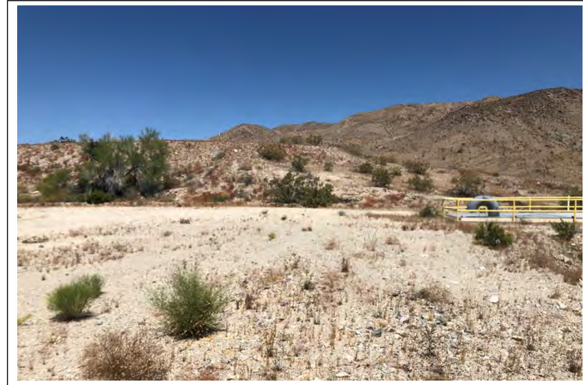
Photograph 8: View to the northeast of East Cottonwood No. 2 Siphon [Work Area 5].
