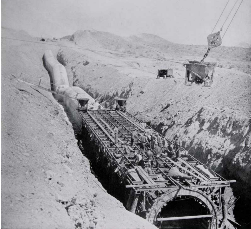
Figure 2. Monolithic Siphon Construction (MWD 1941)
