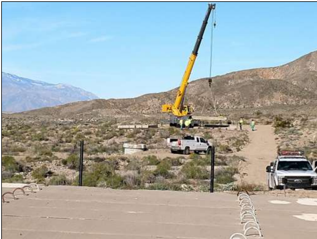
Figure 1-2. Mobile Crane Removing Transition Structure Cover
