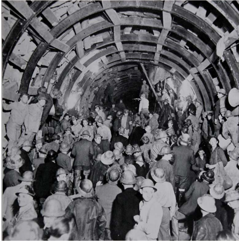
Figure 3. Final holing of the 13-mile San Jacinto Tunnel (MWD 1941)
