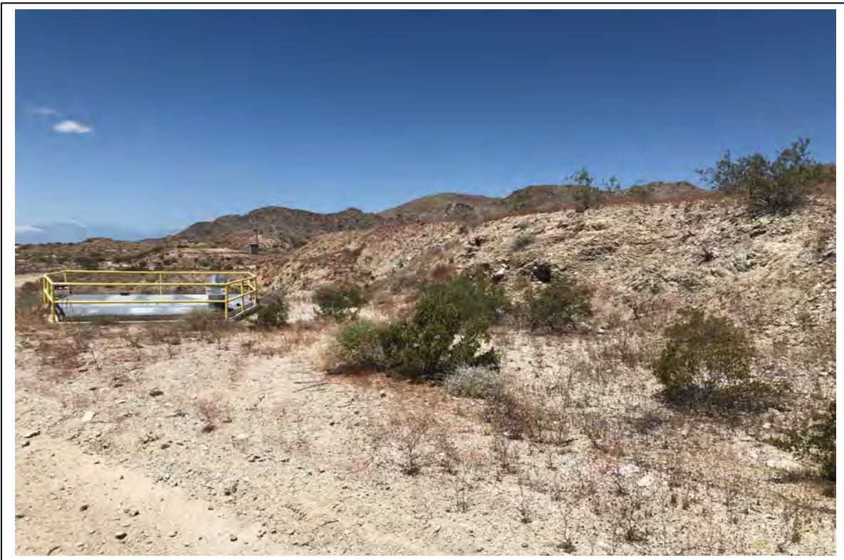
Photograph 11: View to the northwest of East Thermal Siphon [Work Area 10].
