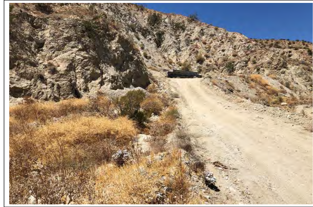
Photograph 22: View to the northwest of Whitehouse Siphon [Work Area 23].
