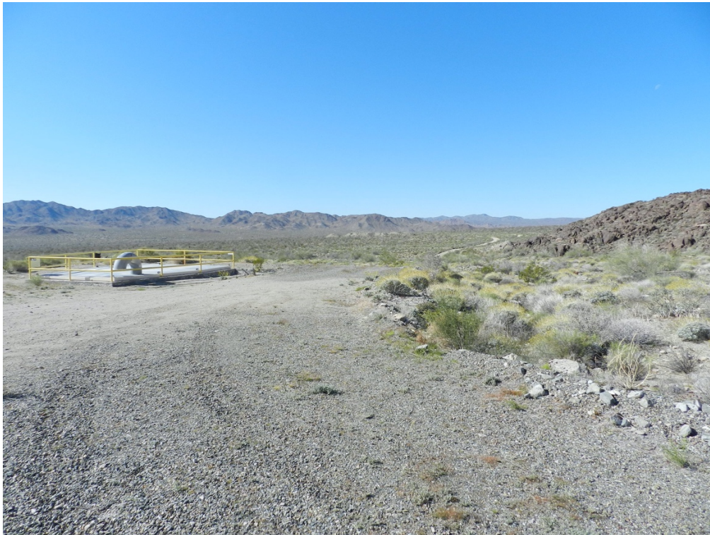
Figure 6. No Name Siphon East. Facing Southeast.
