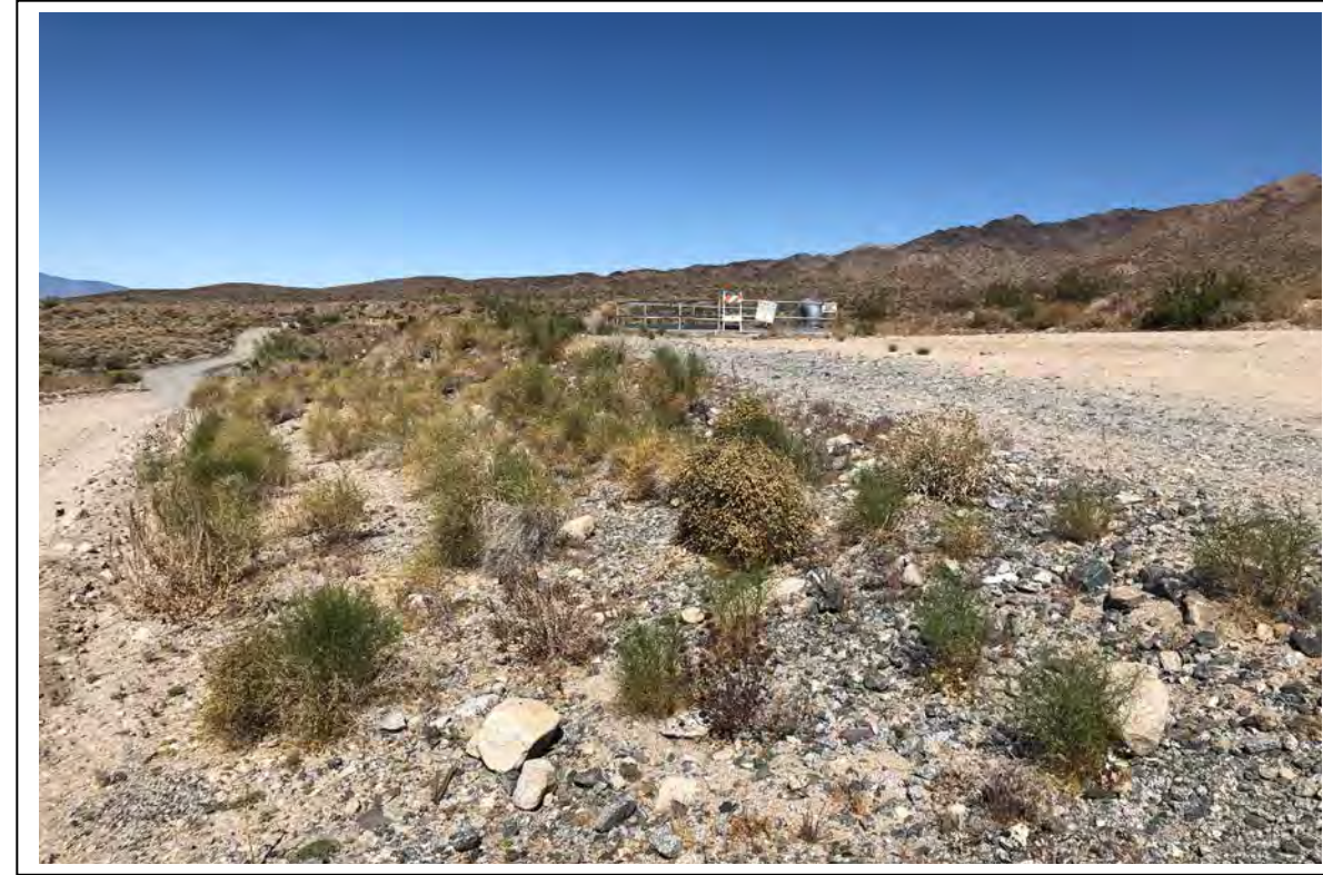
Photograph 2: View to the west of Cottonwood Springs Siphon [Work Area 3].
