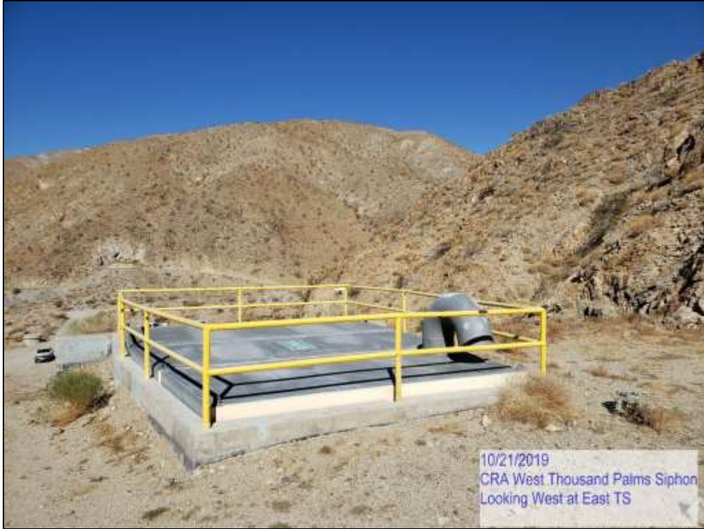
Figure 1-1. Transition Structure at West Thousand Palms Siphon
