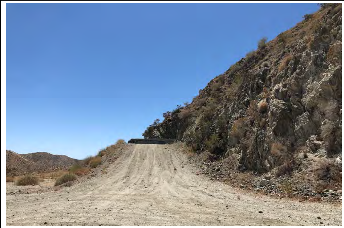
Photograph 23: View to the south of Little Morongo Siphon [Work Area 22].
