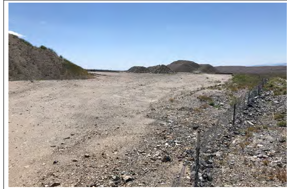
Photograph 26: View to the south of the proposed storage stockpile/sorting area located near End Wash Siphon [Work Area 6].
