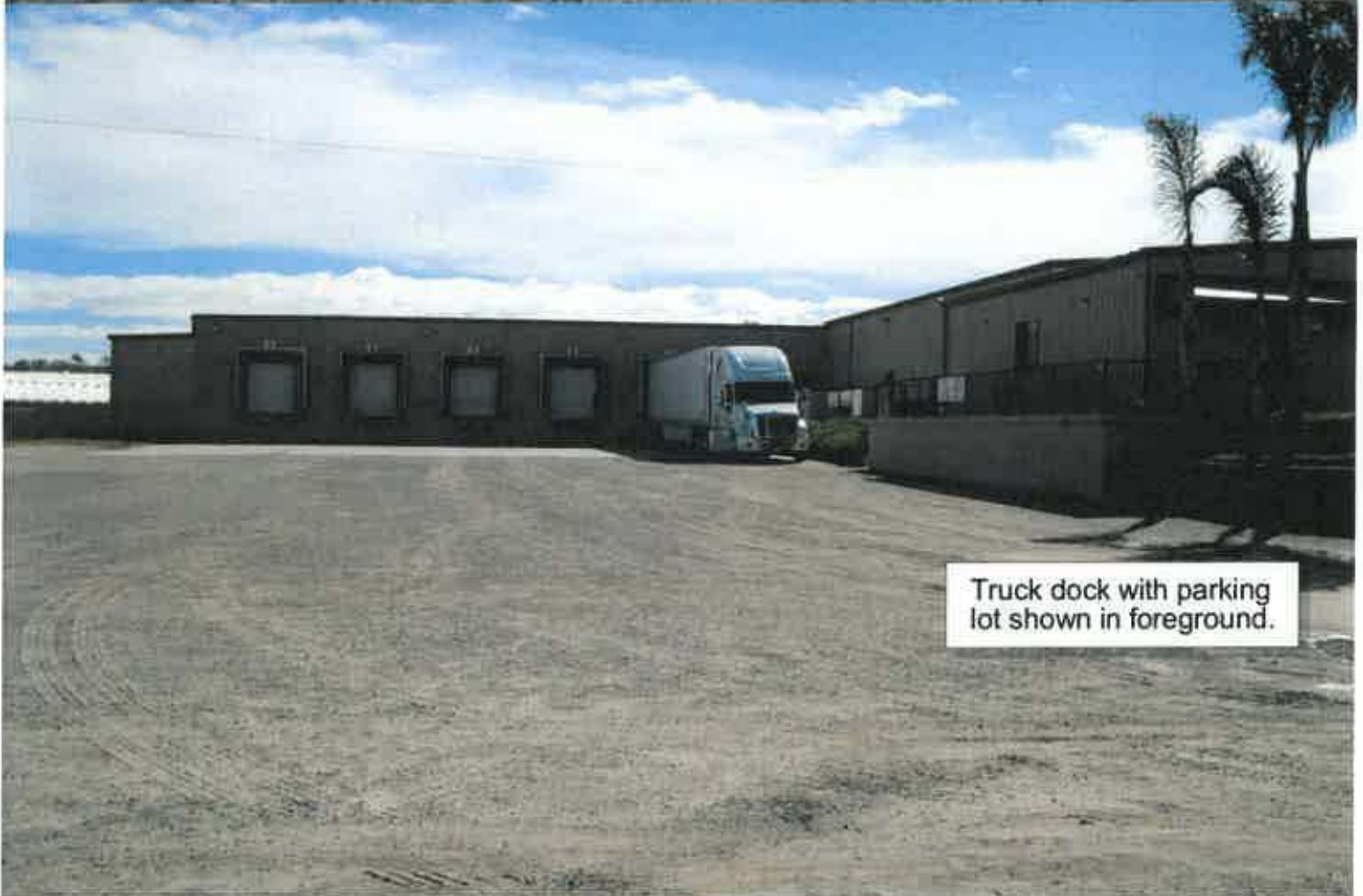
East side of plant.
