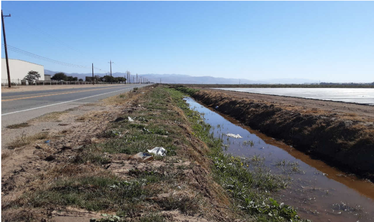
Photograph 9. Vegetated irrigation within drainage in the western portion of the extended Study Area, photograph taken facing east. 10/13/2021
