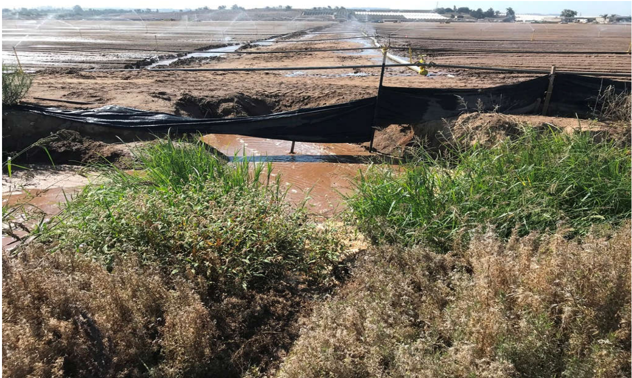
Photograph 3. Active irrigation input to vegetated irrigation drainage, photograph taken facing south. 09/23/2020
