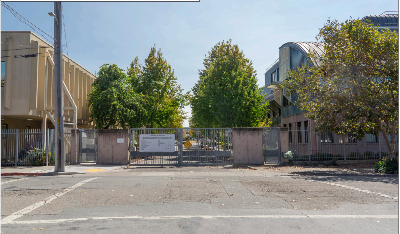
Existing View 10 from Aquatic Park (east side trails) looking East
