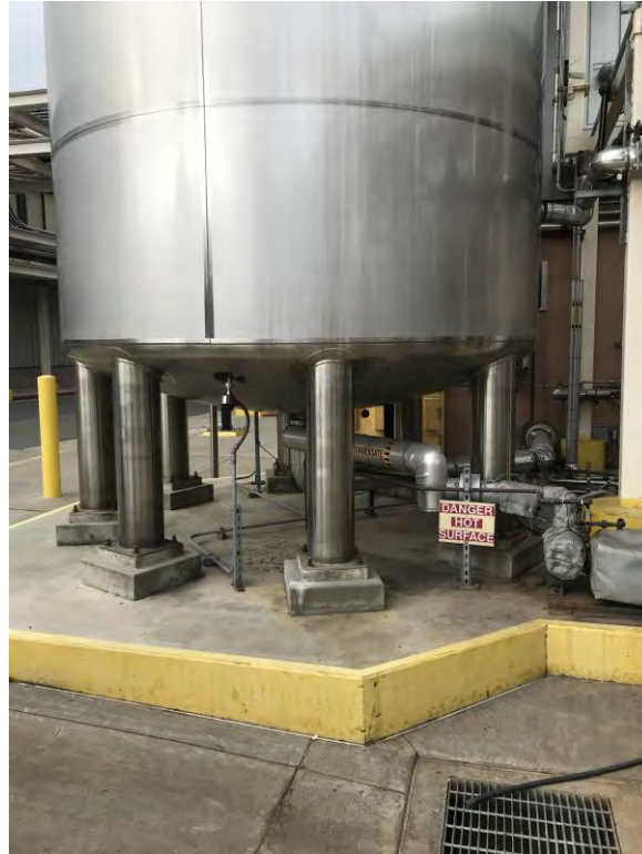
Photograph 3: Water treatment system and storm drain on exterior of building B66 on Parcel 1.
