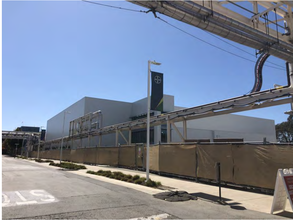
Photograph 17: Building B68 under construction on Parcel 2.
