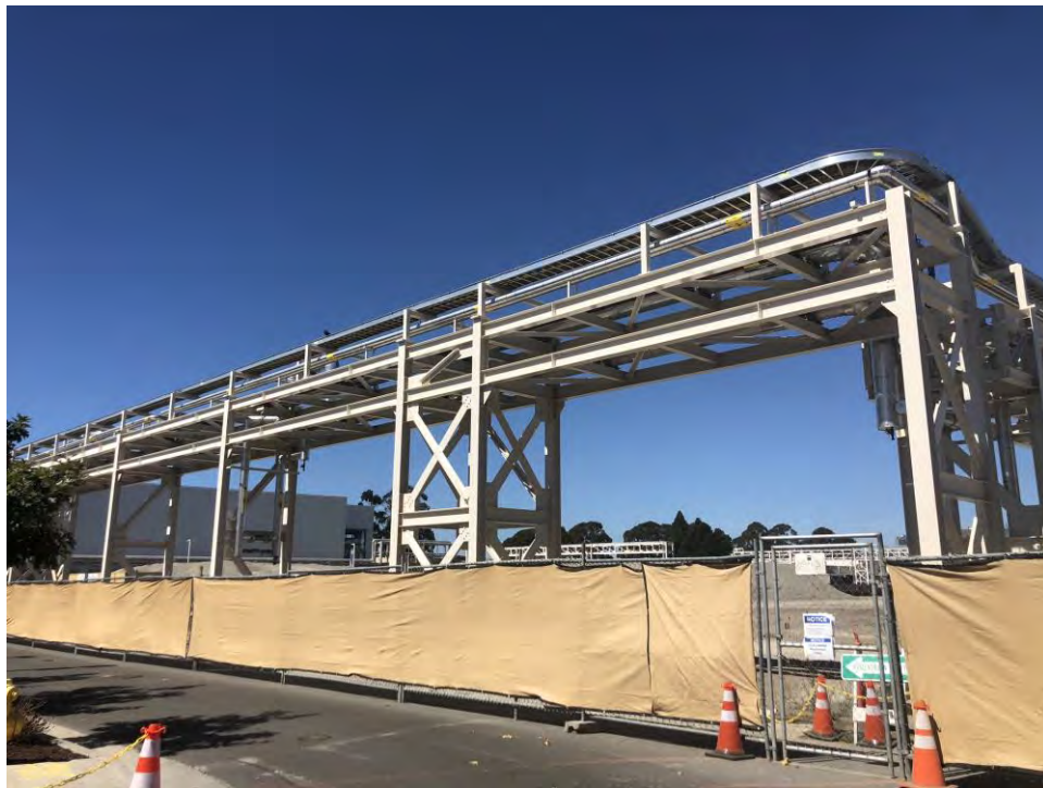
Photograph 18: Demolition site on Parcel 2 (formerly buildings B49, B13, and B52).
