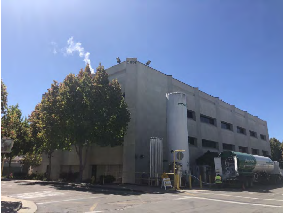
Photograph 1: Building B57 on Parcel 1 and liquid nitrogen tank filling station.
