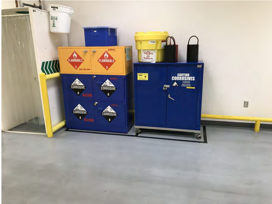
Photograph 29: Flammables and corrosive materials cabinets in building B80.
