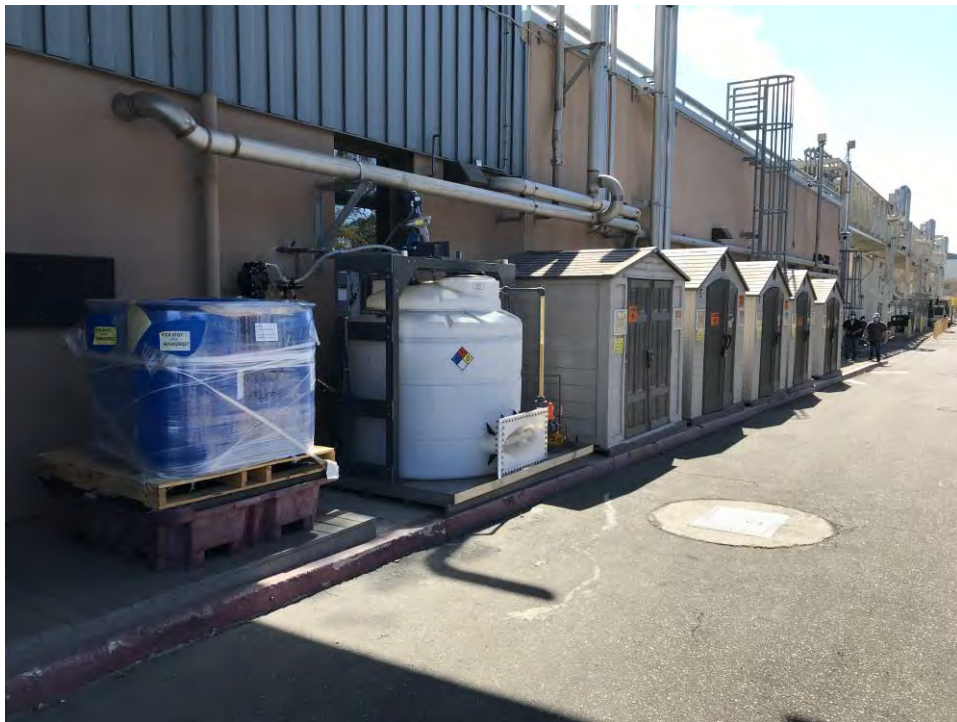
Photograph 2: Biohazard storage unit along exterior of building B60 on Parcel 1.
