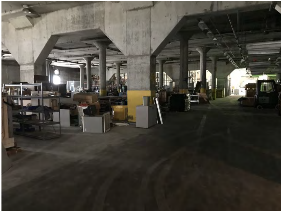
Photograph 22: Interior of building B83.
