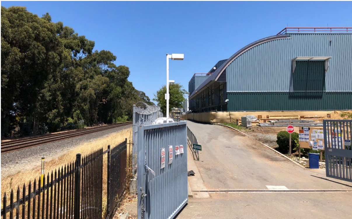
Photograph 6. Northward view of building B80 on the South Properties, adjacent to railroad tracks.
