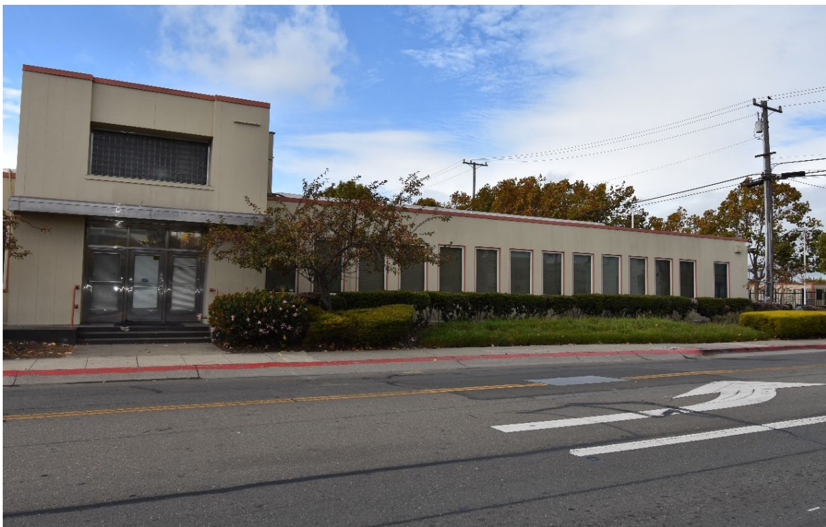
Photograph 4. Westward view from Seventh Street of engineering offices building B56.
