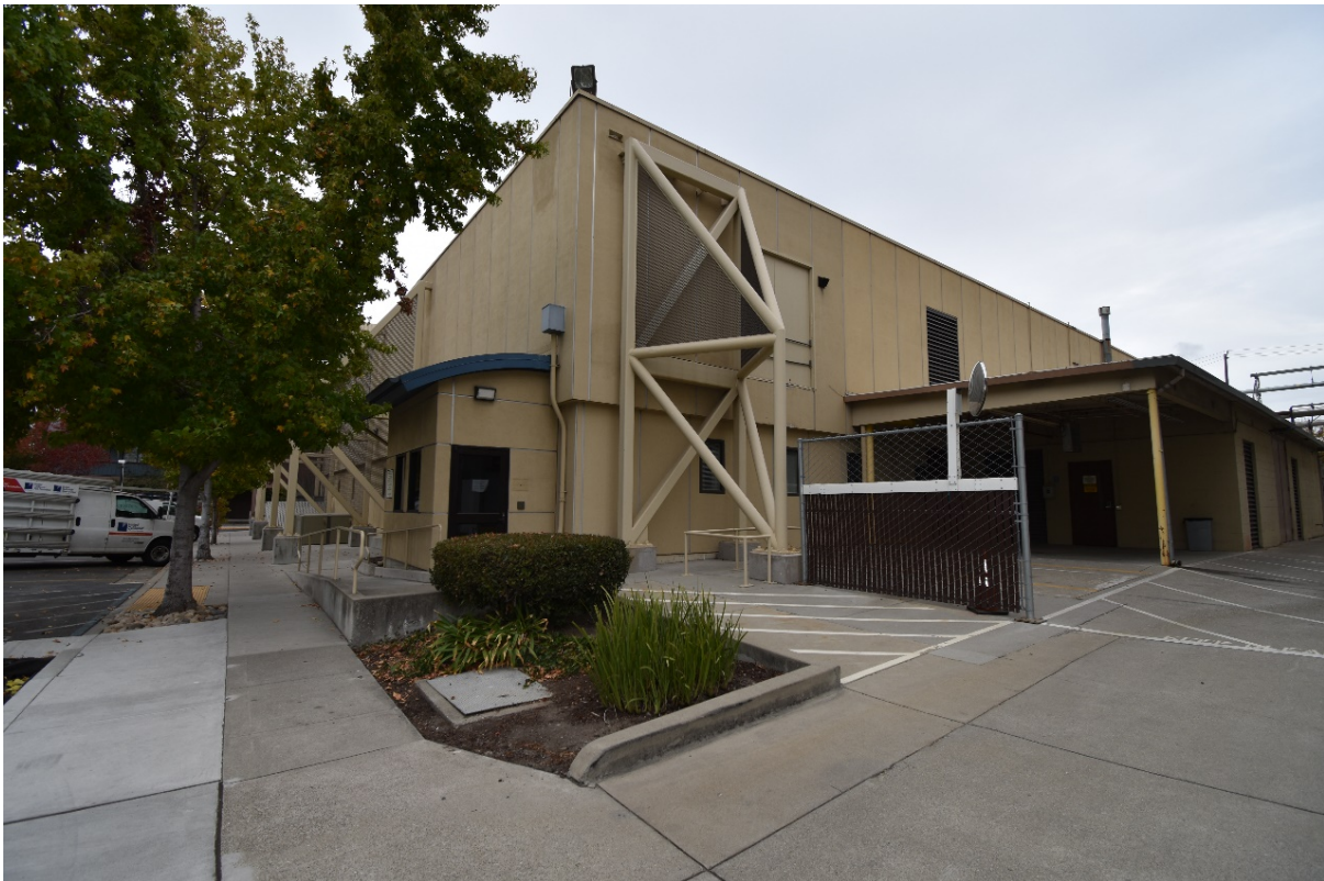
Photograph 2. View looking northwest to laboratory building B53, south of Dwight Way.
