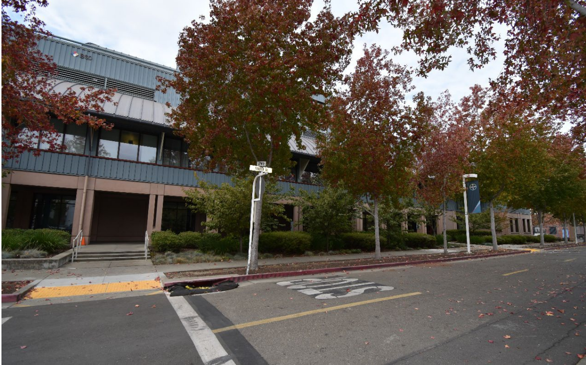
Photograph 1. Westward view from Fourth Street to the rFVIII API building (B60).
