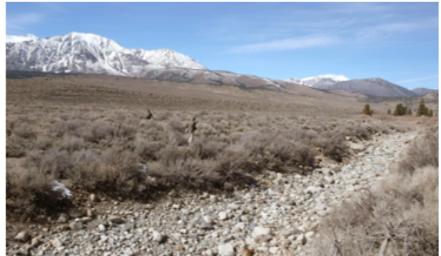
Unlined spillway, looking northwest
