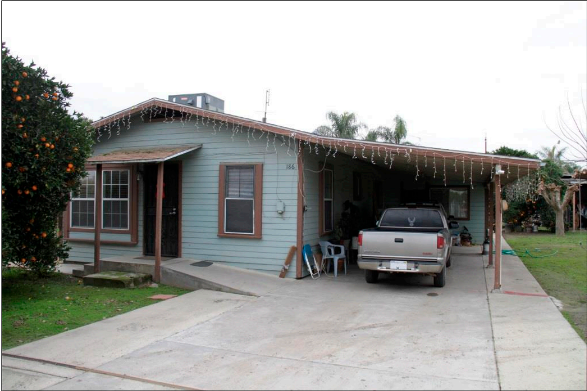
Figure 4 Example of single-family residence at 186 E. Nebraska Avenue; view to the south.
