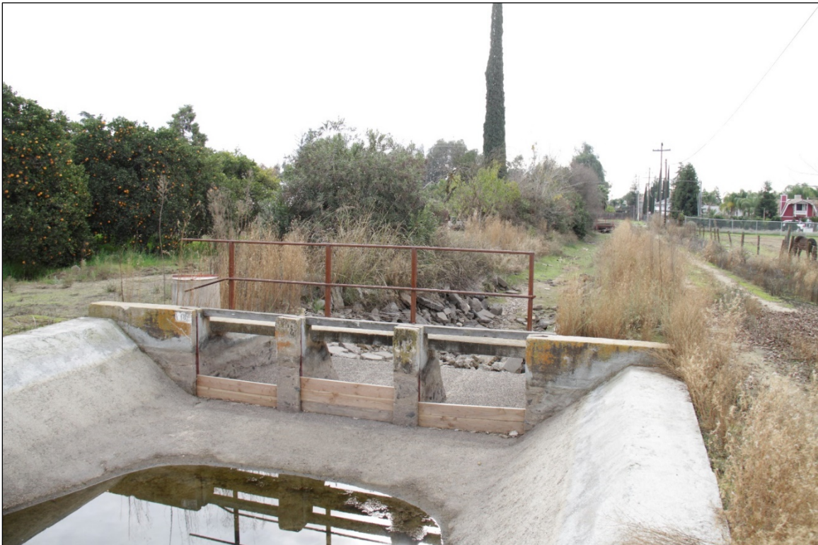
Figure 5 Dinuba Town Ditch; view to the south.
