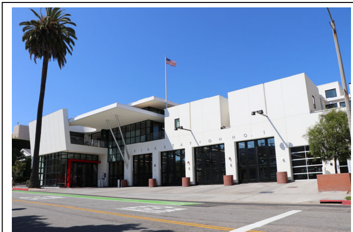
Station No. 1 was relocated from 1444 7 th Street to 1337 7 th Street. The new SMFD Fire Station No. 1 was open for operation in July 2020. The new station provides expanded space to support existing operations. (The relocation did not expand staffing or the number of assts at Station No. 1.)
