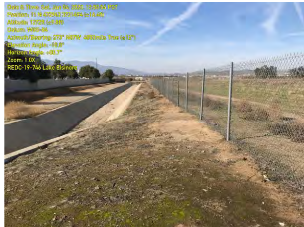
Photo 1a. East end of concrete channel that runs along the southern boundary of the site, facing west. The project site is to the right of the chain link fence (01.04.2020).
