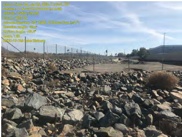
Photo 1. West end of concrete channel that runs along the southern boundary of the site, facing east (01.04.2020).
