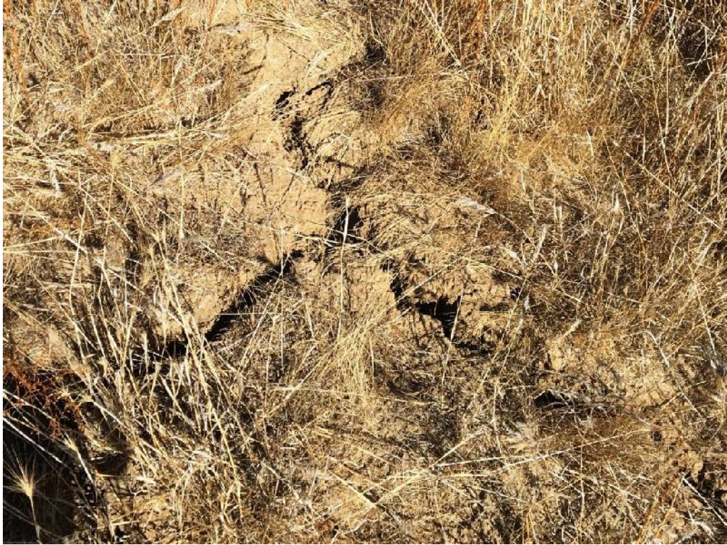
Photo 7. Soil cracks in Bosanko clay in southwestern BSA.
