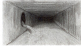
Underground storm drain tunnel
