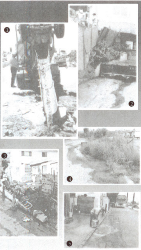
Photos (top to bottom): 1) Illicit discharge from washing down cement truck chute. 2) Erosion and runoff from a construction site. 3) Inadequate containment at a construction site resulting in runoff into the street. 4) Unusual vegetative growth indicates a constant discharge. 5) Restaurant worker dumping floor wash water from bucket into the gutter.
