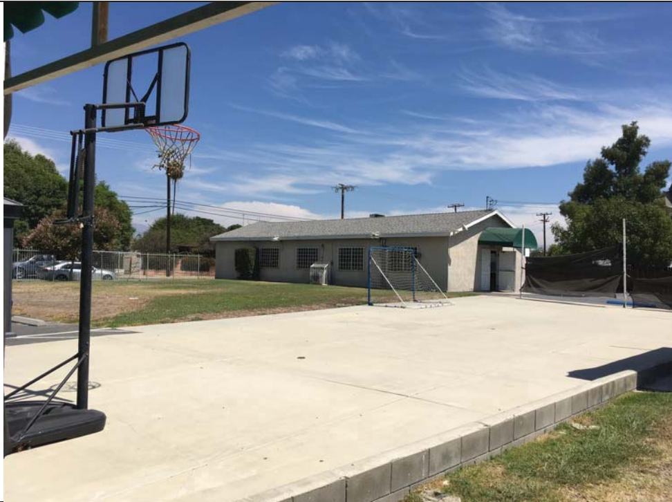
Photo #3 View of the youth chapel in the northeastern portion of the Property.
