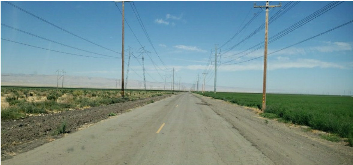
Photograph 4: Pipeline route in northwestern portion of project site.
