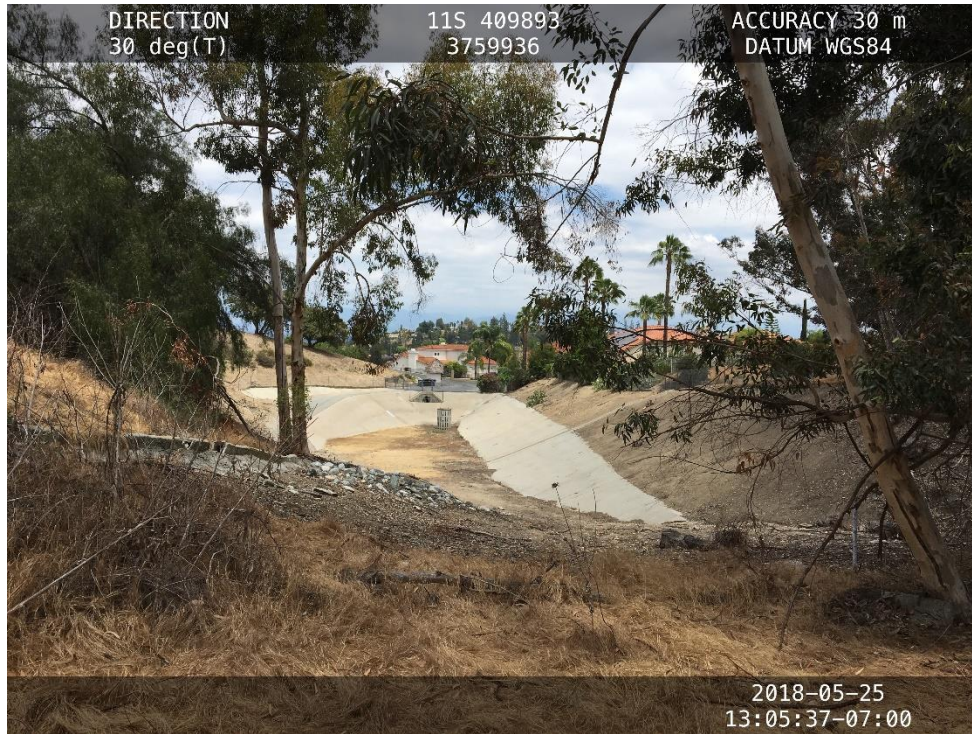
Photo 7. Depicts a retention basin north of Drainages 3 and 4 and shows the lack of hydrological connection from the drainages to the basin.
