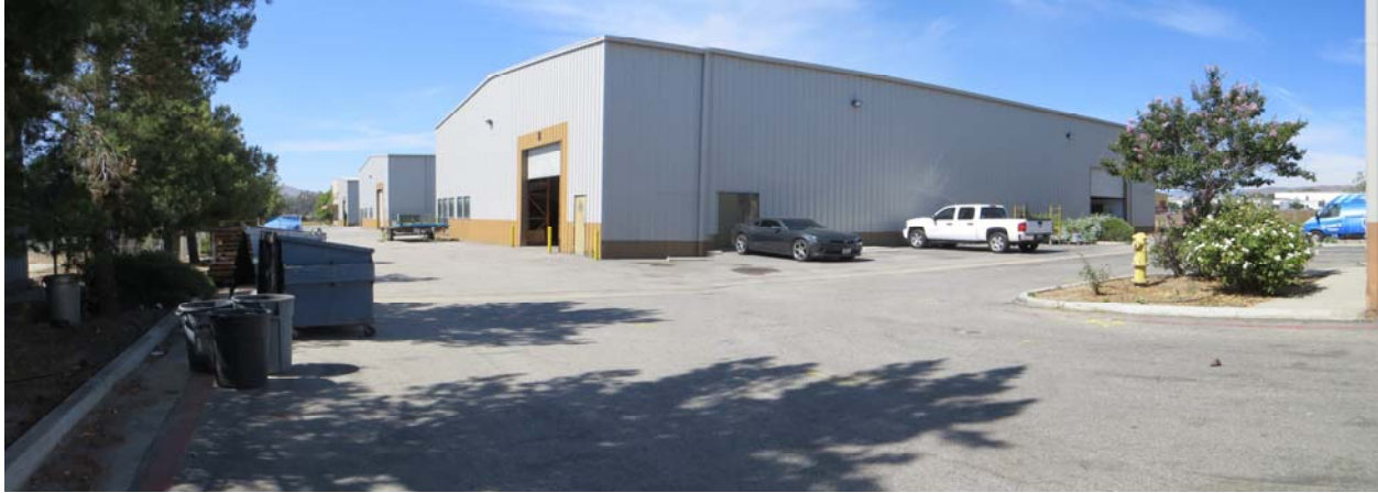
Photograph 15: Southwest view of the middle of the east adjoining site. 224 Malbert, Unit C, in foreground with Units B and A in the background.
