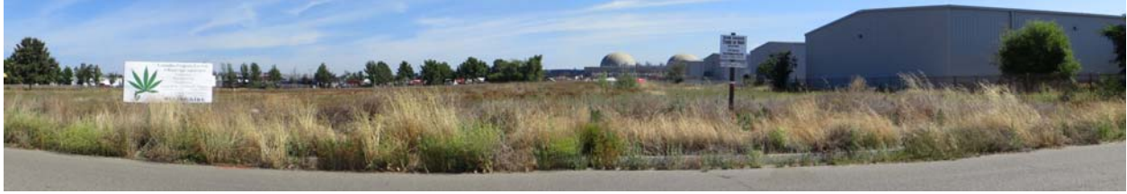
Photograph 1: North view of the Property from Malbert Street. Buildings on the right are located at 224 Malbert Street (east adjoining site.)
