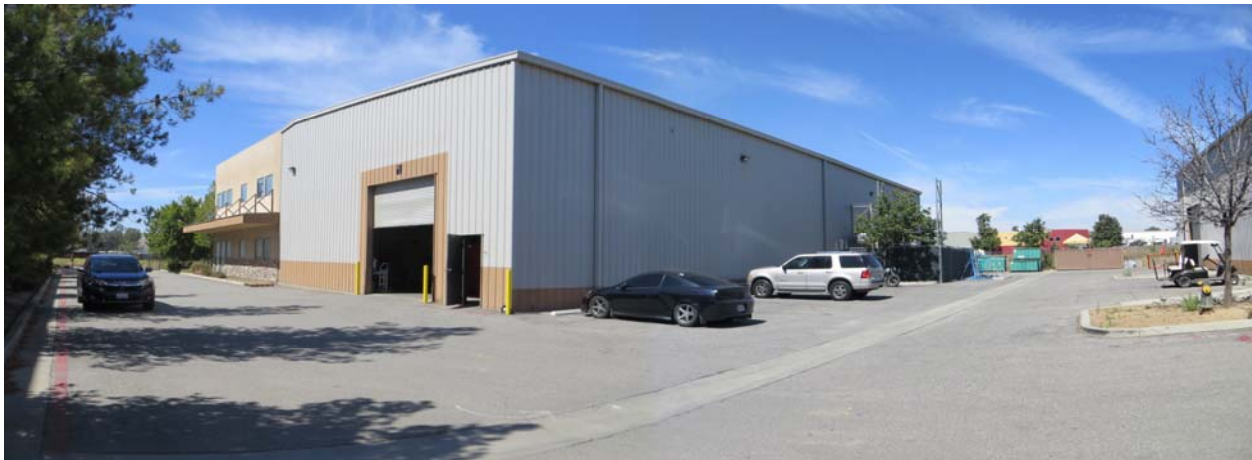
Photograph 16: Southwest view of the south end of the east adjoining site. This warehouse is 224 Malbert, Unit A, occupied by Skylon.
