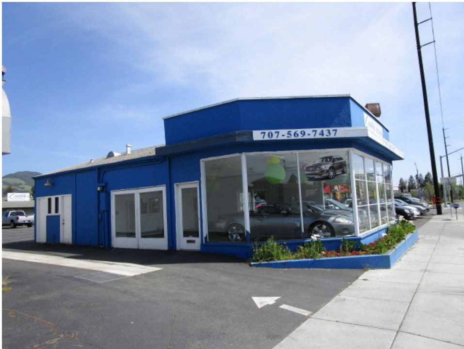
56. Quality Motors (2620 Santa Rosa Avenue) adjacent to the west
