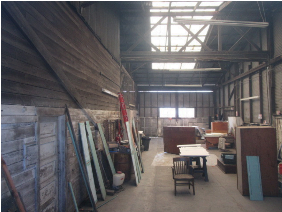
34. Interior of the former Hulsman Transportation building
