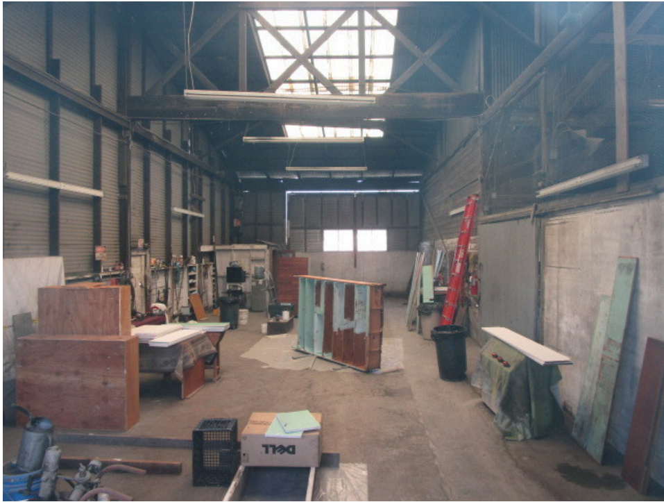
31. Interior of the former Hulsman Transportation building
