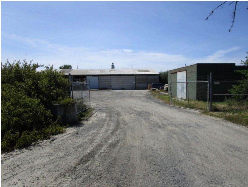
6. Gate on the central portion of the 325 Yolanda property
