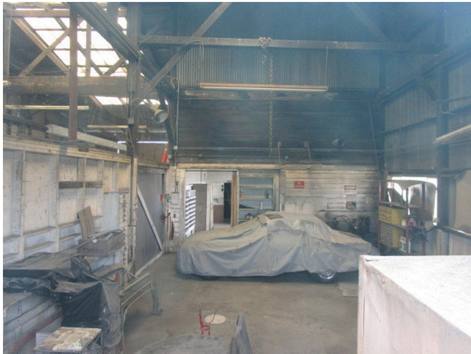
30. Interior of the former Hulsman Transportation building
