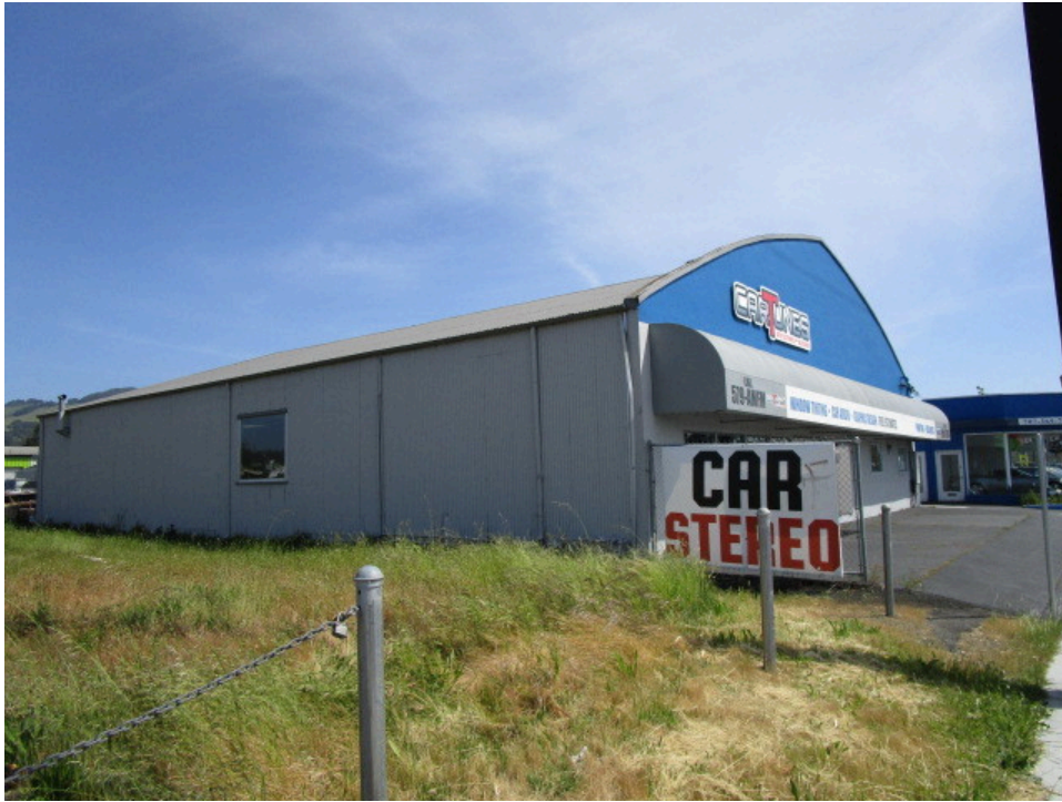
57. Car Tunes (2612 Santa Rosa Avenue) adjacent to the west and south
