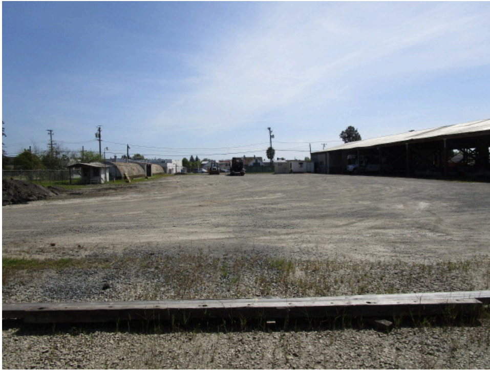
7. View south of the 325 Yolanda property
