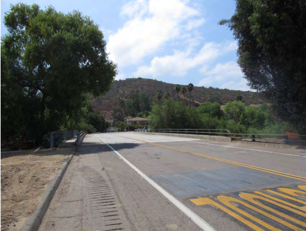
Photo 7. Looking southeast at Old River Road where it crosses Moosa Creek.
