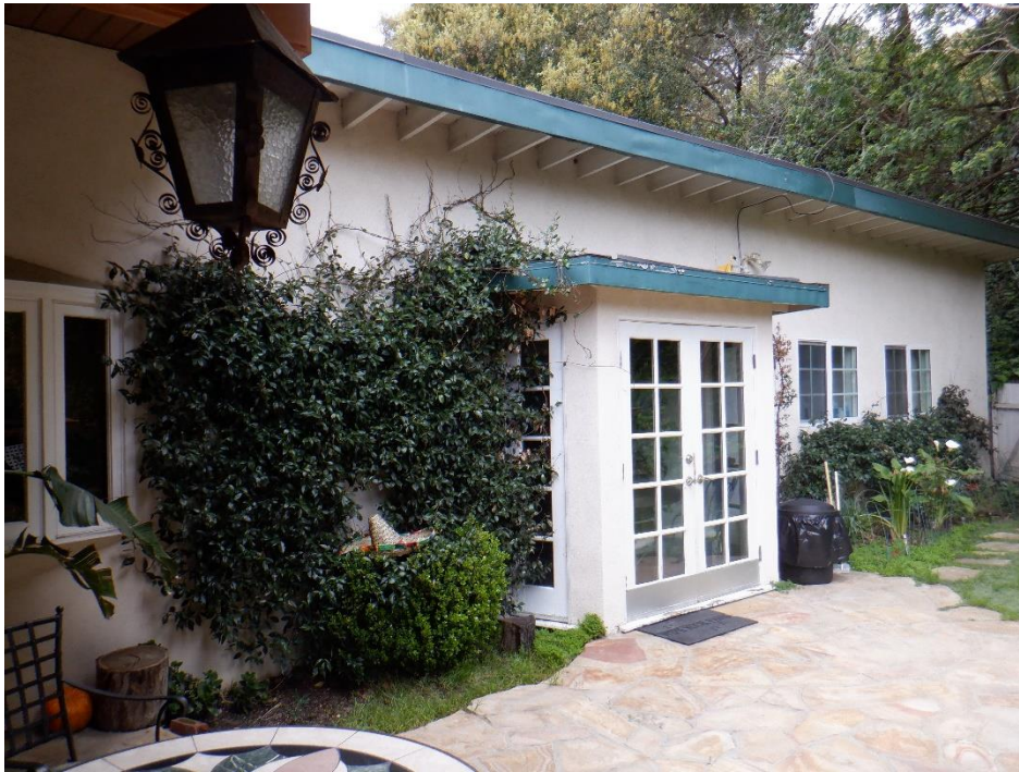
Detail of exposed roof rafters in the wide eave overhangs, clerestory windows, and hanging Spanish style lantern.
