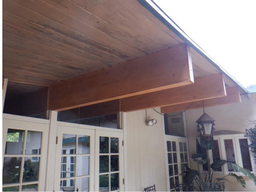
Exhibit 19. Detail of exposed roof beams in the wide eave overhangs, clerestory windows, and hanging Spanish style lantern.
