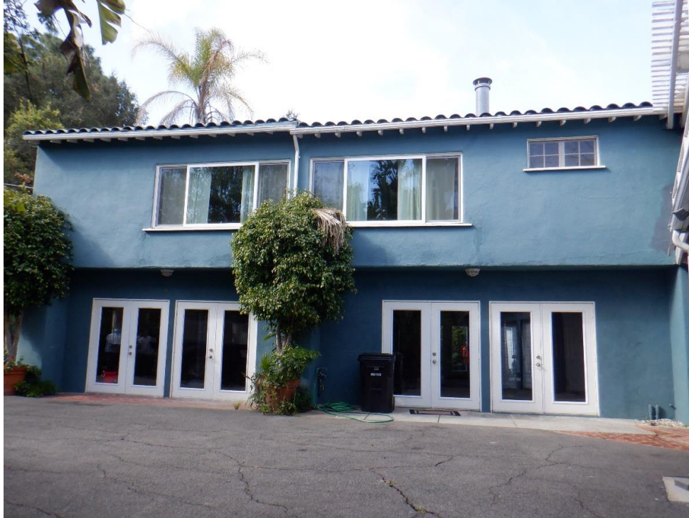
Exhibit 25. East façade with four sets of vinyl glazed French doors on the ground level and two sliding windows and a casement window on the upper floor. Notice the different roofline levels and the roof-tail rafters between the original northern half versus the southern addition added circa 1978.
