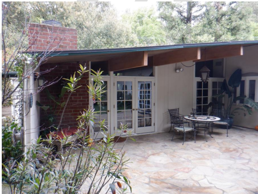
Exhibit 18. French doors, exposed roof beams in wide eave overhangs with a hanging Spanish style lantern on the east façade within the enclosed private courtyard. Notice the low, broad brick chimney.
