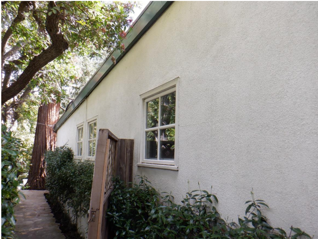
West façade with entry gate and three fixed windows, looking north.
