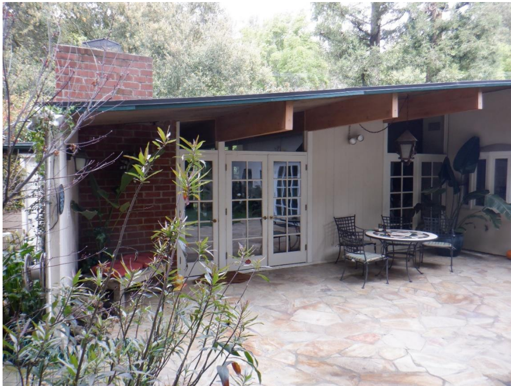
French doors, exposed roof rafters in wide eave overhangs with a hanging Spanish style lantern on the east façade within the enclosed private courtyard. Notice the low broad brick chimney.
