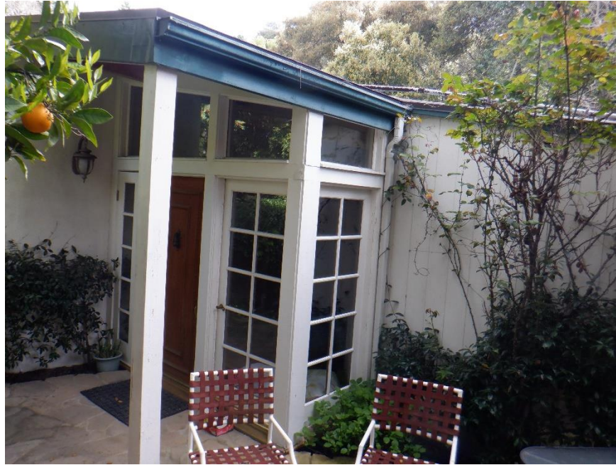
Front entry courtyard with recessed door on west façade, looking north.
