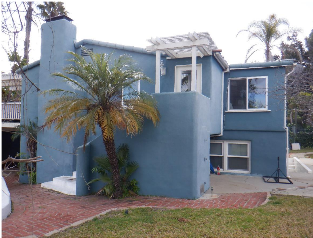
North façade with broad chimney and second story entry.
