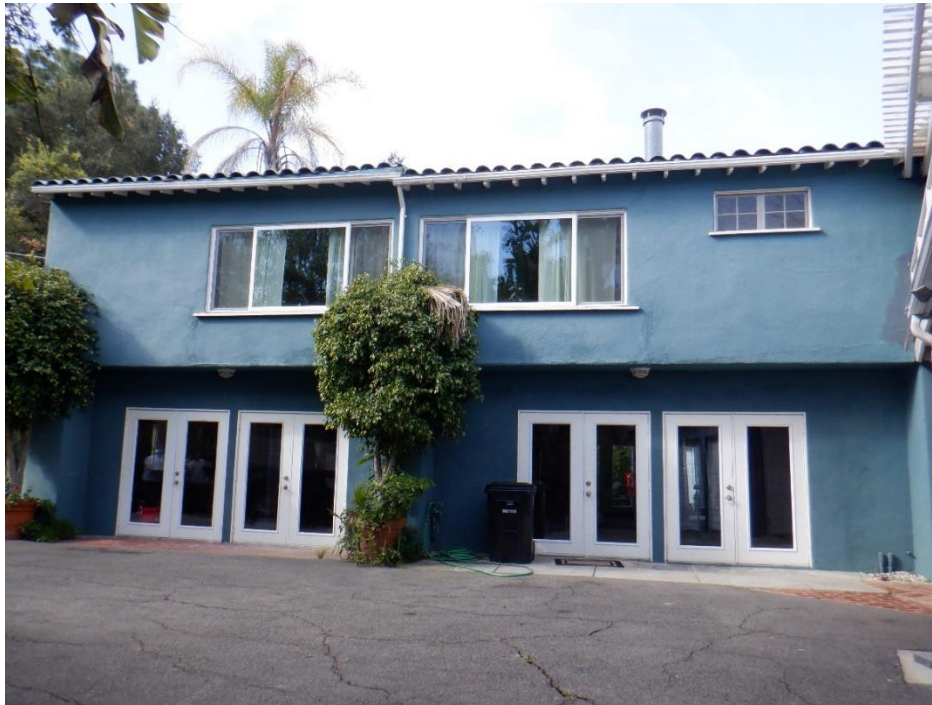
East façade with four sets of vinyl glazed French doors on the ground level and two sliding windows and a casement window on the upper floor. Notice the different roofline levels and the roof-tail rafters between the original northern half versus the southern addition added circa 1978.
