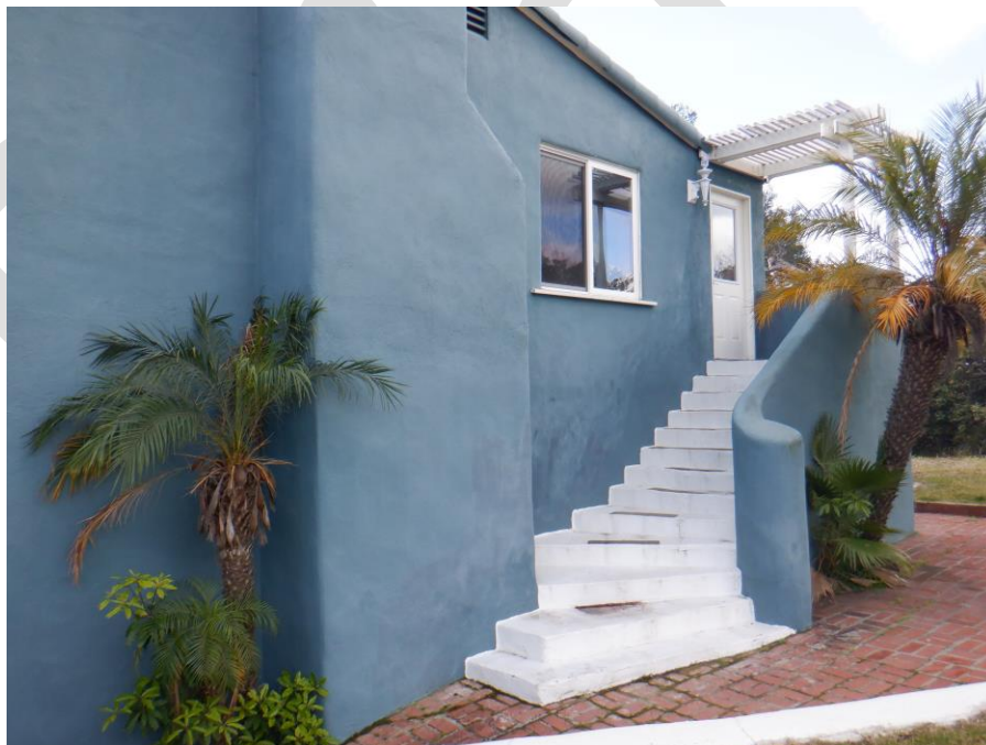
Exhibit 28. North façade entry with curving concrete stairs and curved stucco railing. The entry features an attached lattice patio cover.
