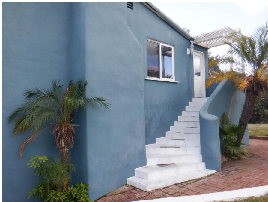
North façade entry with curving concrete stairs and curved stucco railing. The entry features an attached lattice patio cover.
