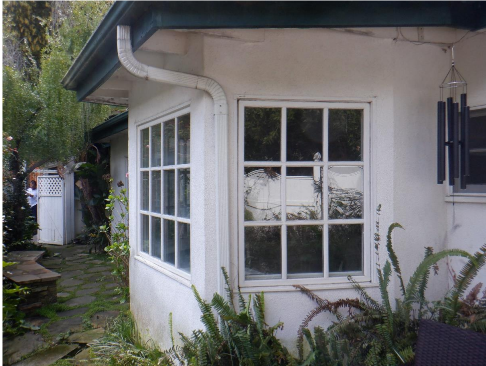
Exhibit 17. Pop-out addition added to the north façade in 1998, looking east.
