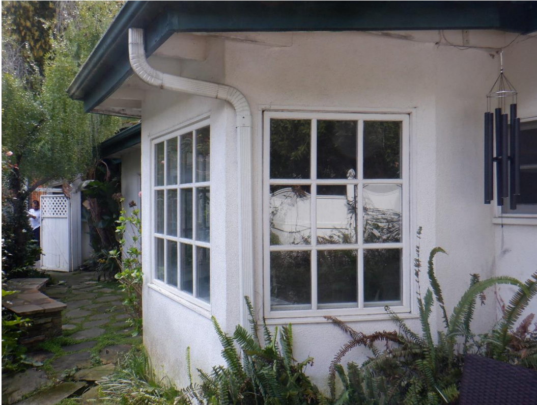
Pop-out addition added to the north façade, looking east.
