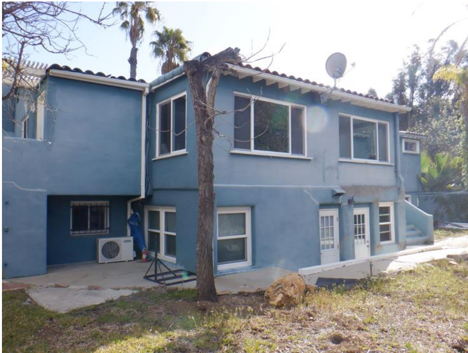
Addition on the west façade added sometime before 1962.
