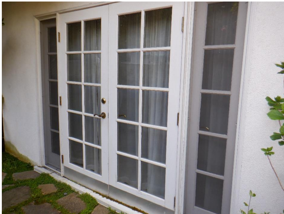
French door detail on north façade, looking southwest.
