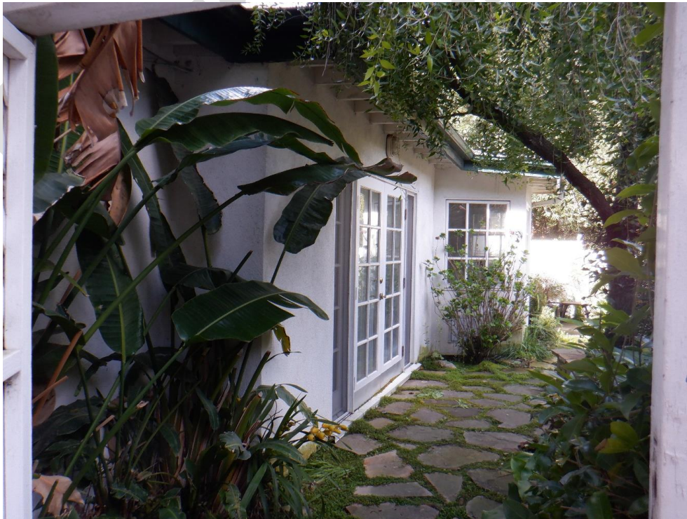
Exhibit 16. Enclosed side-yard walkway along the north façade with a 122-square foot addition from 1998.
