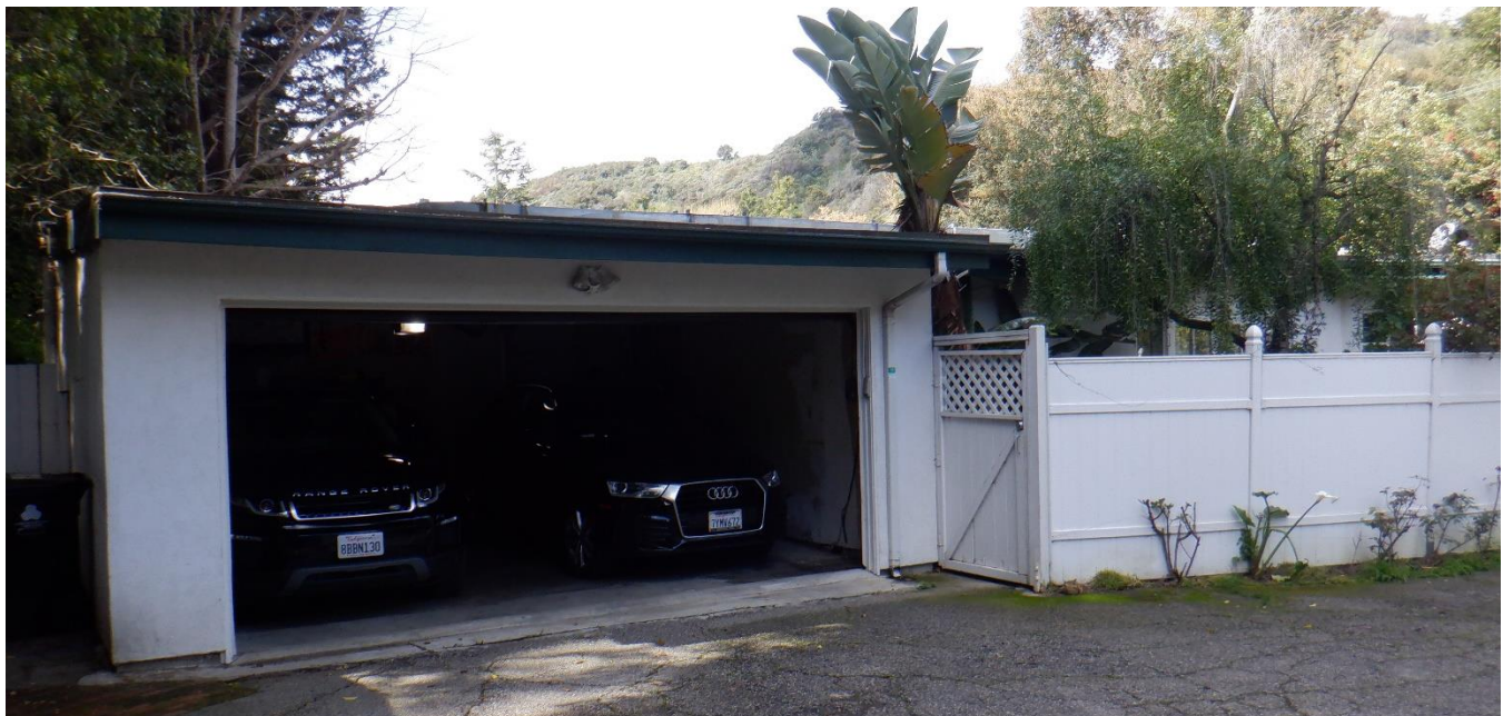
Attached two-car garage on the north façade, looking southwest from the driveway.
