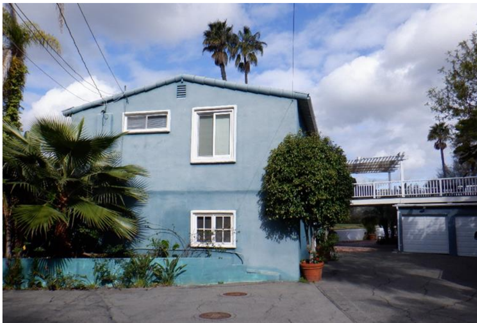
South façade with detached garage in the background, looking northwest from the driveway.
