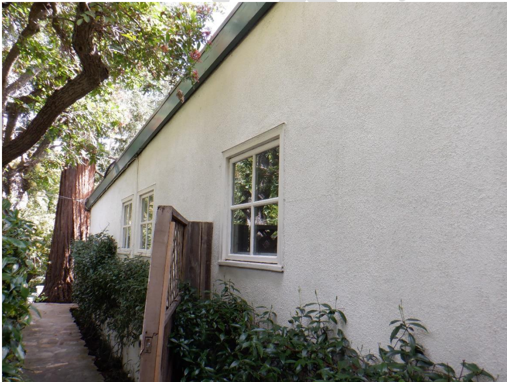
Exhibit 14. West façade with entry gate and three fixed windows, looking north.
