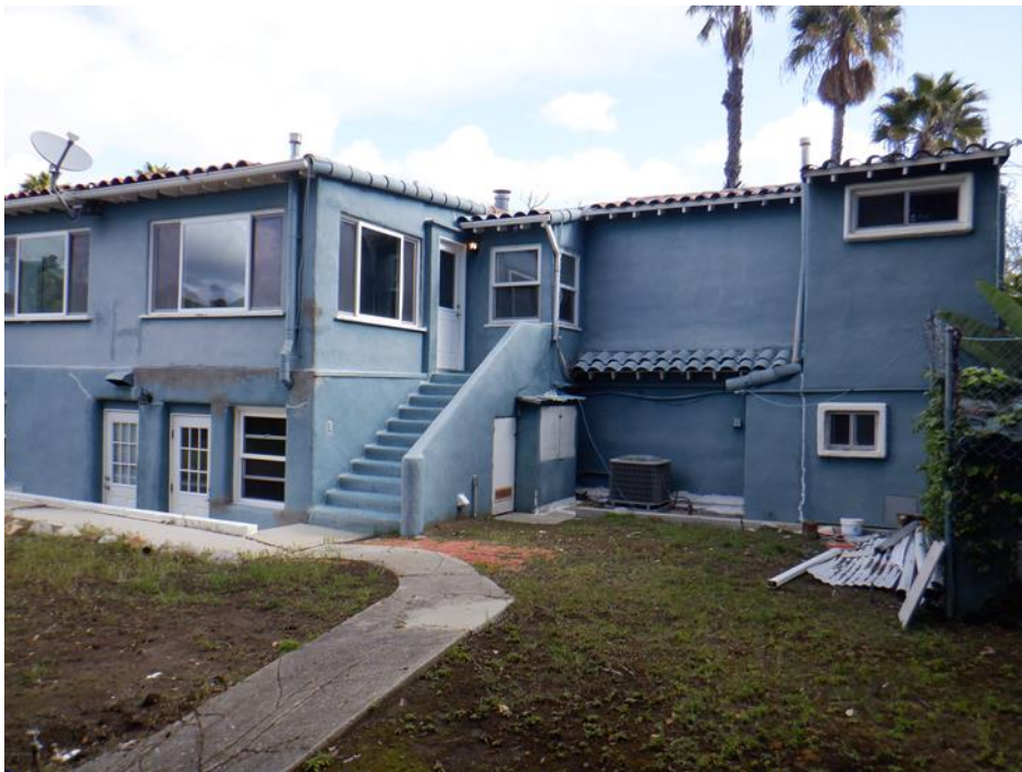
West façade with variations of windows and three entries. This photograph shows the two major additions to the house. The original southwest corner of the house is at the top of the staircase with an addition to the west and another on the south.
