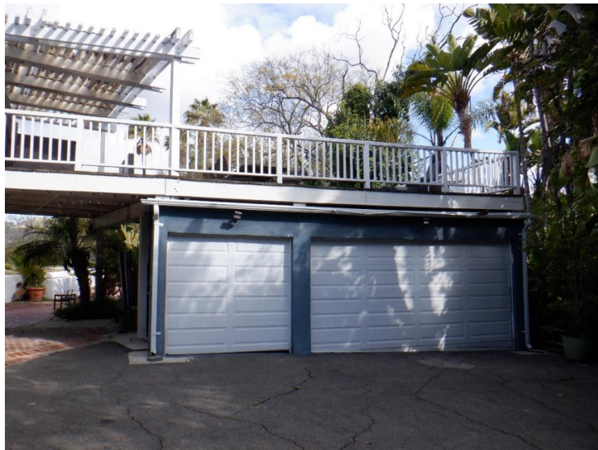
Second story balcony with three-car garage added in 1991.
