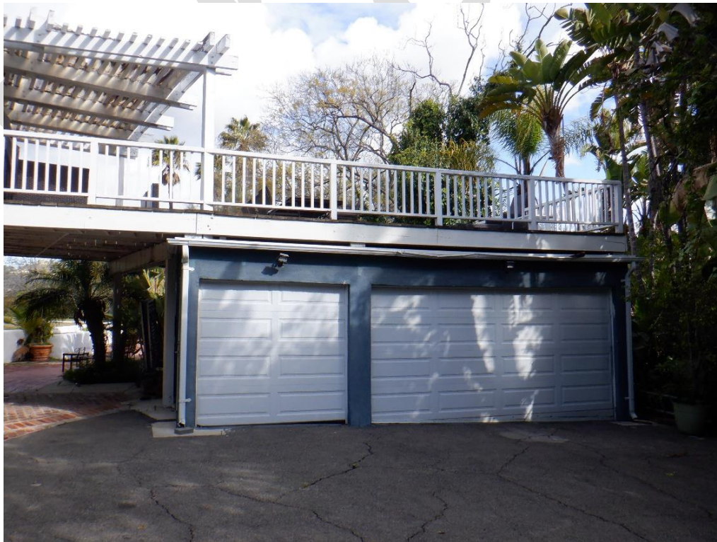
Exhibit 26. Second story balcony with three-car garage.
