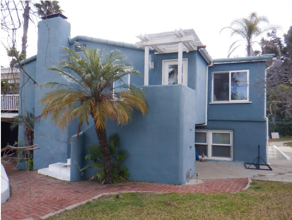
Exhibit 27. North façade with broad chimney and second story entry.
