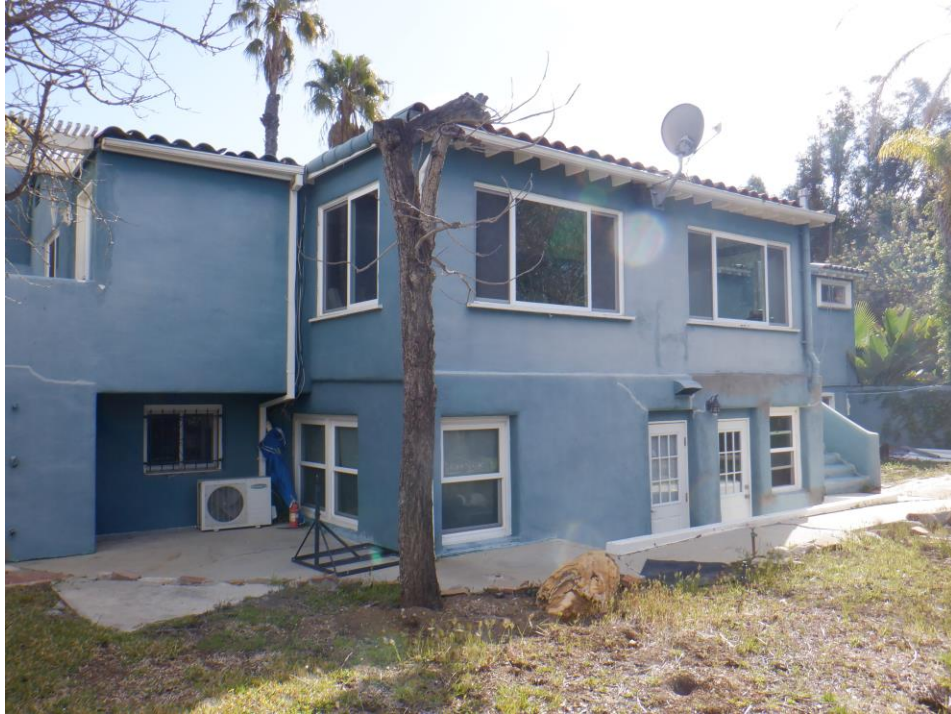
Exhibit 29. Addition on the west façade added sometime before 1962.
