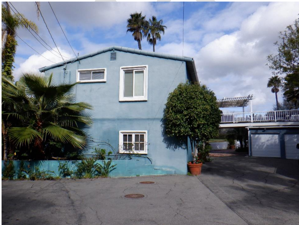
Exhibit 24. South façade with detached garage in the background, looking northwest from the driveway.
