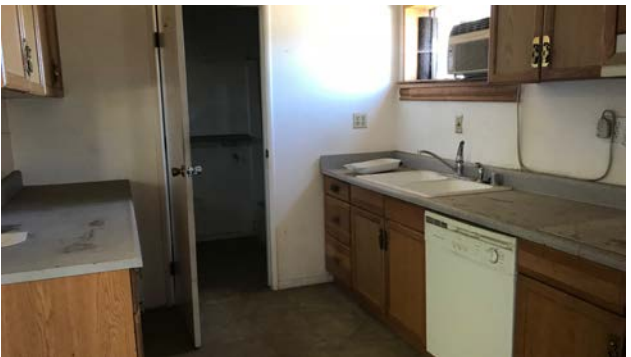
Photograph 10. View inside the residence on the second floor of the structure on the southwestern portion of the subject property.
