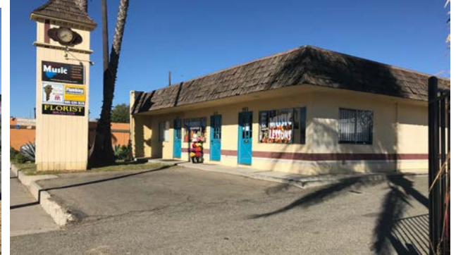
Photograph 9. View of western adjacent commercial businesses, facing northwest.
