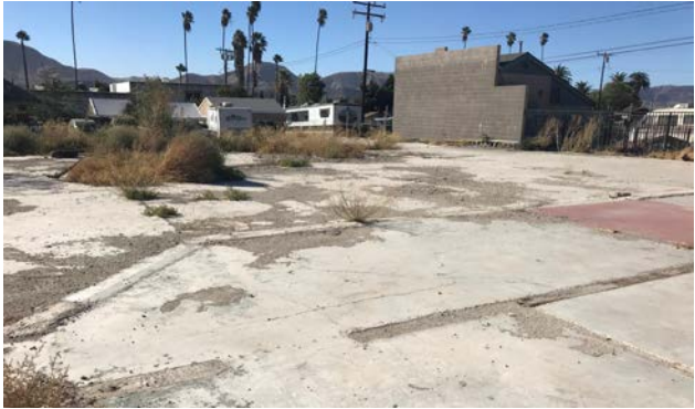
Photograph 1. View of the undeveloped concrete area located on the northern portion of the subject property, facing west.
