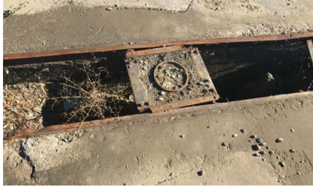
Photograph 2. View of the in-ground hoists present at the undeveloped concrete area on the northern portion of the subject property.
