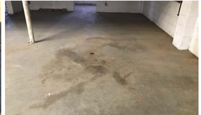
Photograph 9. View of staining inside the former automotive repair building on the southern portion of the subject property.
