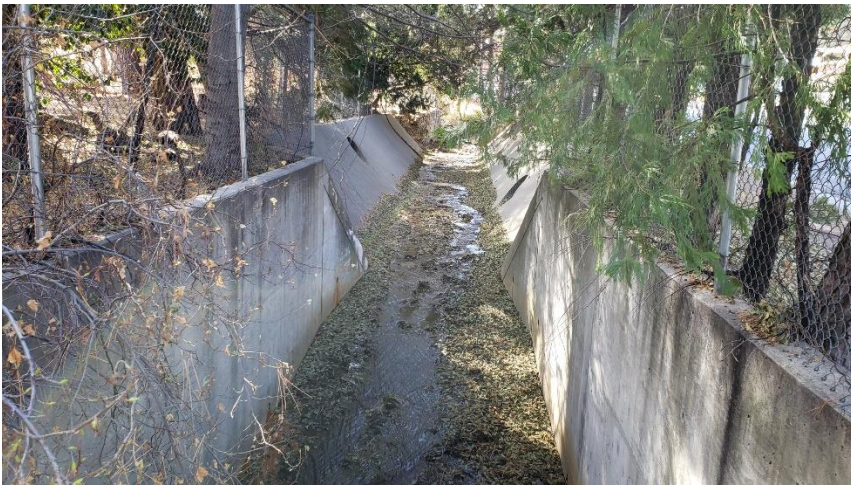
Photo 10. Photo depicts a concrete lined channel with 8-foot wide box culvert and water flowing (east) approximately 100-foot north of site.
