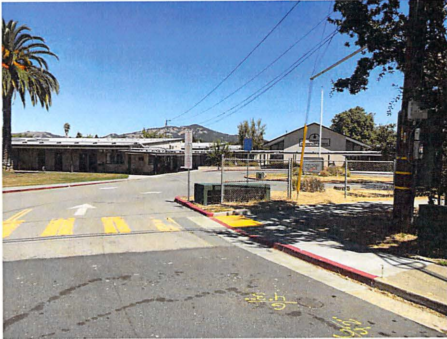
Figure 5: View of Access to Lynwood School from End of Lynwood Drive
