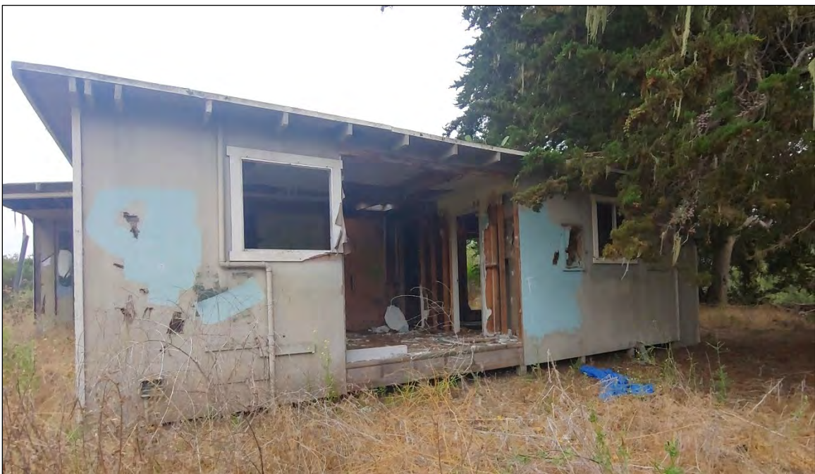
Figure 5-2 North elevation of the residence, view facing south.
