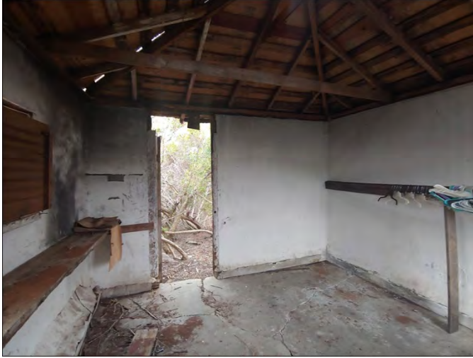
Photo 14: Shed interior. View facing west.
