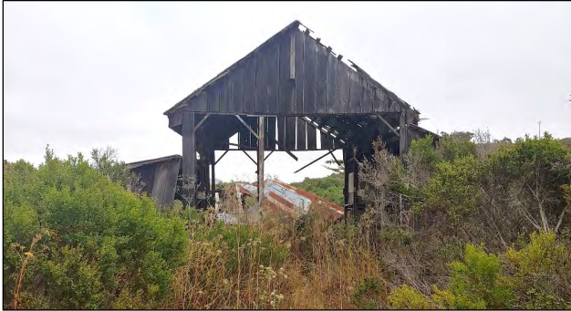
Photo 8: West elevation of the barn, view facing east. View obscured by vegetation.
