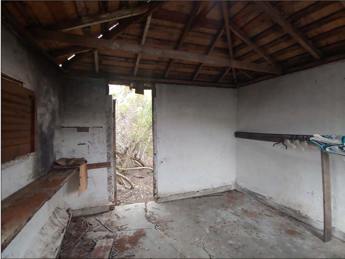
Figure 5-11 Shed interior. View facing west.
