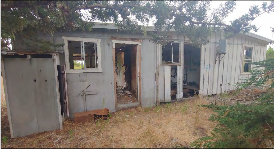
Figure 5-3 West elevation of the residence with addition on the left, view facing east.
