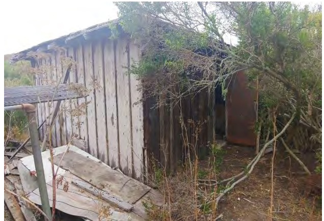
Photo 12: Shed exterior. View facing southeast.
