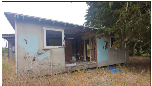
Photo 5: North elevation of the residence, view facing south.
