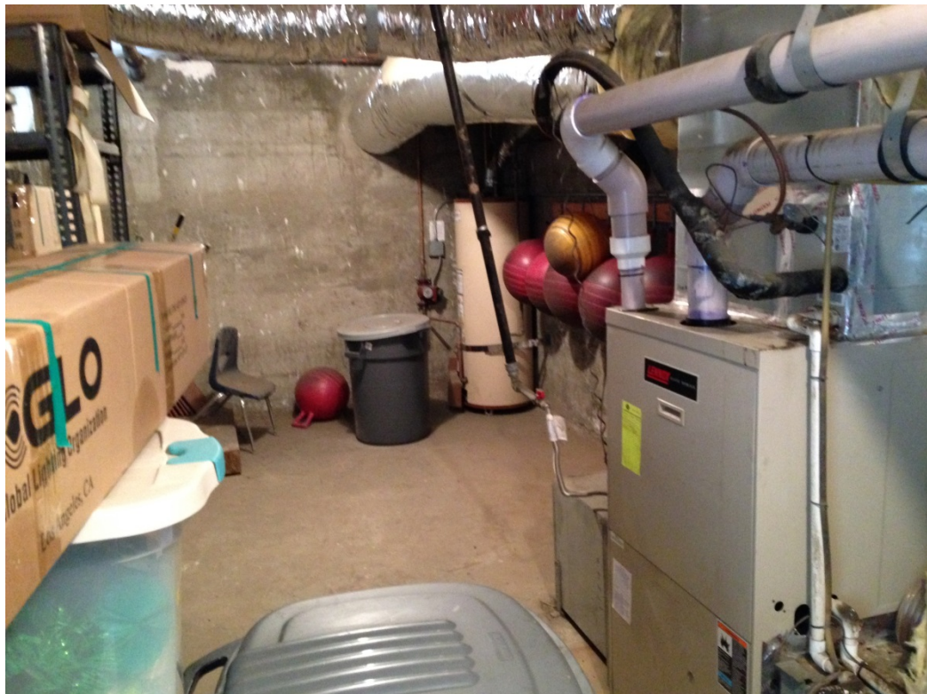
Photo No. 10: View of the mechanical room for the church offices/classrooms.
