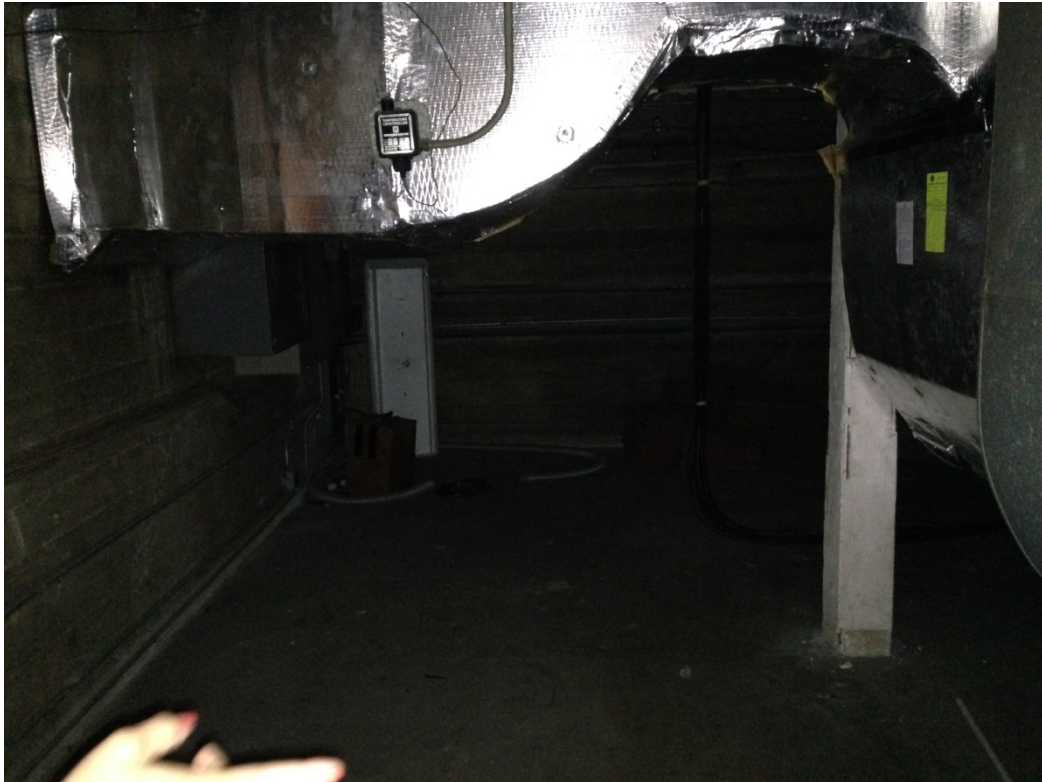
Photo No. 11: View of the mechanical room for the church sanctuary.
