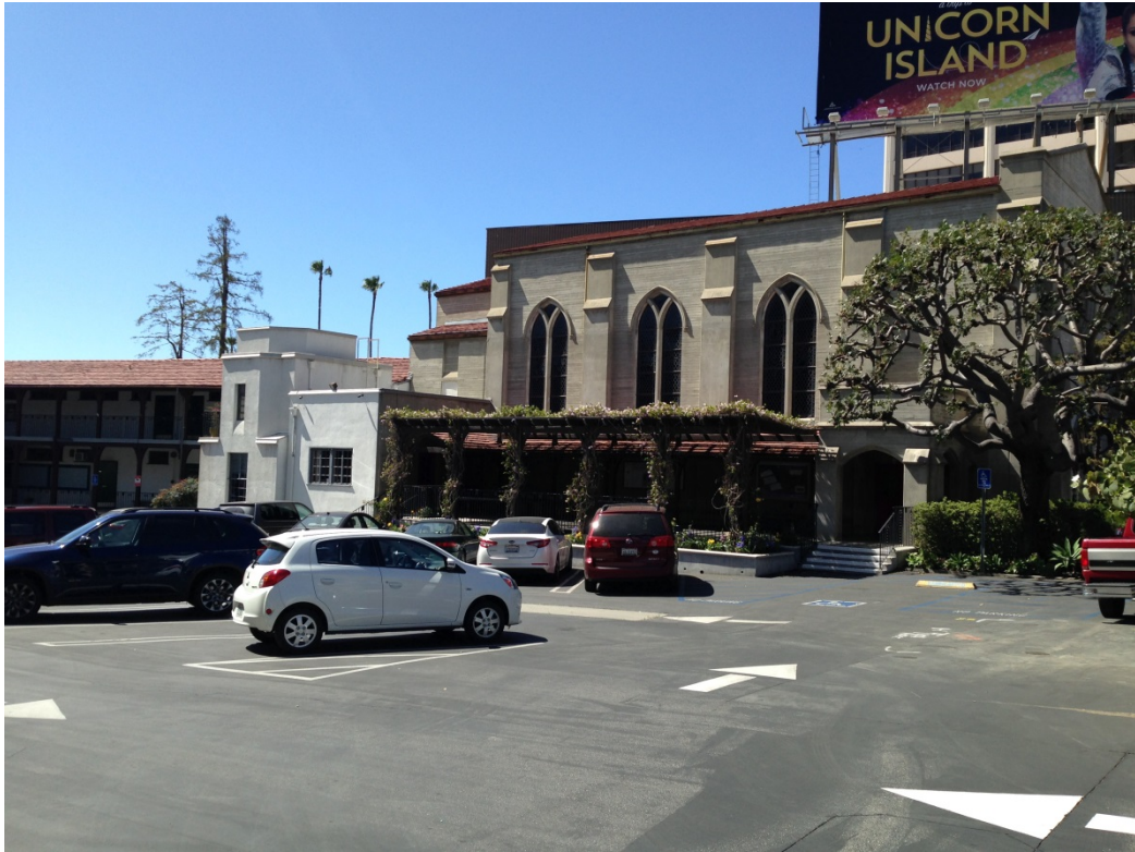
Photo No. 3: View to the west of the subject property, including the northern surface parking lot, sanctuary, and church offices.
