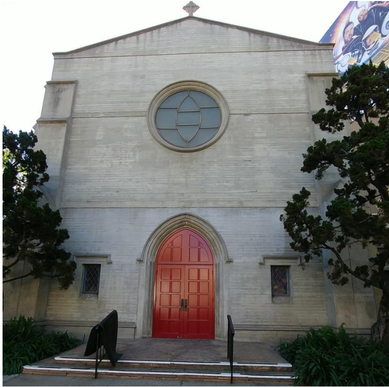
Figure 6 North elevation of church, view looking south
