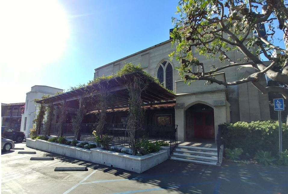
Figure 8 East elevation of church, view to the southwest
