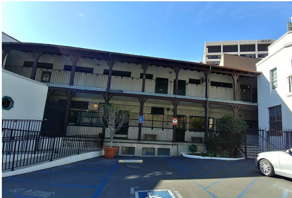
Figure 10 Preschool, east elevation, view to the west
