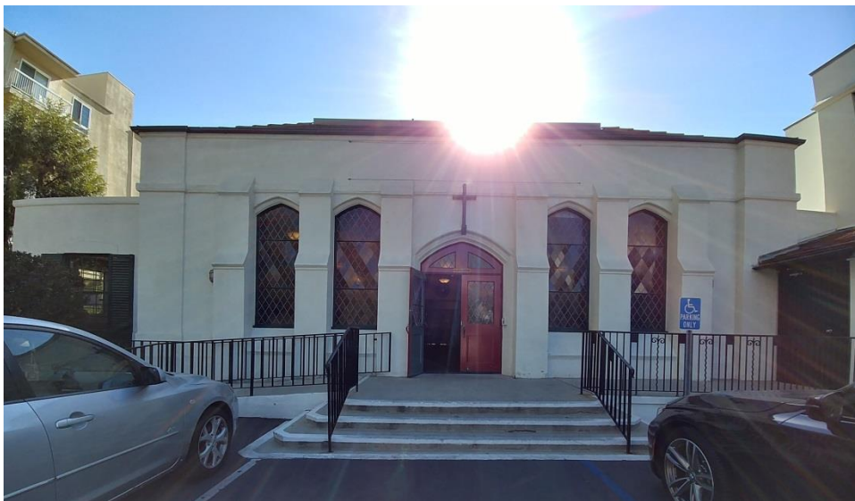
Figure 12 Closeup of Fellowship Hall's north elevation, view to the south
