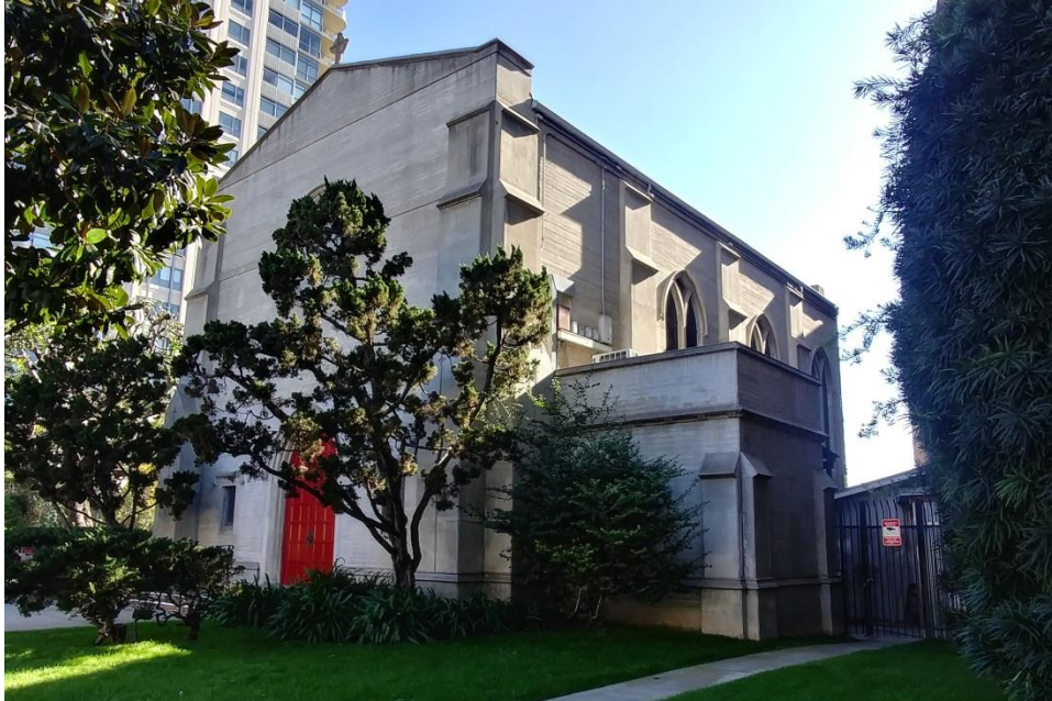
Figure 7 North and west elevations of church, view looking southeast
