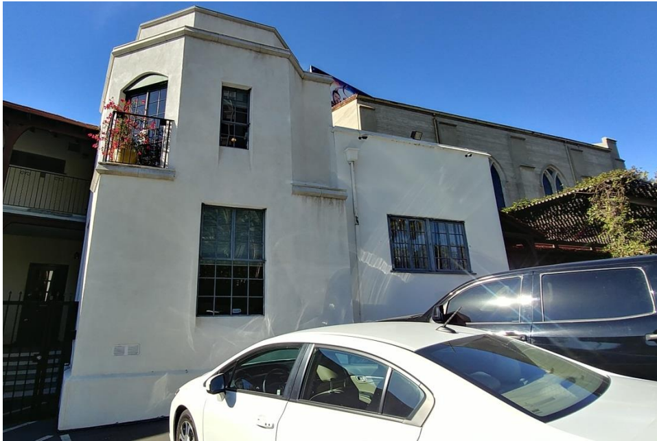
Figure 9 Administration office, east elevation, view to the northwest
