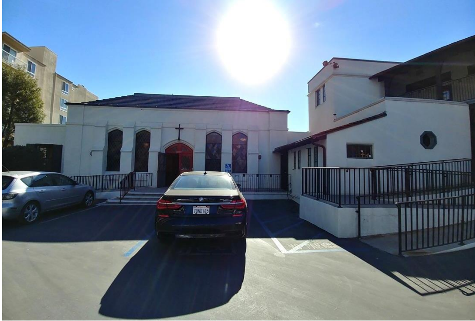
Figure 11 Fellowship hall and office space, view to the south
