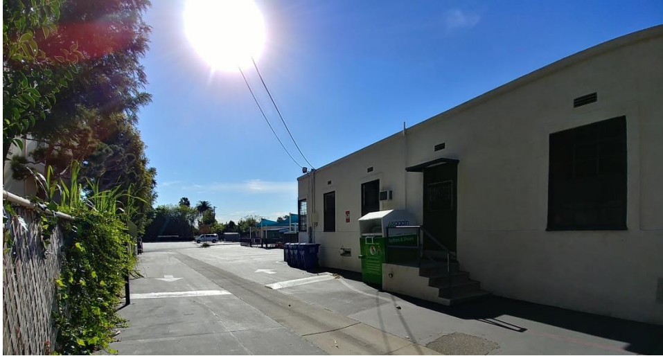
Figure 13 East elevation of Fellowship Hall and rear parking lot, view to southwest
