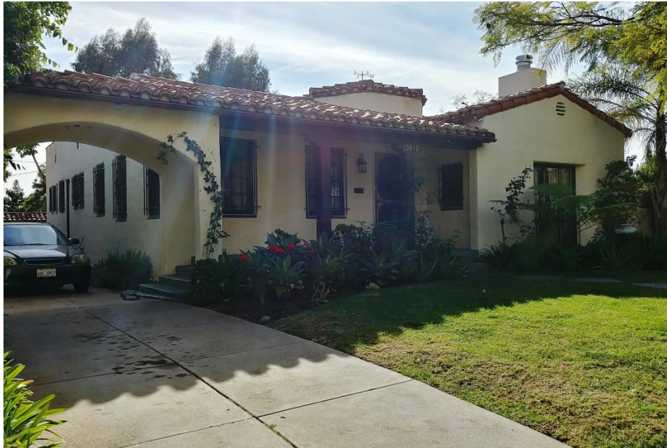
Figure 16 North façade and east elevation of 10812 Ashton Avenue, view to southwest
