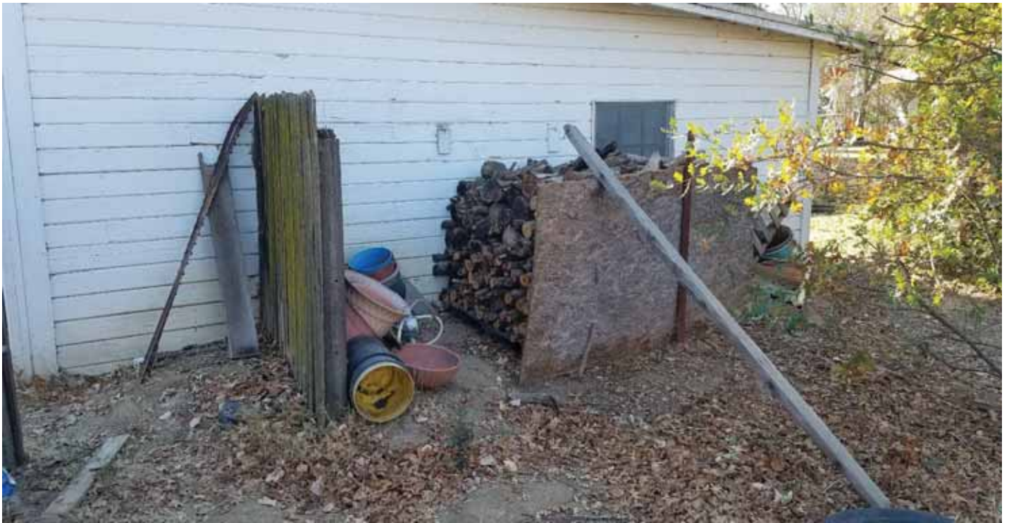
Photo 9: Looking southwest at the north wall of the garage.
