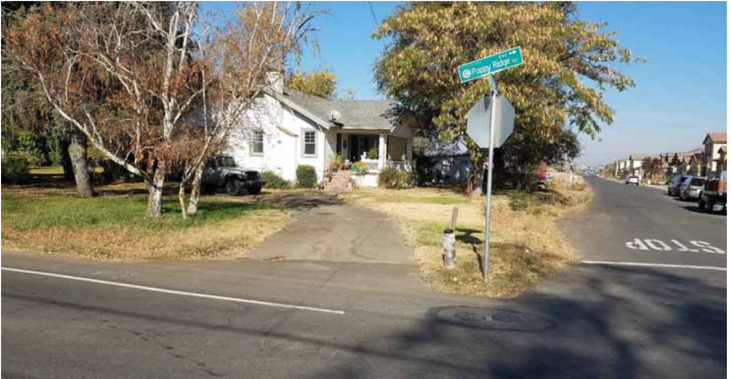
Photo 1: Looking north at the southeast corner of the Site from the intersection of Poppy Ridge and Lousada.
