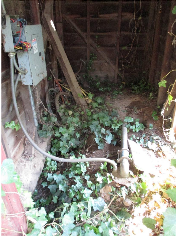
Figure 24. Photo showing the interior of the ca. 1920 well house building.
