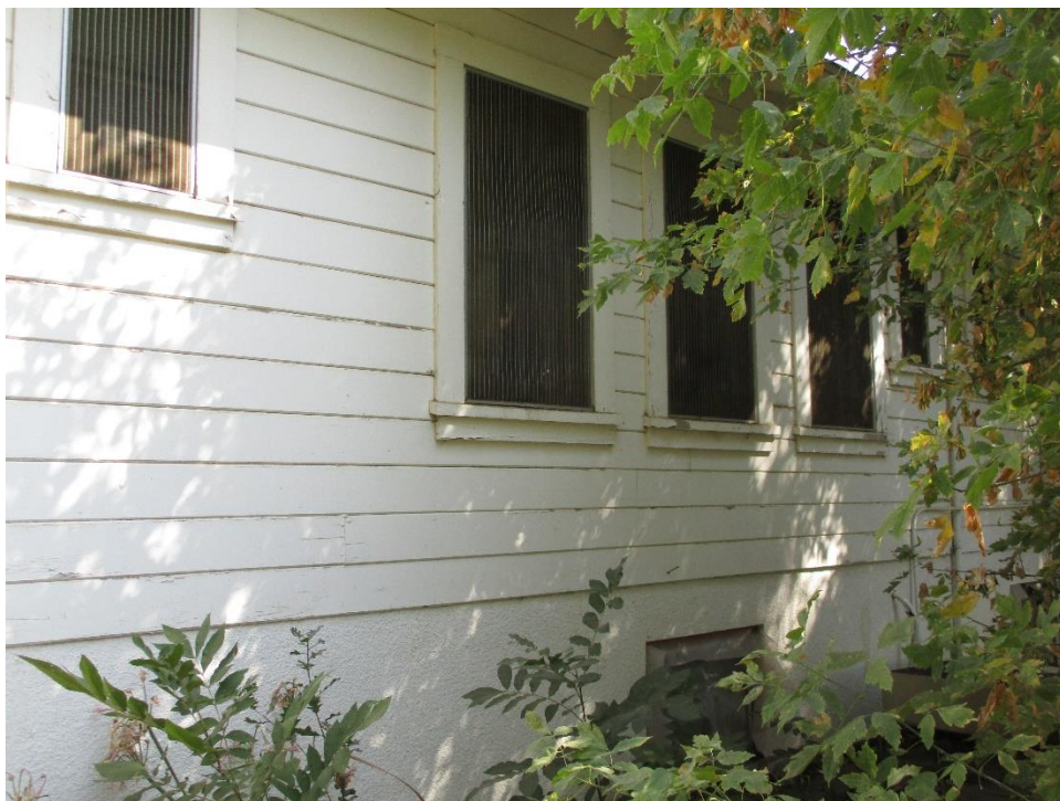
Figure 7. Photo showing the metal window screens.
