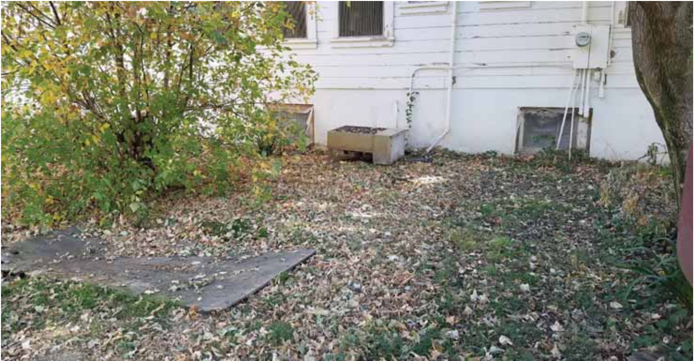
Photo 5: Western wall of the residence looking east.
