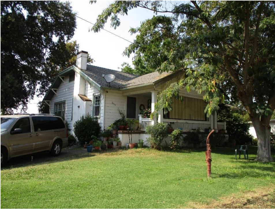
Figure 3. Photo showing the south and east elevations, facing northwest.
