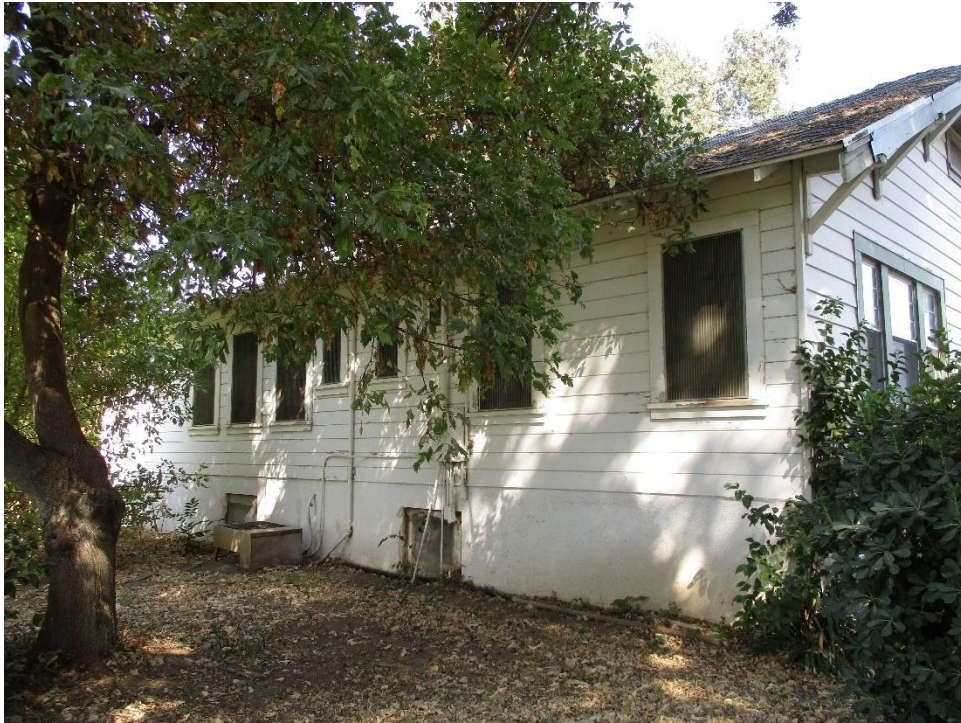
Figure 17. West elevation, facing northeast.
