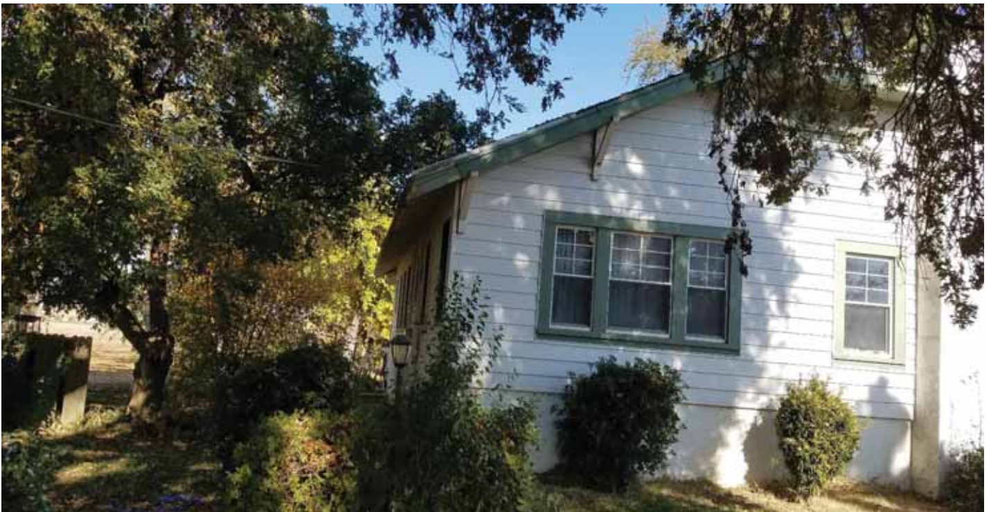
Photo 2: Looking north at the southwest corner of the residence.
