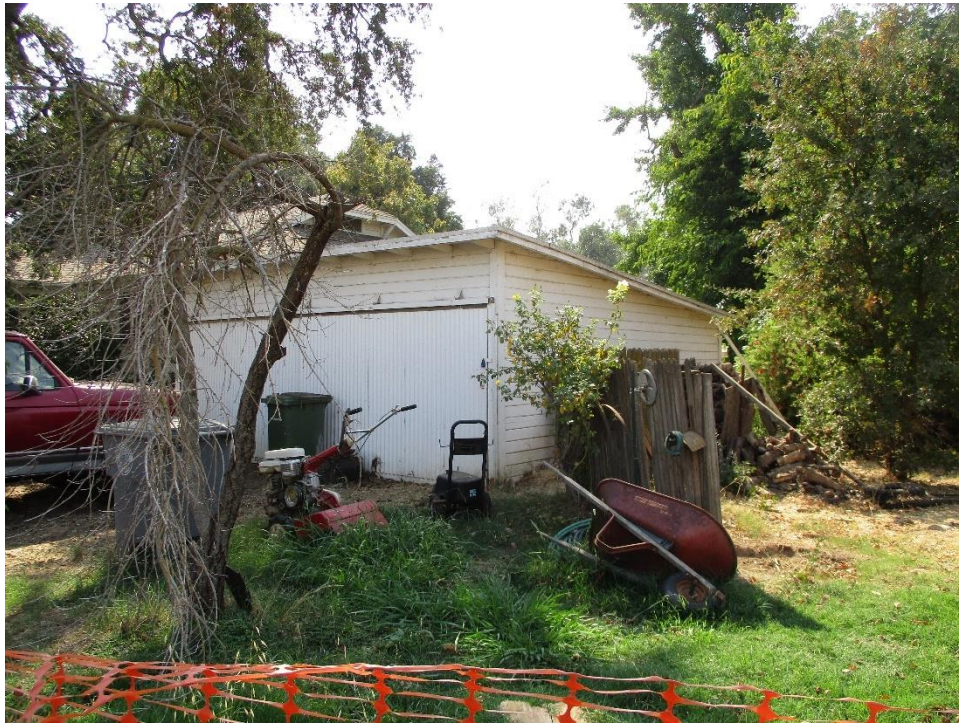
Figure 21. Photo showing the east and north elevations, facing southwest.
