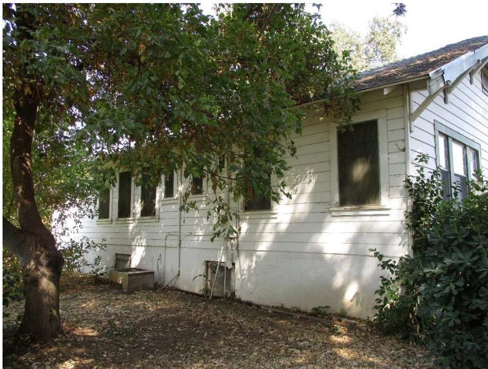
Figure 6. West elevation, facing northeast.
