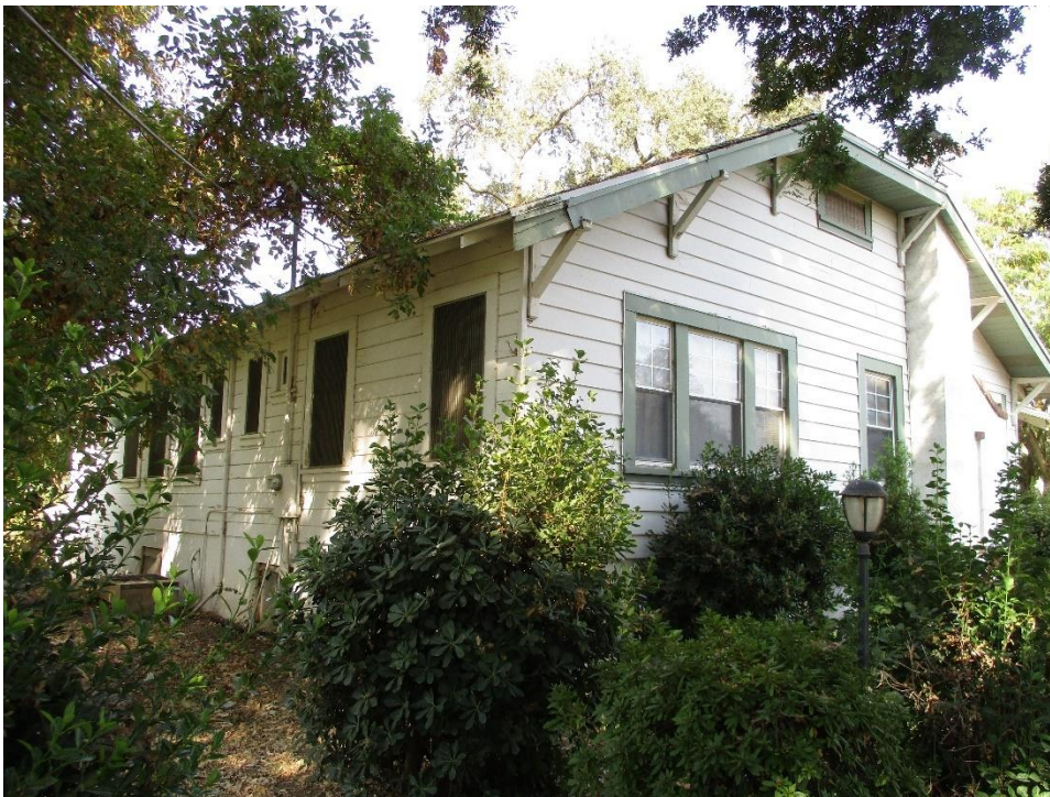
Figure 5. Photo showing the south and west elevations, facing northeast.
