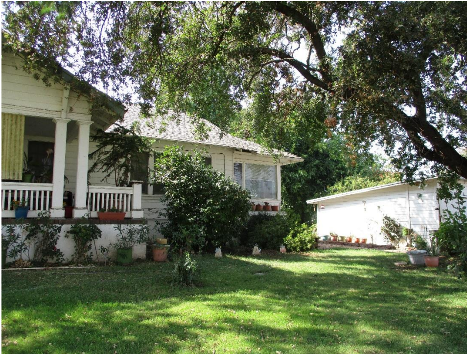
Figure 2. East elevation, facing northwest.
