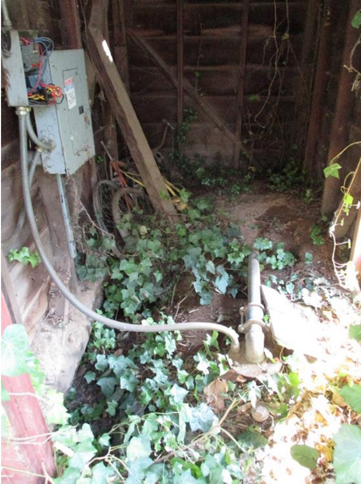
Figure 13. Photo showing the interior of the ca. 1920 well house building.
