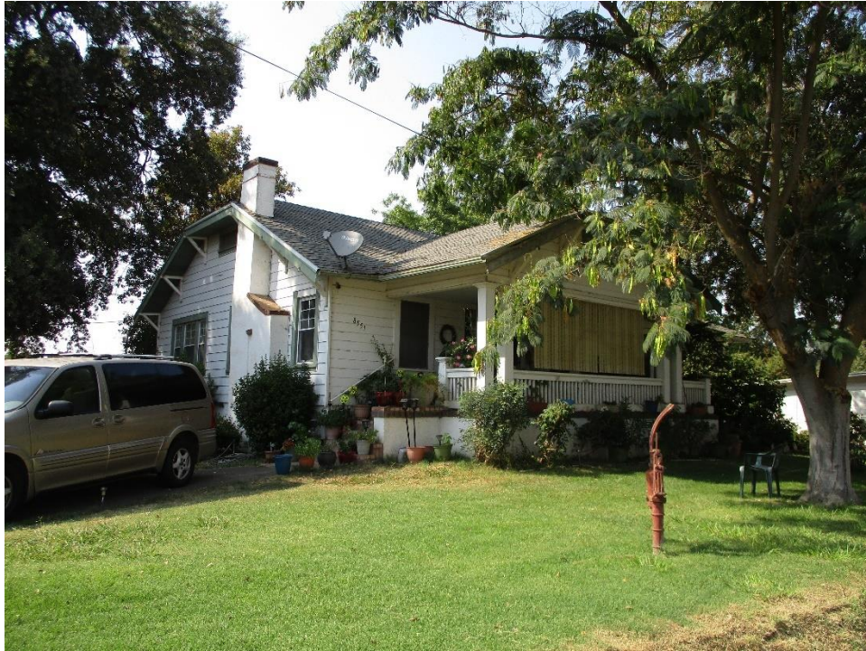
Figure 14. Photo showing the south and east elevations, facing northwest.
