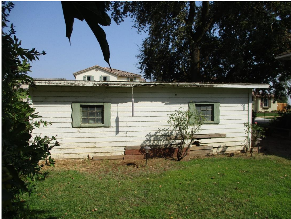
Figure 22. West elevation, facing east.
