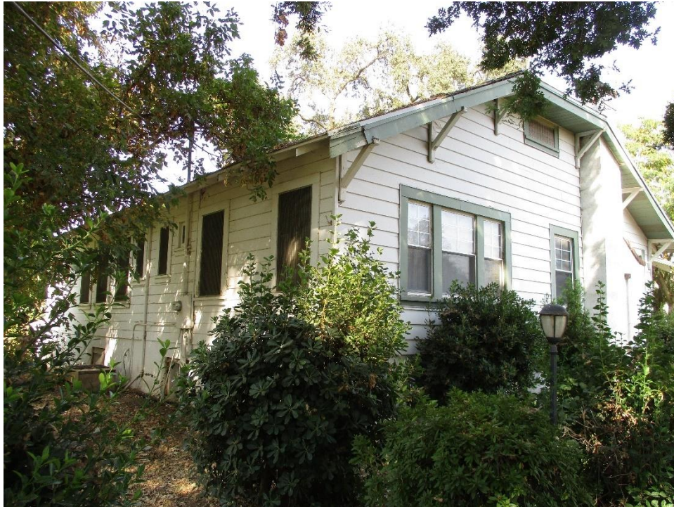
Figure 16. Photo showing the south and west elevations, facing northeast.
