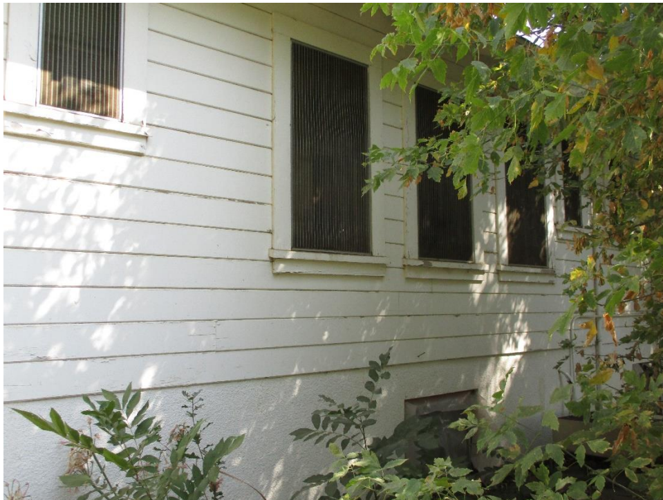
Figure 18. Photo showing the metal window screens.
