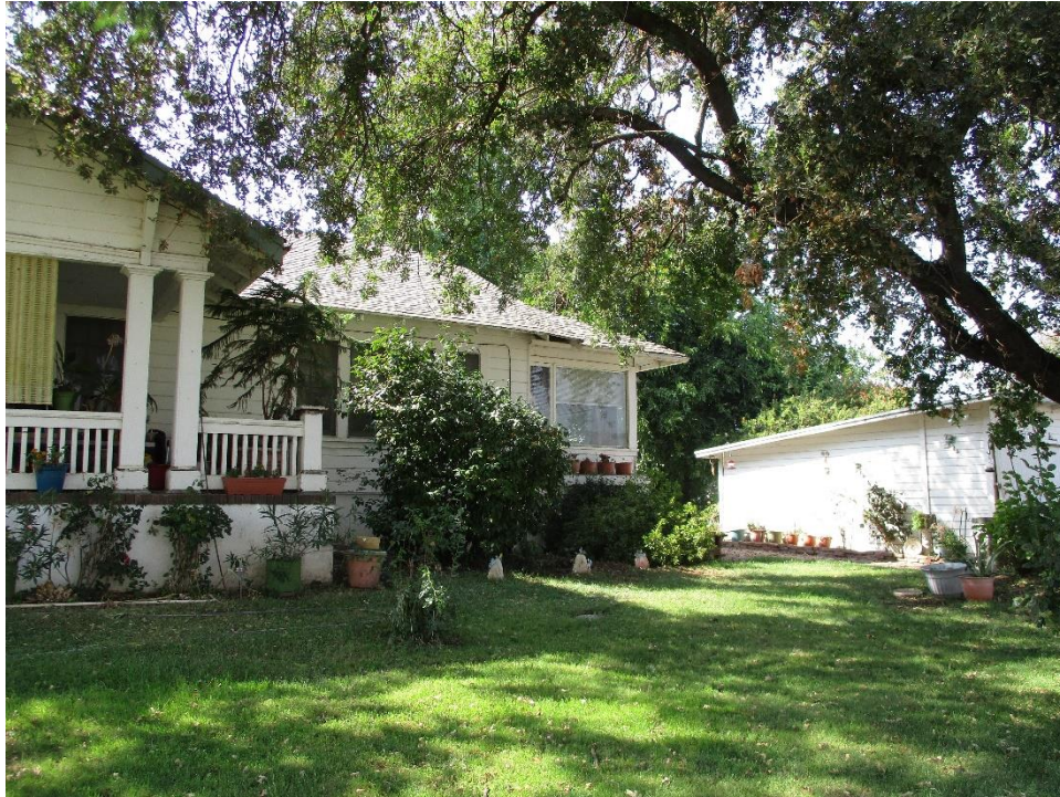
Figure 13. East elevation, facing northwest.
