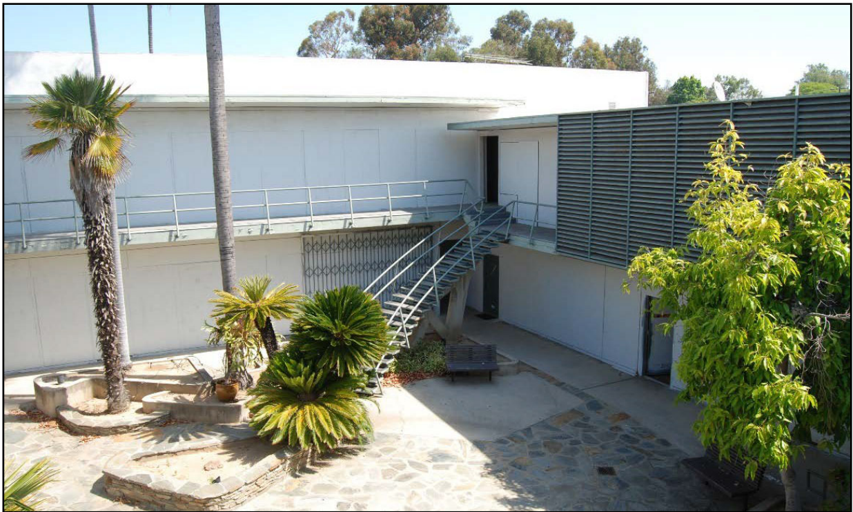
Barry Building, courtyard, view looking northeast.
