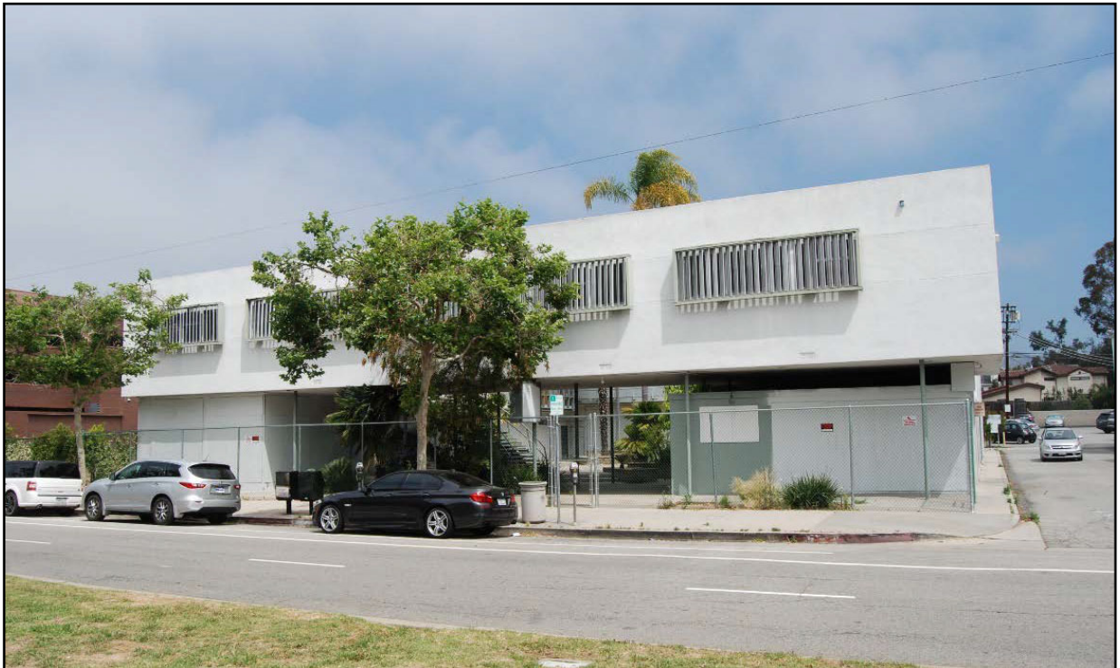
Barry Building, south façade, view looking northwest.
