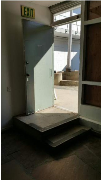
A first floor tenant's interior does not have a level landing at the entry door maneuvering space.
