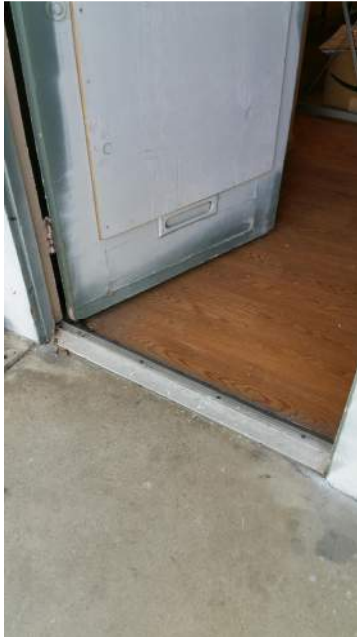
An original mail slot mounted at about 9” from the floor.
