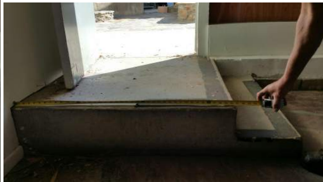
A first floor tenant's interior does not have a level landing at the entry door maneuvering space.
