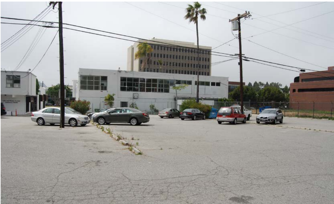
Photo 4: Barry Building, overall view southwest from parking lot. HRG
