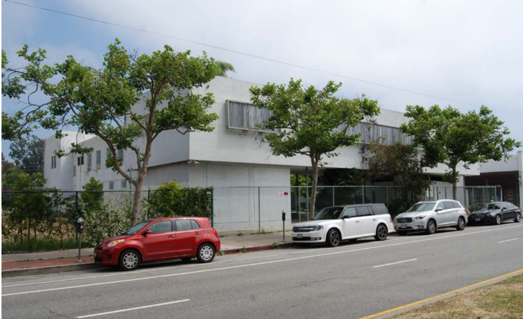
Photo 1: Barry Building, overall view northeast from San Vicente Boulevard. HRC
