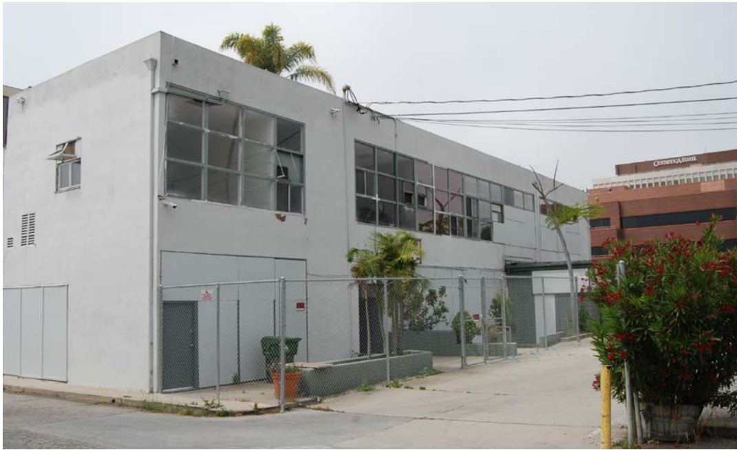
Photo 5: Barry Building, north façade, view southwest from parking lot. HRC
