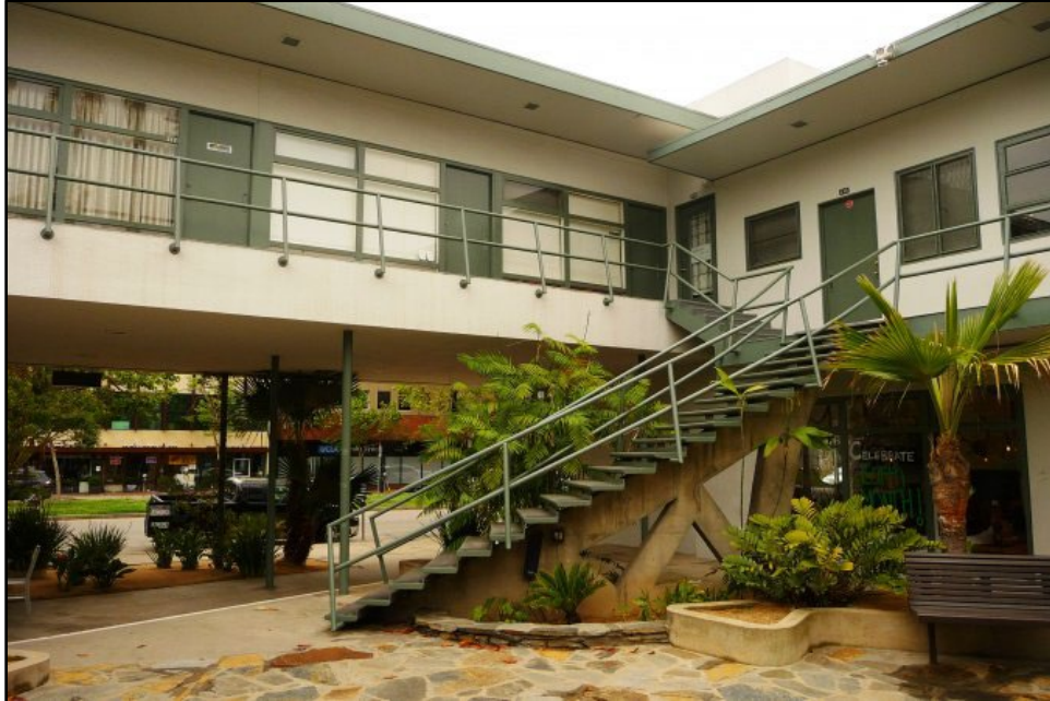
Figure A-9. Interior courtyard of the Barry Building facing southward (Los Angeles Conservancy 2020b).
