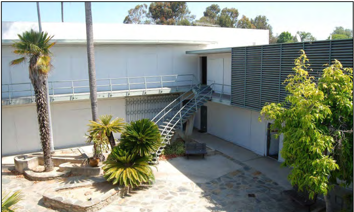
Barry Building, courtyard, view looking northeast.
