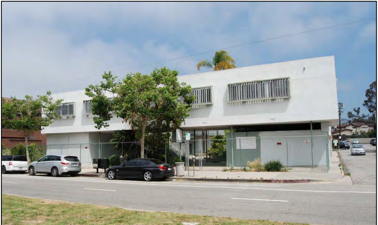
Barry Building, south façade, view looking northwest.
