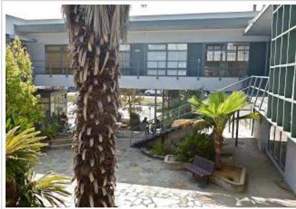
Above: The view from the back balcony towards the street side, showing the cantilevered 2nd floor.
