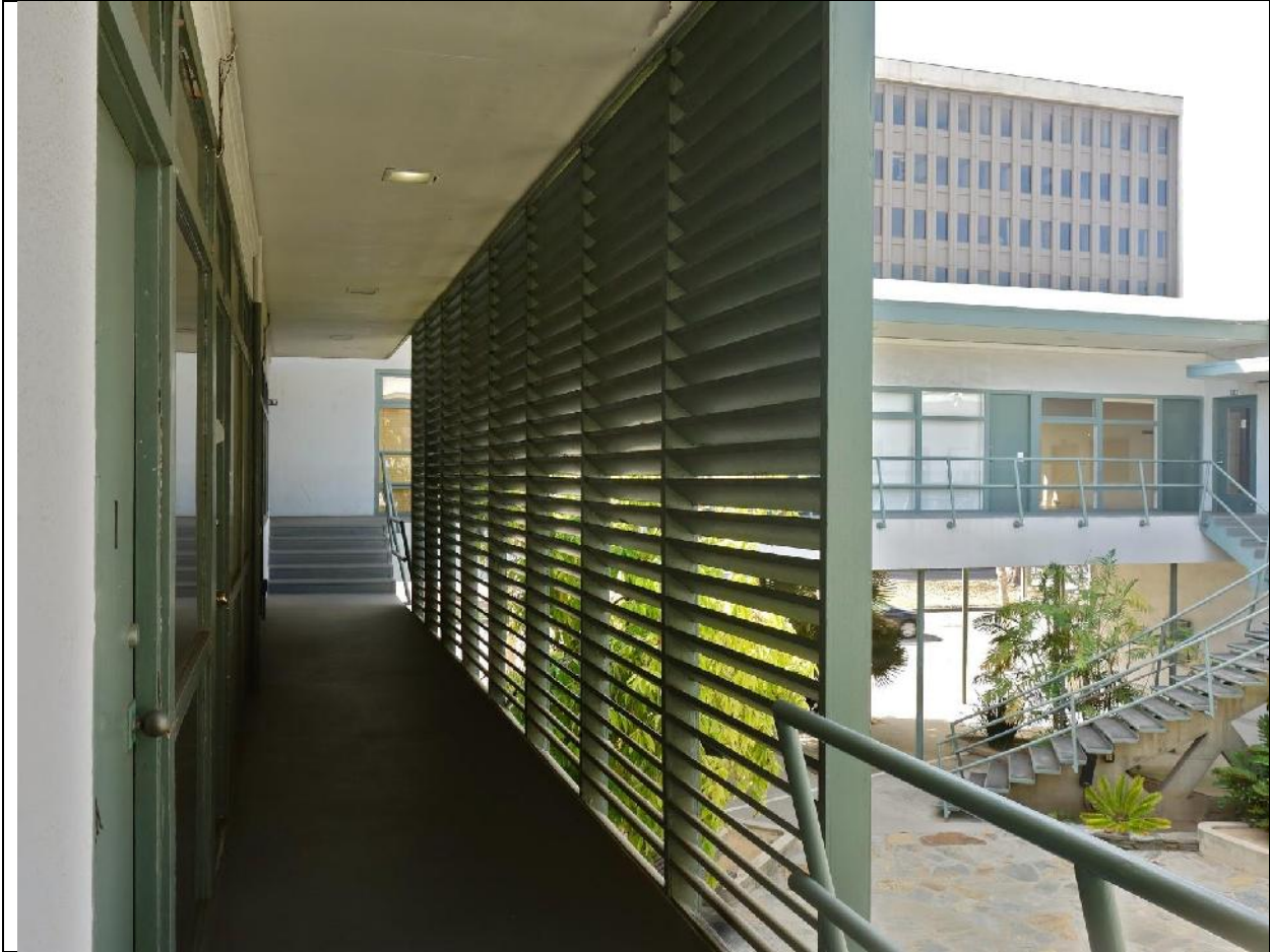
Above: Louvers block glare from the offices on the east side of the building. (photo by Laura Clayton Baker)
