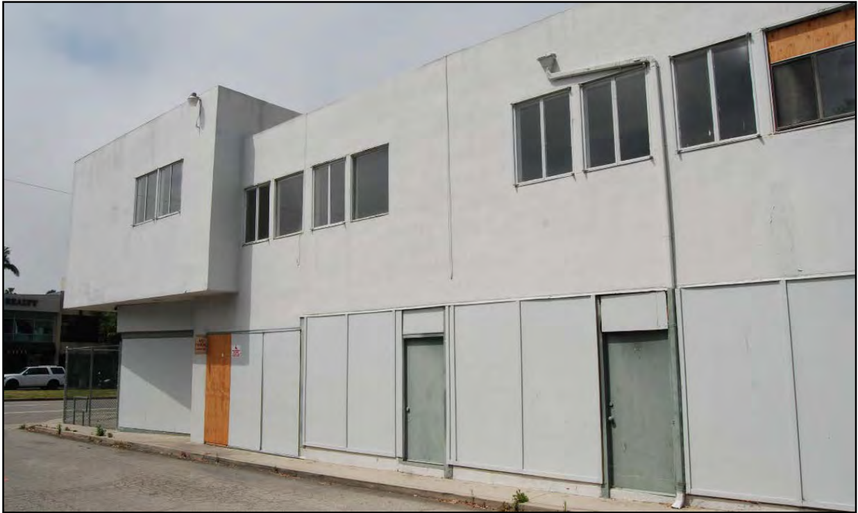
Barry Building, east façade, view looking southwest.
