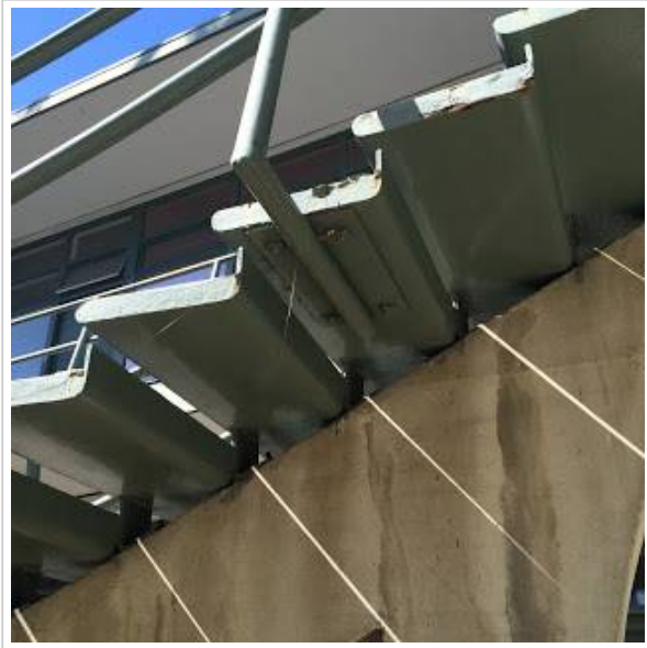
Above and below: The stairs are cantilevered from a central concrete spine.
