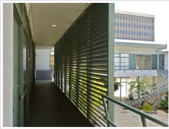
Above: Louvers block glare from the offices on the east side of the building.
