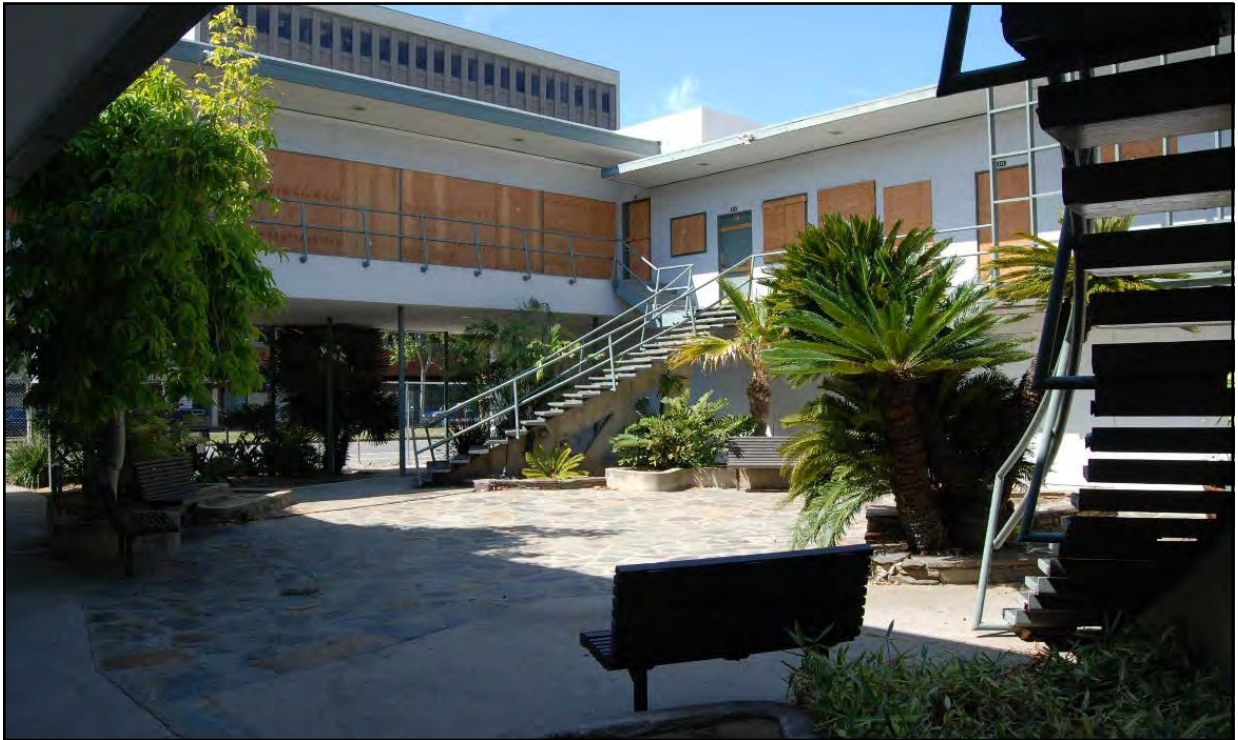
Barry Building, courtyard, view looking southwest.
