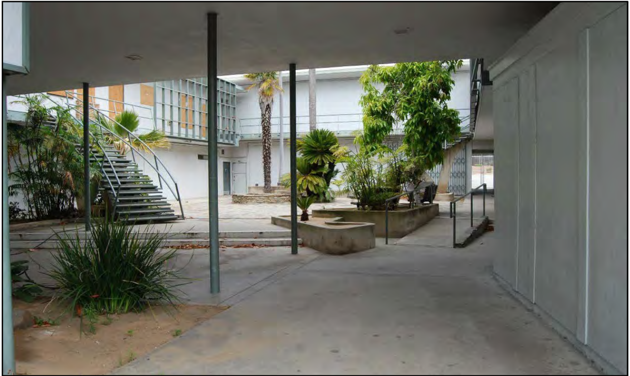
Barry Building, view looking northwest from street into courtyard.
