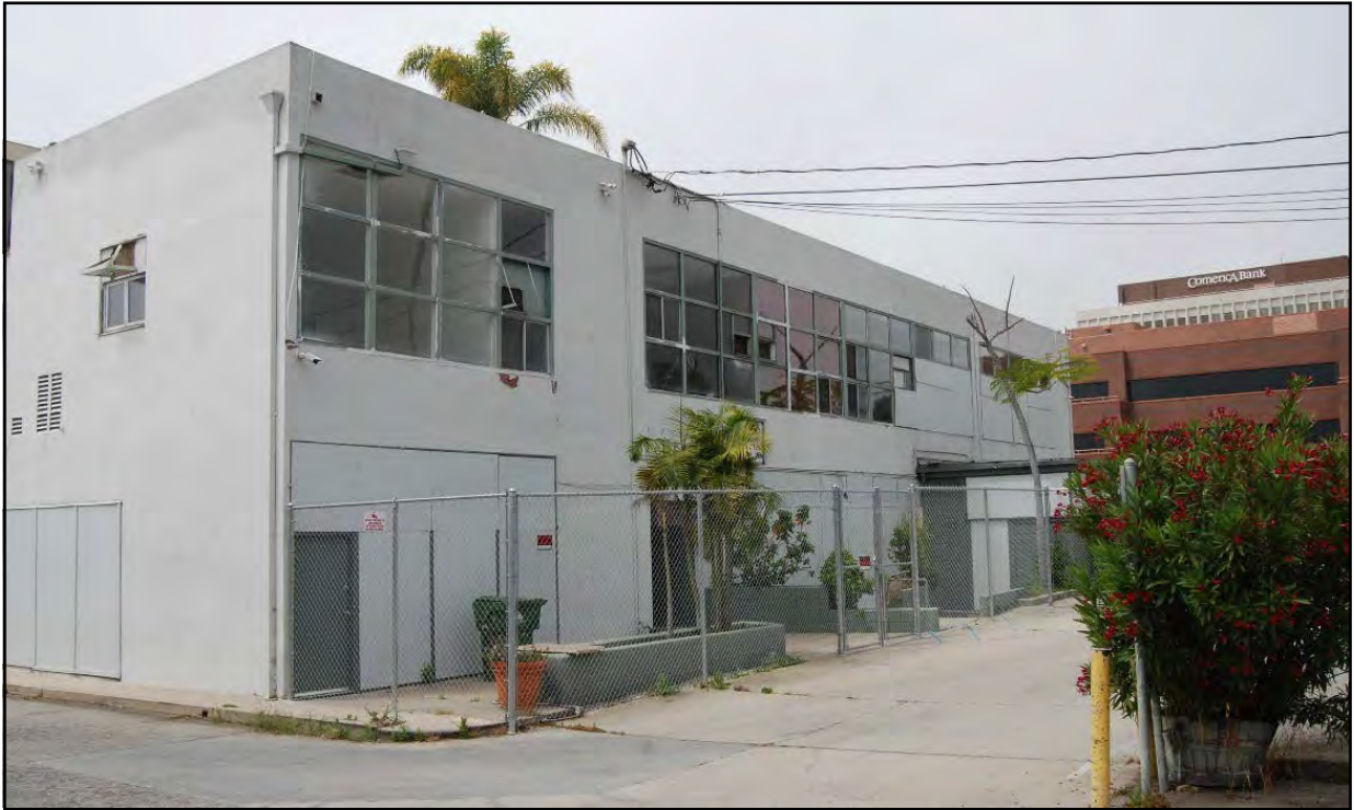
Barry Building, north façade, view looking southwest.
