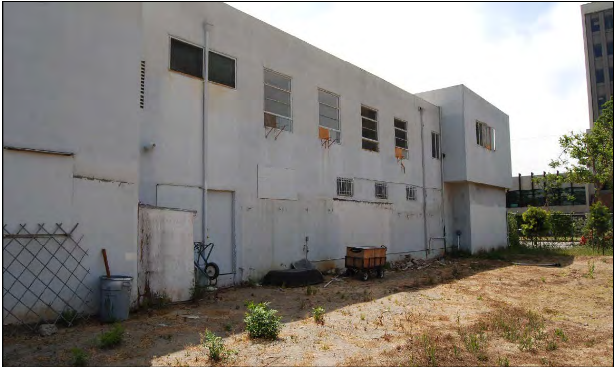
Barry Building, west façade, view looking southeast.
