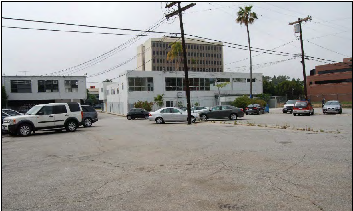
Barry Building, north and east façades, view looking southwest.
