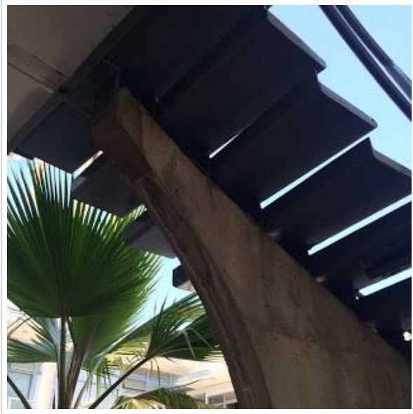
Above and below: The stairs are cantilevered from a central concrete spine.
