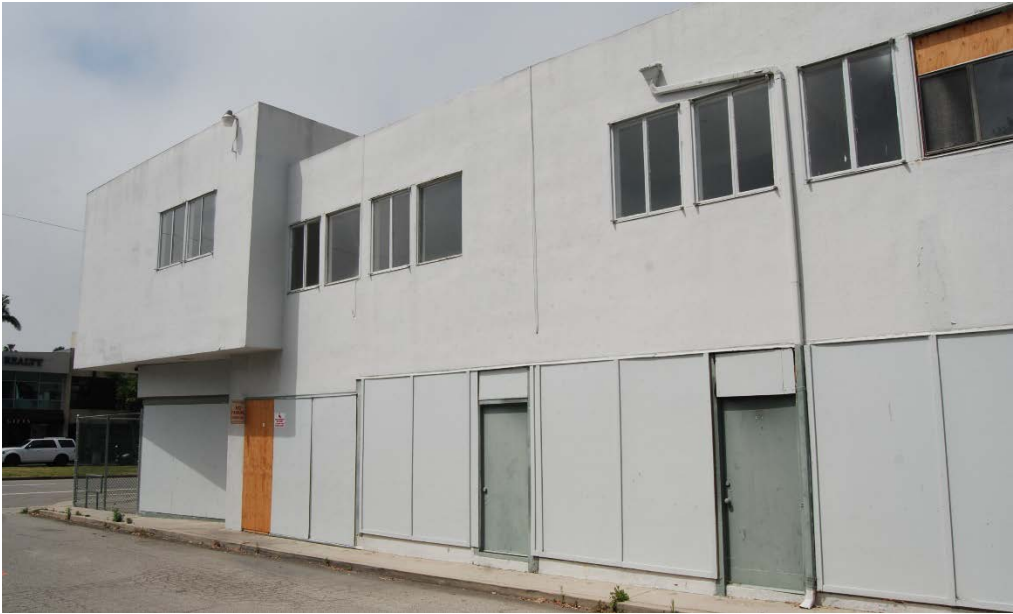
Figure 7: Barry Building, east façade, view looking southwest, May 2017 (HRG).
