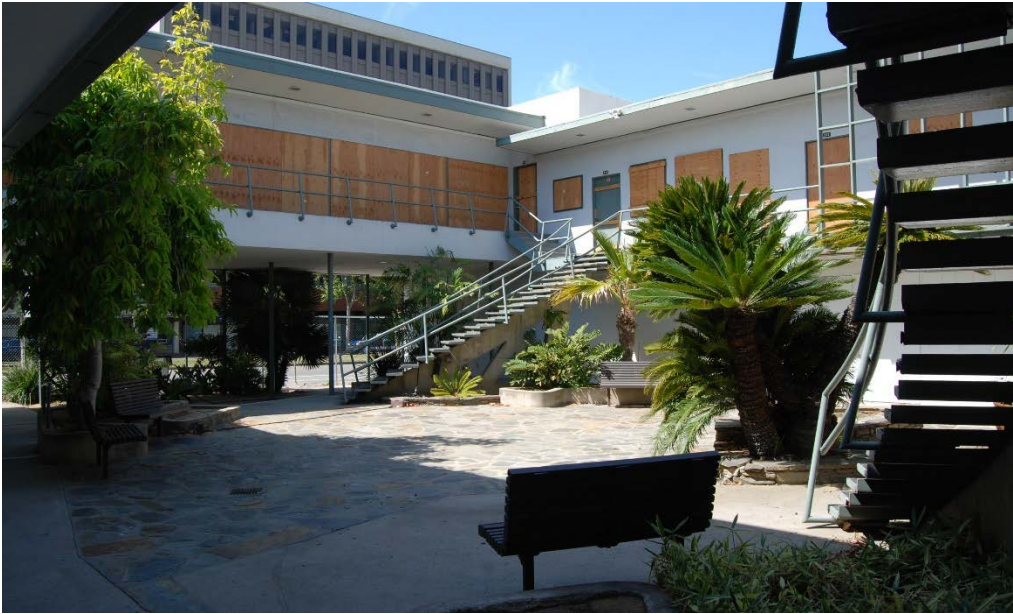
Figure 5: Barry Building, courtyard, view looking southwest, May 2017 (HRG).
