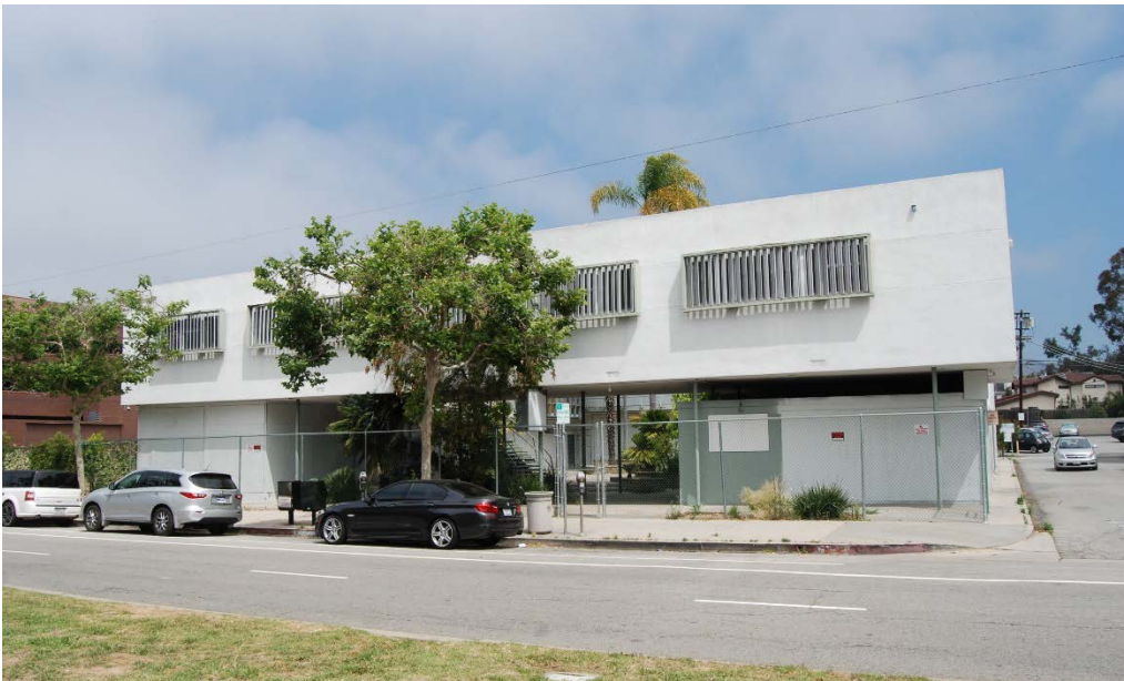
Figure 2: Barry Building, south façade, view looking northwest, May 2017 (HRG).
