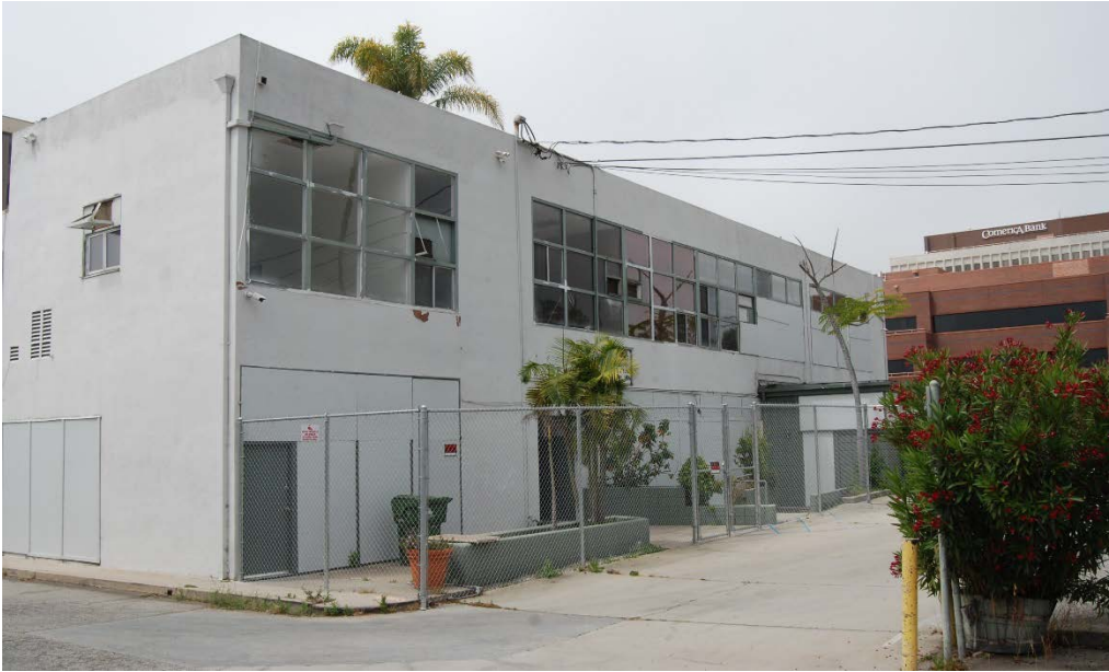
Figure 8: Barry Building, north façade, view looking southwest, May 2017 (HRG).
