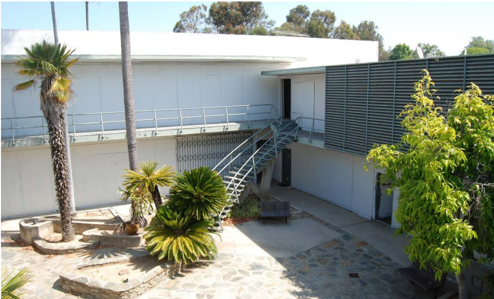
Figure 6: Barry Building, Courtyard, view looking northeast, May 2017 (HRG).
