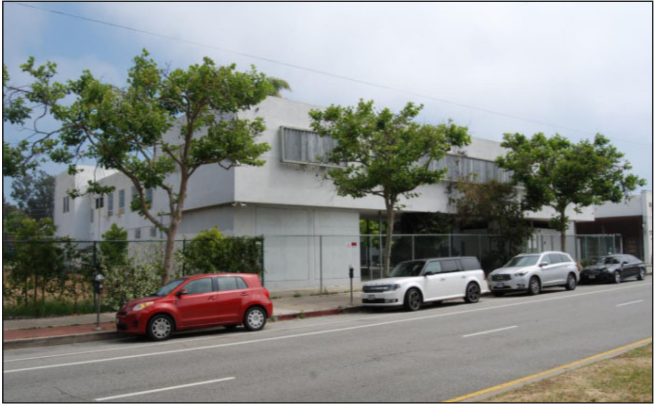
Photo 1 : Barry Building, overall view northeast from San Vicente Boulevard.
