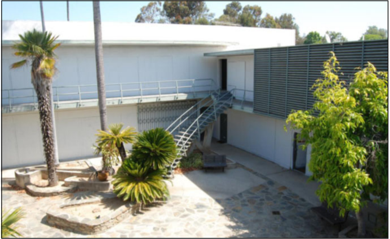
Photo 9: Barry Building, courtyard, view northeast from second floor balcony.
