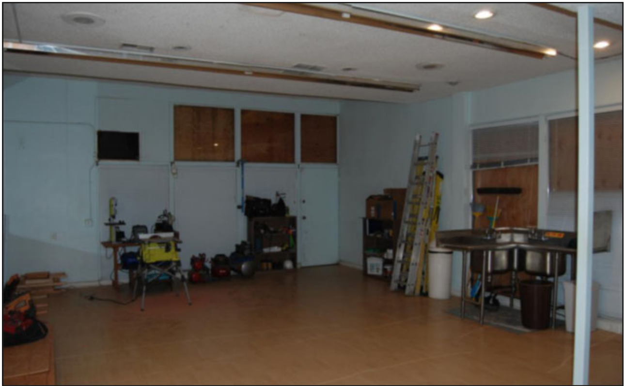
Photo 10: Barry Building, interior, typical first floor office suite, view northeast.
