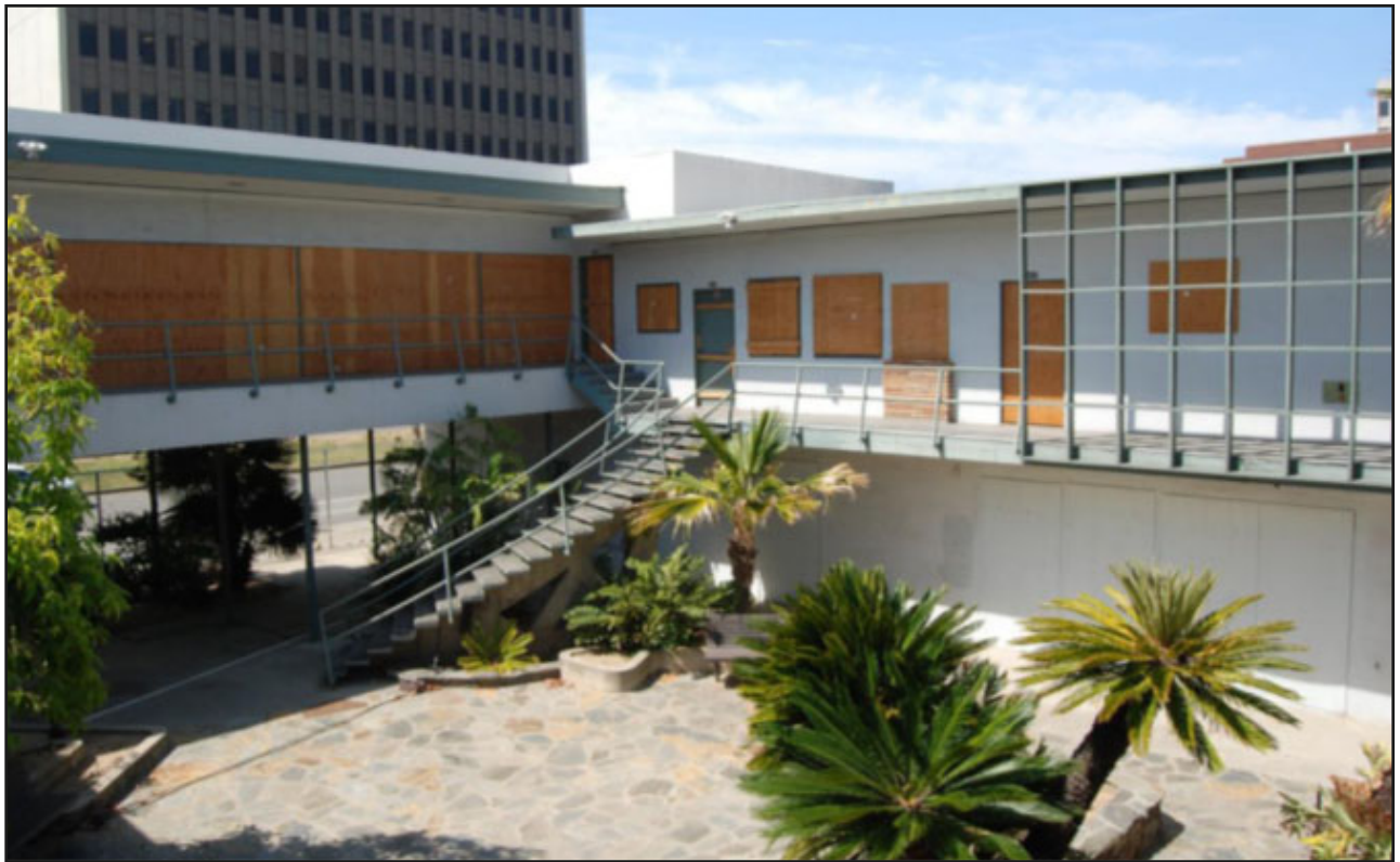
Photo 8: Barry Building, courtyard, view southwest from second floor balcony.
