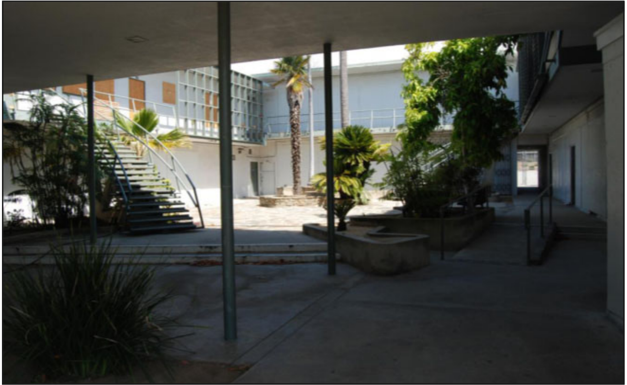
Photo 7: Barry Building, courtyard, view northwest from San Vicente Boulevard.
