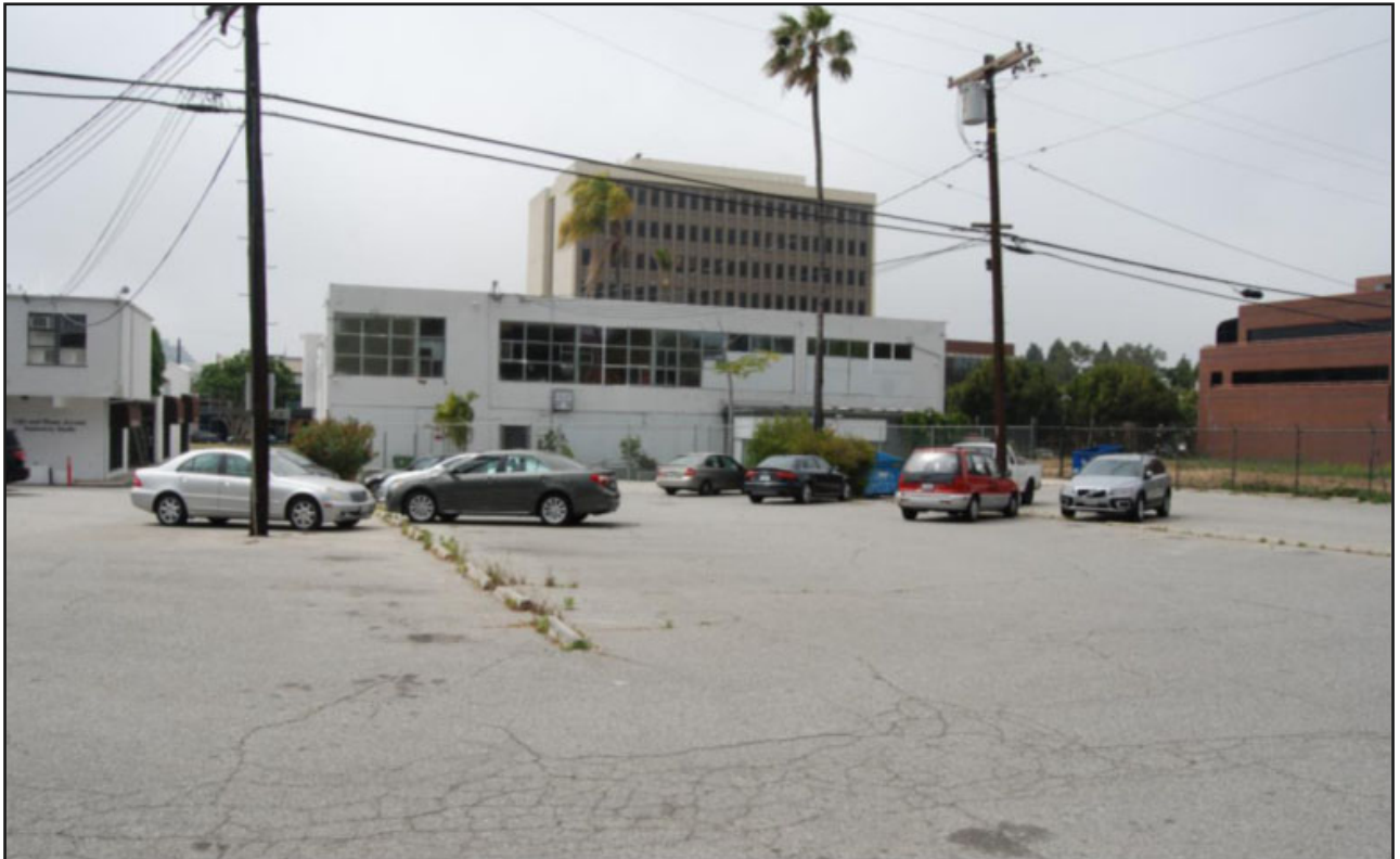
Photo 4: Barry Building, overall view southwest from parking lot.
