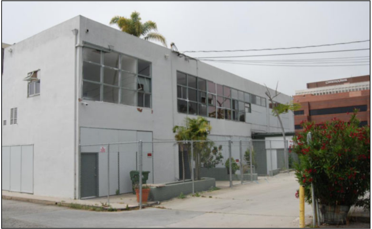
Photo 5: Barry Building, north façade, view southwest from parking lot.
