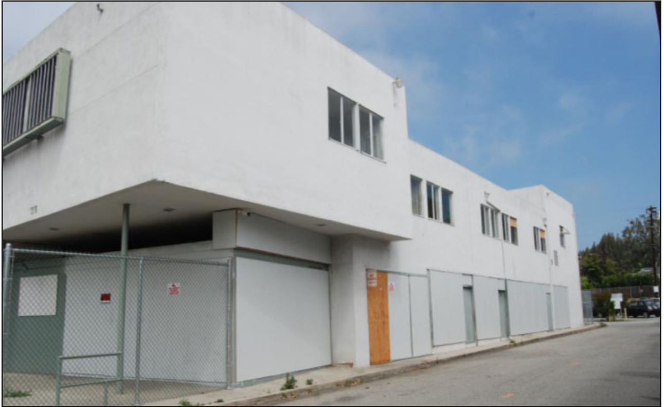
Photo 3: Barry Building, east façade and driveway, view northwest from San Vicente Boulevard.
