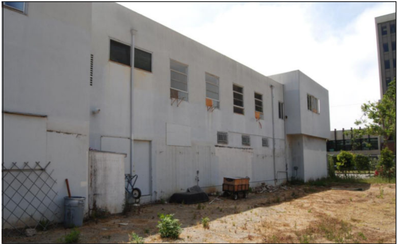
Photo 6: Barry Building, west façade, view southeast from adjacent parcel.
