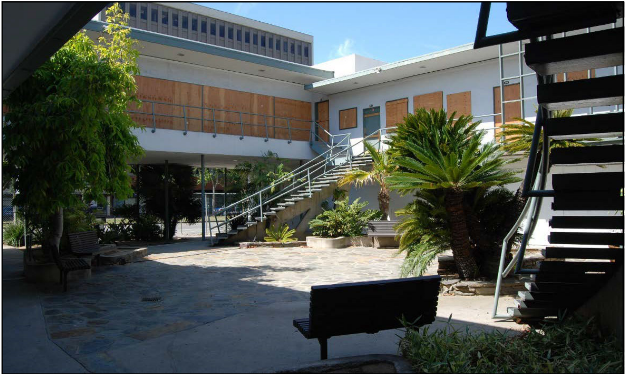
Barry Building, courtyard, view looking southwest.
