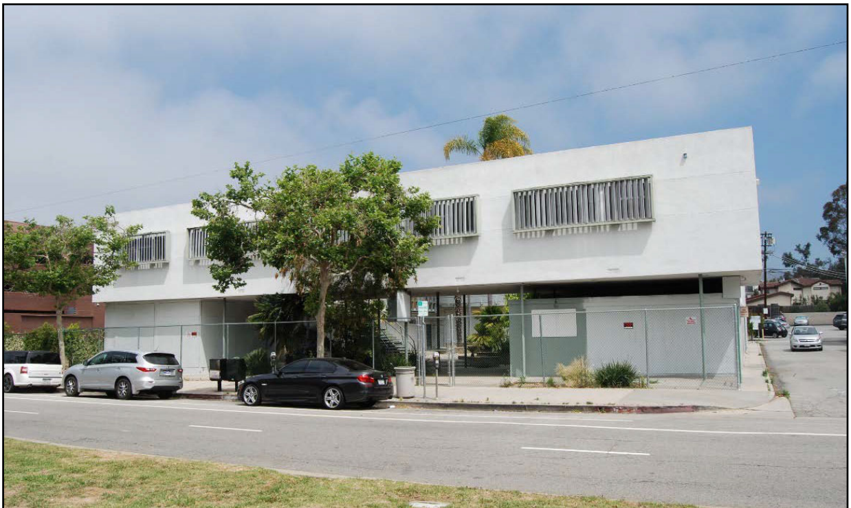
Barry Building, south façade, view looking northwest.
