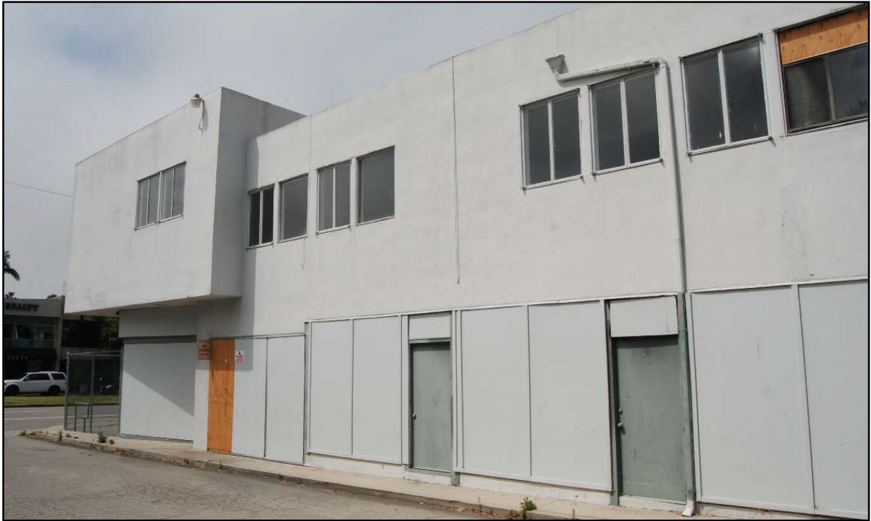
Barry Building, east façade, view looking southwest.
