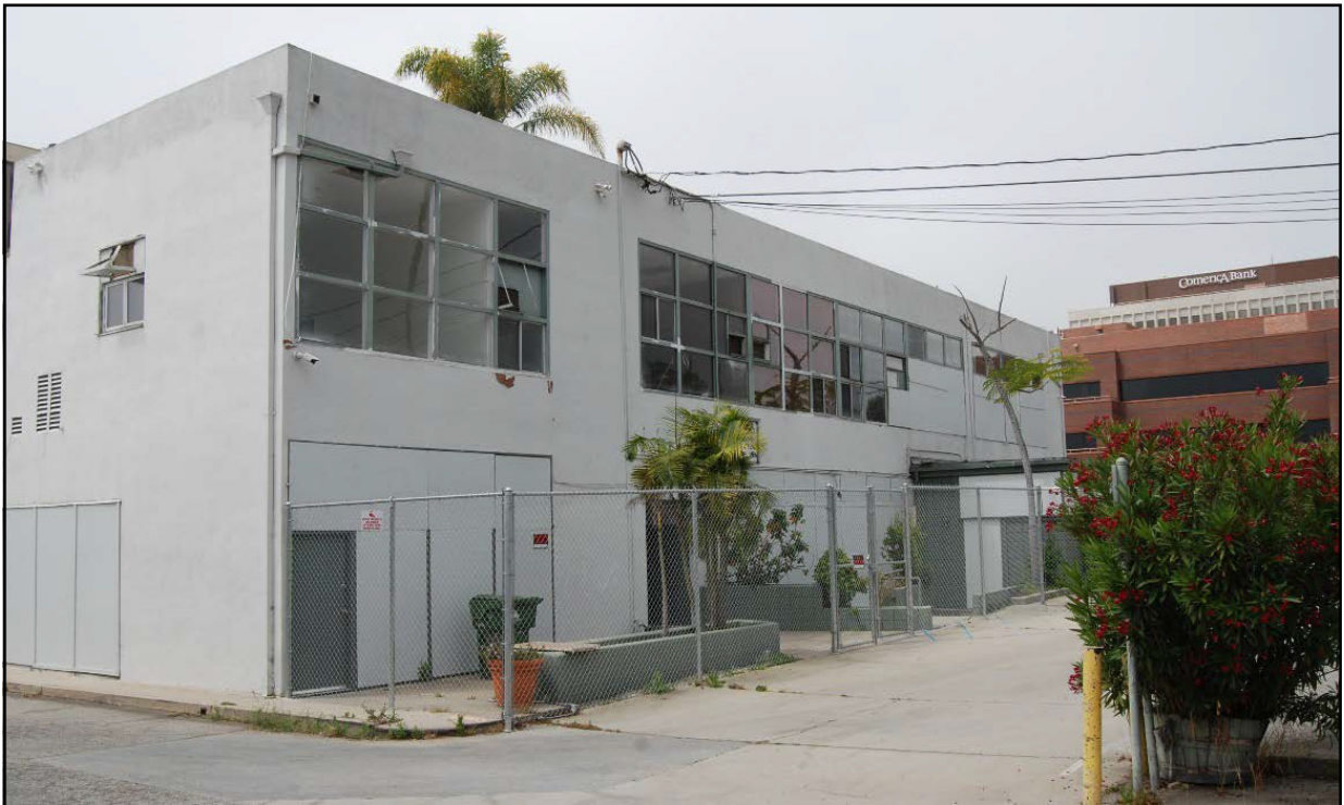
Barry Building, north façade, view looking southwest.
