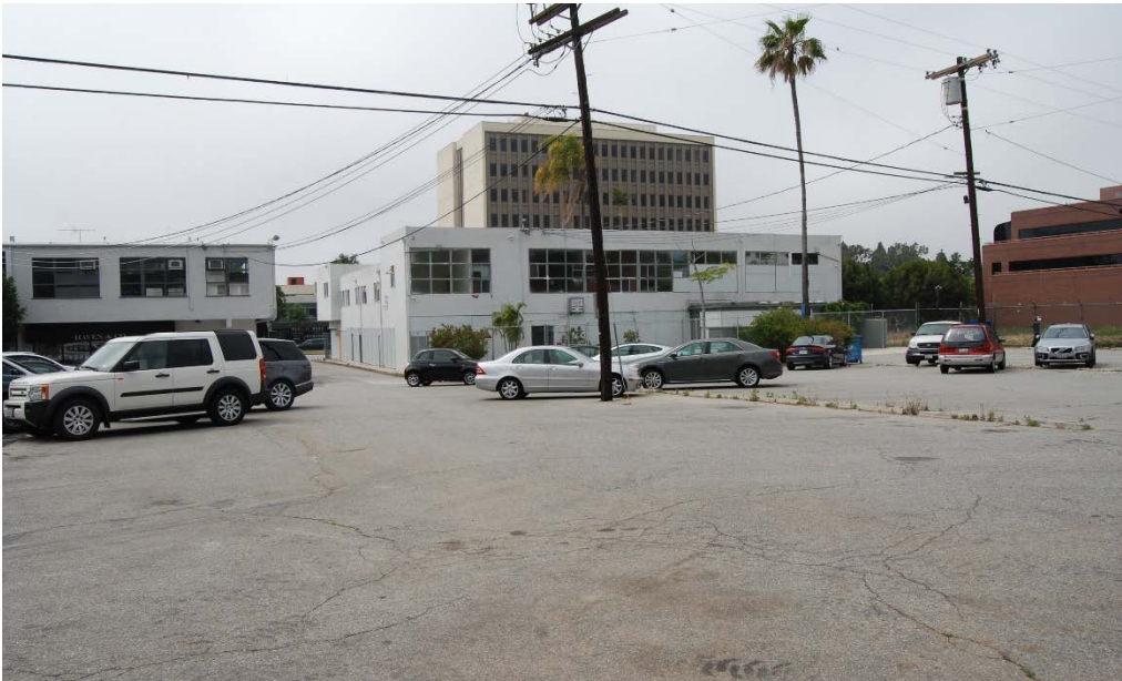
Figure 10: Barry Building, north and east façades, view looking southwest, May 2017 (HRG).
