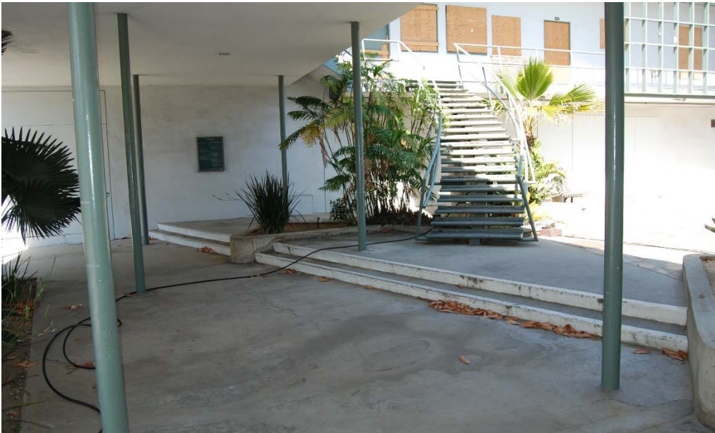
Figure 4: Barry Building, view looking northwest of courtyard entrance, May 2017 (HRG).
