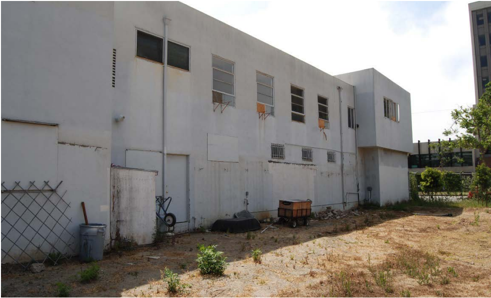
Figure 9: Barry Building, west façade, view looking southeast, May 2017 (HRG).
