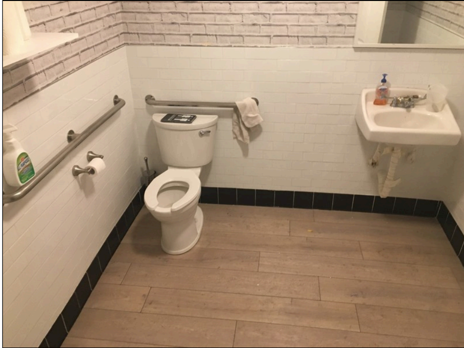
Photo 6: Representative view of restroom.
