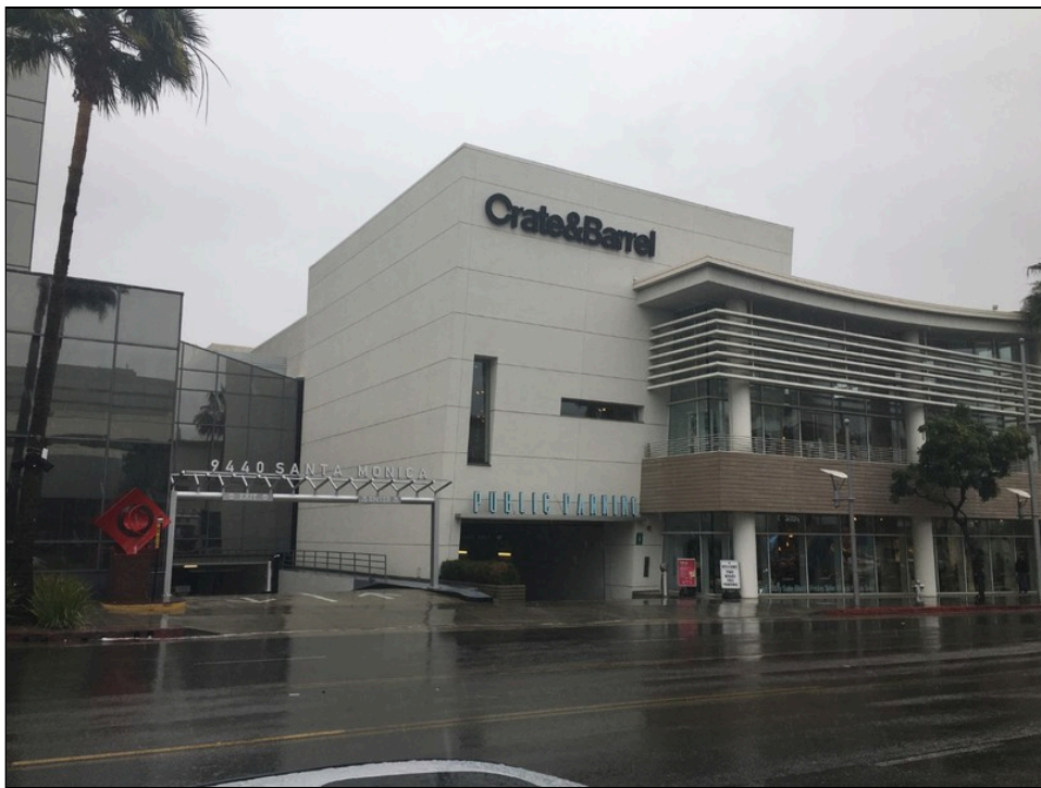
Photo 22: View of northeast adjacent properties.
