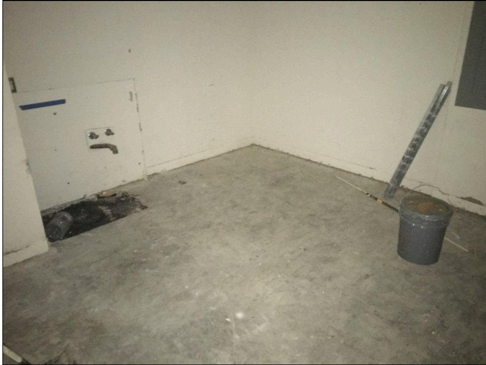
Photo 12: View of vacant room.
