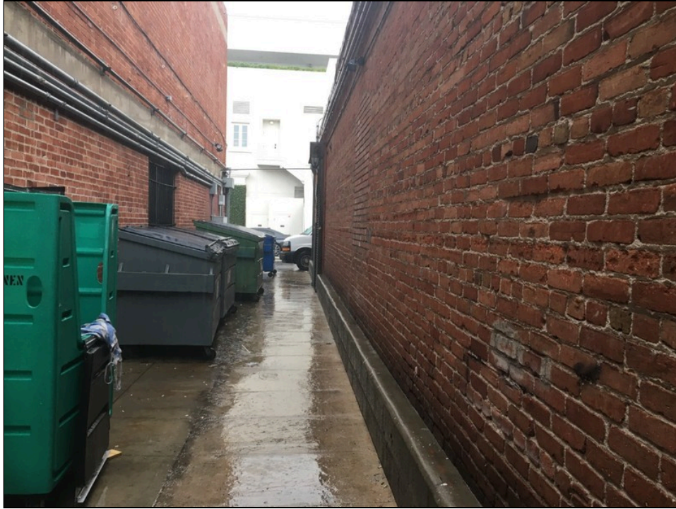
Photo 19: View of southern concrete-paved walkway on the southwest portion of the subject property looking southwest.
