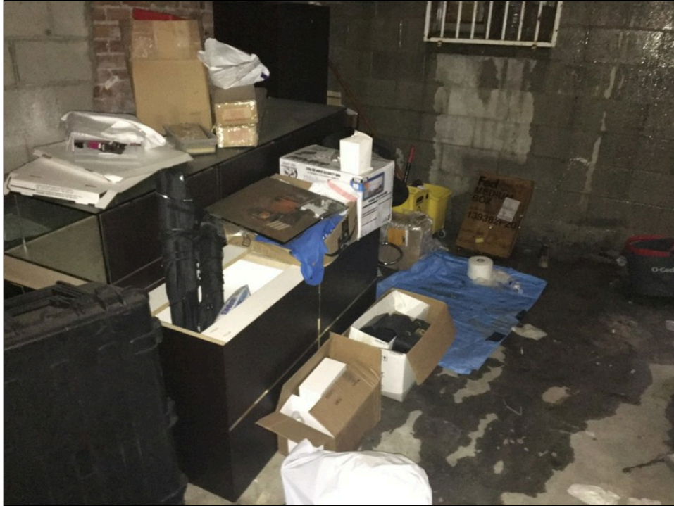
Photo 18: View of interior of storage area on the central portion.
