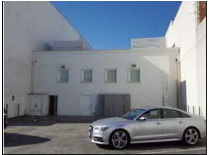
2. The east side of the subject property.
