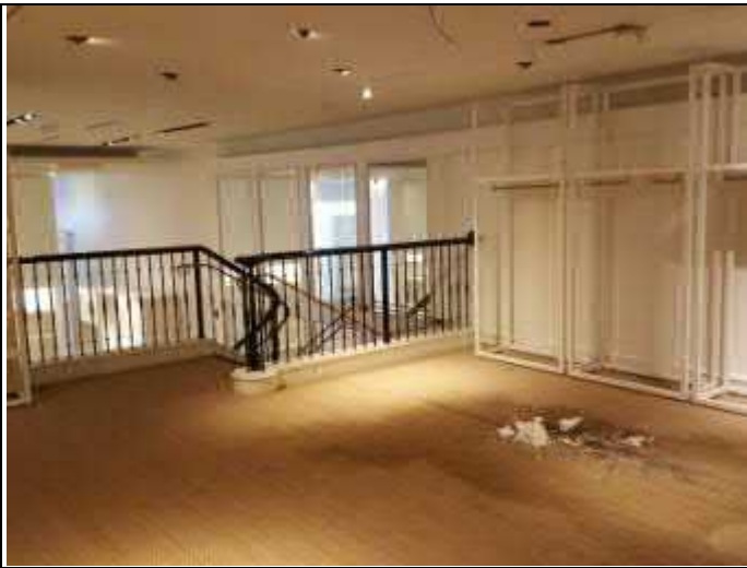
13. Mezzanine area with ceiling material on floor.
