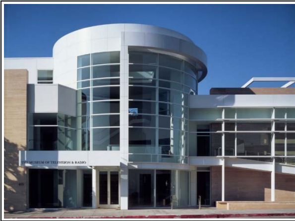
Detail of entrance rotunda, n.d. Note signage with original name (Richard Meier and Partners LLP).
