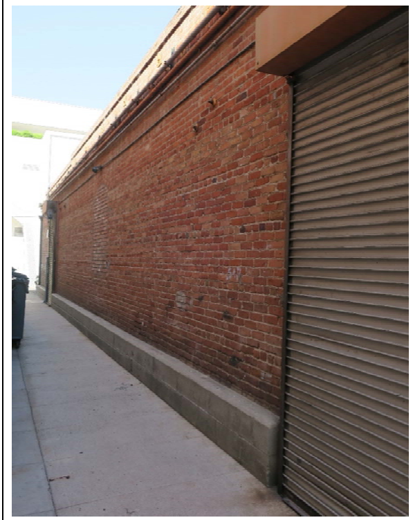
Side (southeast) façade, view west (ARG, 2020)
