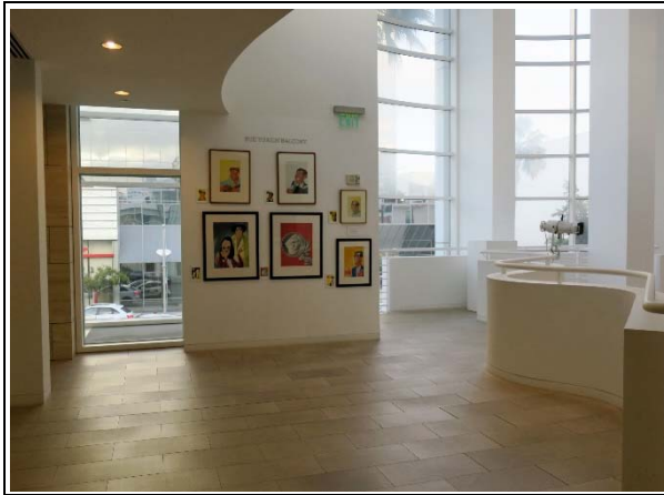
Second floor balcony. Note undulation (ARG, 2019).
