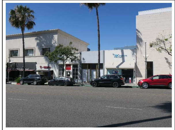
Primary façade, view southwest (ARG, 2020)
