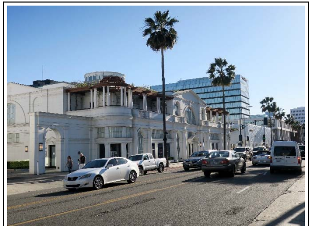
Northwest elevation, view southwest (ARG, 2019).
