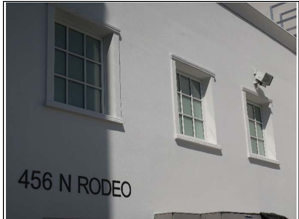
Detail of upper-story windows and painted signage on rear façade (ARG, 2020)
