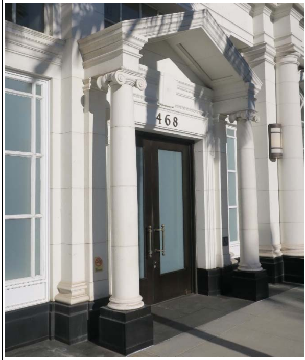
Detail of entrance on primary elevation, view southeast. Note columns and pediment (ARG, 2019).
