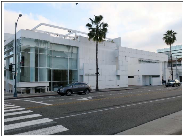
Northwest elevation, view southwest (ARG, 2019).
