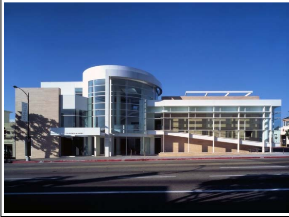
Primary (northeast) elevation, view southwest, n.d. (Richard Meier and Partners LLP).
