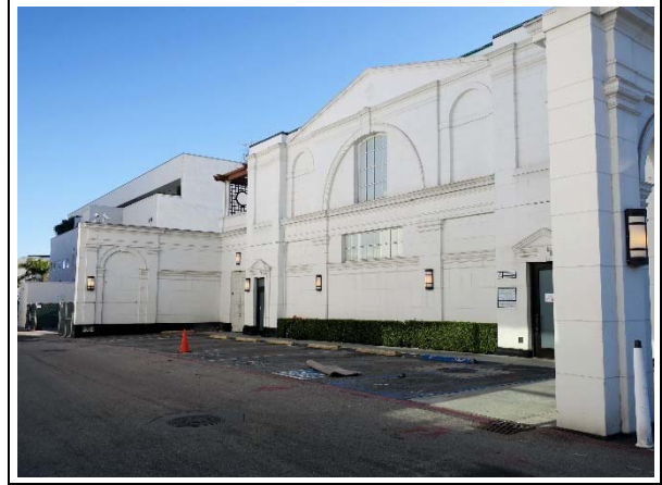
Northeast elevation and parking, view southwest. Note wing wall with blind arch (ARG, 2019).
