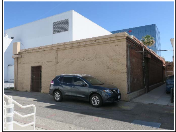
Rear façade, view northeast (ARG, 2020)
