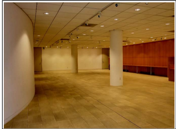
Second floor console center. Note light maple accents (ARG, 2019).
