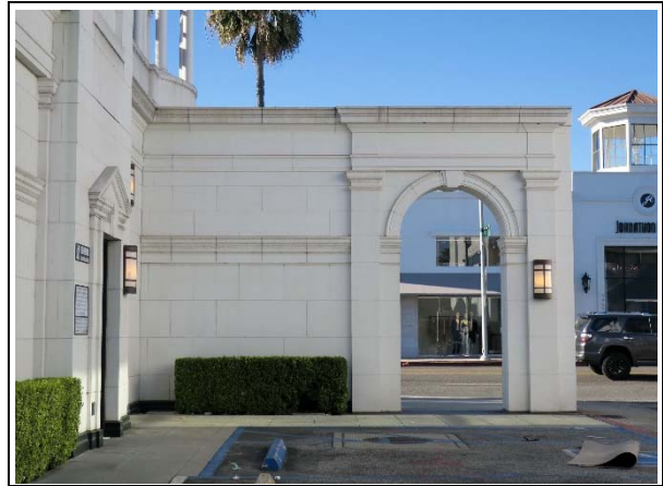
Projecting wing wall with rounded arch, pilasters, and entablature, view northwest (ARG, 2019).
