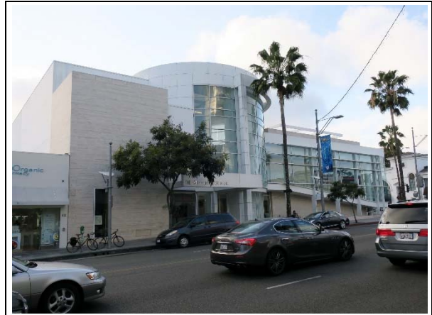
Primary (northeast) elevation, view northwest (ARG, 2019).
