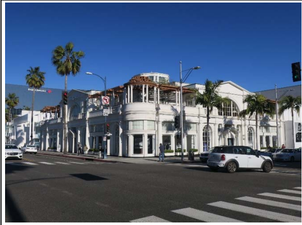
Primary (southwest) and northwest elevations, view east (ARG, 2019).
