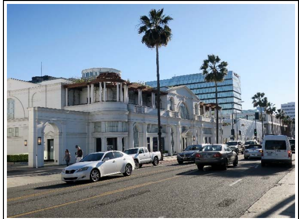
Northwest elevation, view southwest (ARG, 2019).
