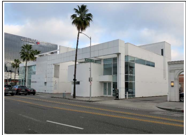
Northwest elevation, view east (ARG, 2019).
