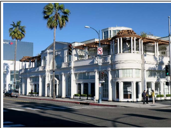
Northwest elevation, view east (ARG, 2019).
