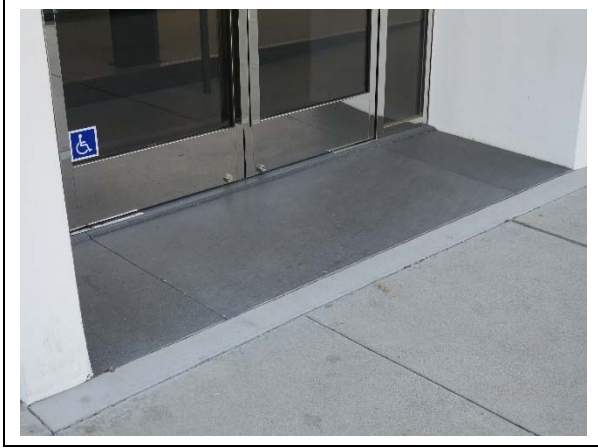
Detail of stone entrance threshold on primary façade (ARG, 2020)
