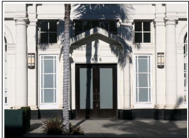
Detail of entrance on primary elevation, view northeast (ARG, 2019).
