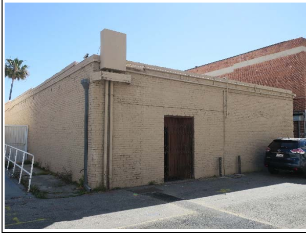
Rear (southwest) façade, view east (ARG, 2020)
