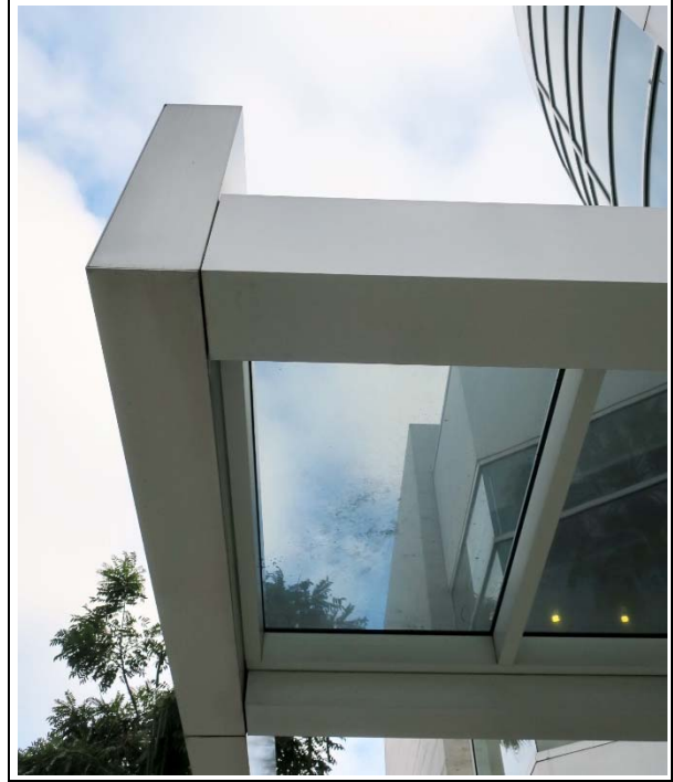
Glazed, cantilevered canopy above primary entrance (ARG, 2019).
