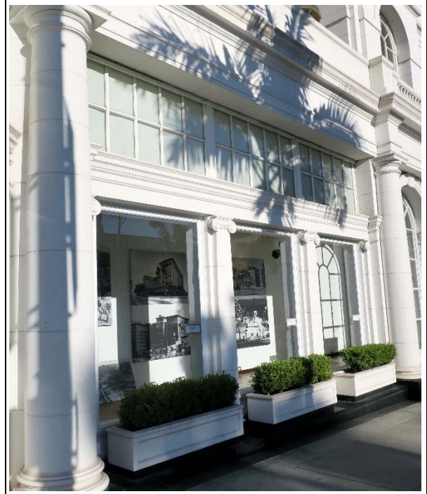
Detail of storefront system on primary elevation, view southeast (ARG, 2019).
