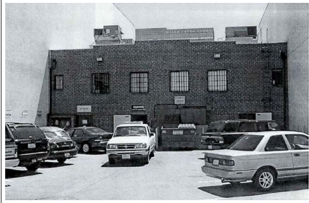
Subject building, rear façade, 1999 (included in building permit record, City of Beverly Hills Community Development Department)
