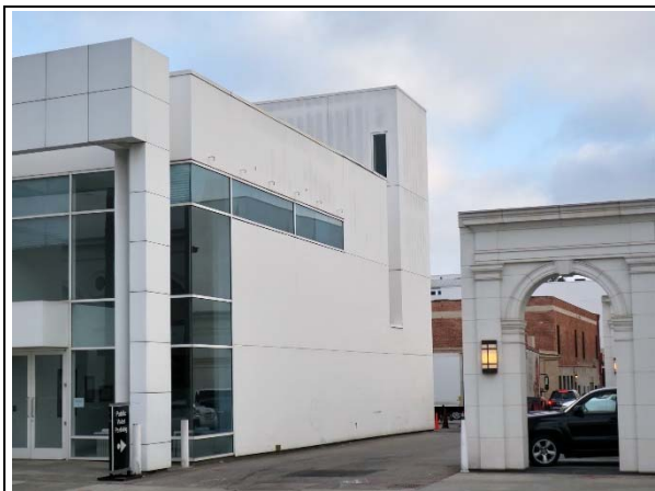
Southwest elevation, view southeast (ARG, 2019).
