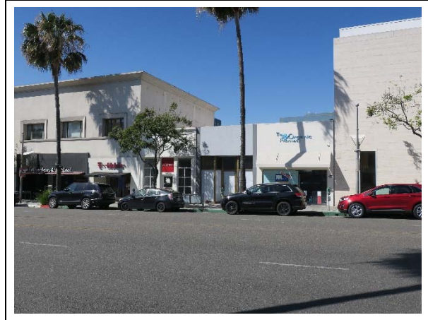
Primary façade, view southwest (ARG, 2020)
