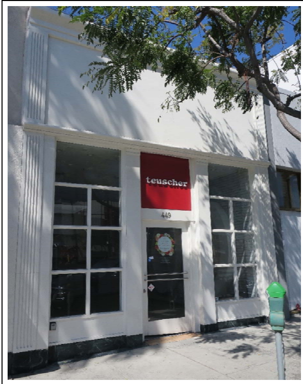
Detail of south storefront (449 N Beverly Dr) on primary façade (ARG, 2020)
