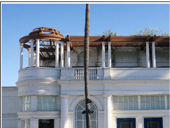
Detail of pergola with column supports on northwest elevation, view southeast (ARG, 2019).
