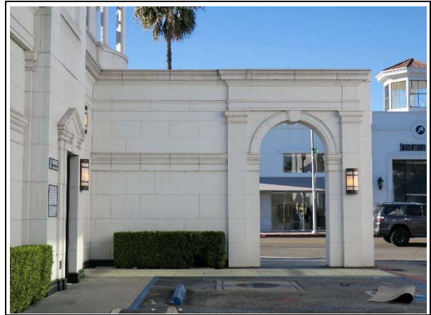
Projecting wing wall with rounded arch, pilasters, and entablature, view northwest (ARG, 2019).
