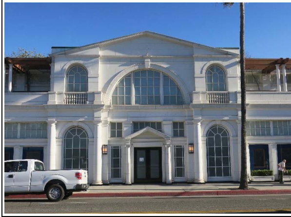
Prominent central bay with pediment on northwest elevation, view southeast (ARG, 2019).
