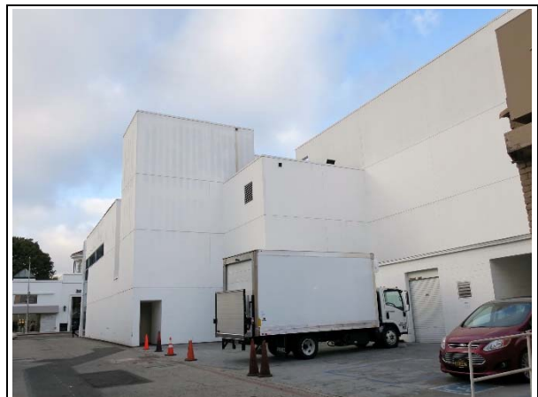
Southwest elevation, view north (ARG, 2019).
