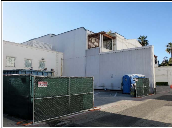
Southeast elevation, view northwest (ARG, 2019).
