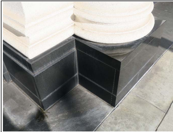
Detail of polished stone at base of building (ARG, 2019).
