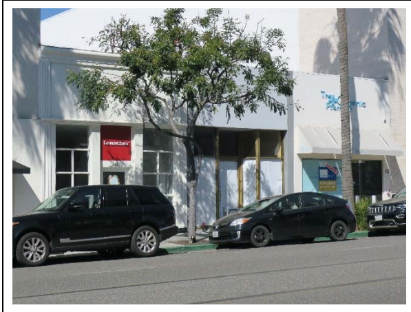
Primary (northeast) façade, view northwest (ARG, 2020)
