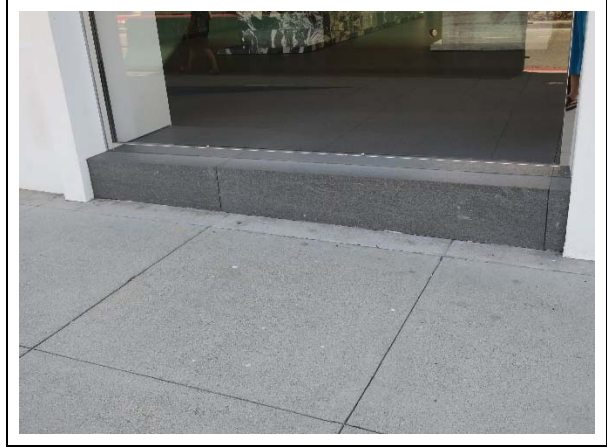
Detail of stone bulkhead on primary façade (ARG, 2020)
