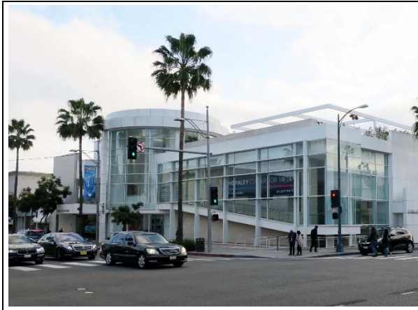
Primary (northeast) elevation, view southeast (ARG, 2019).
