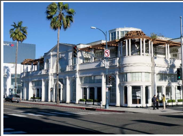
Northwest elevation, view east (ARG, 2019).
