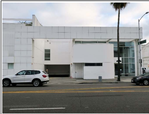
Driveway to subterranean parking garage, northwest elevation, view southeast (ARG, 2019).
