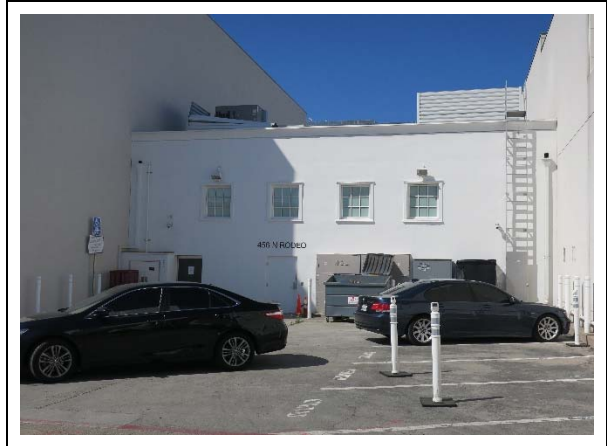
Rear (northeast) façade, view south. Note parking lot in foreground (ARG, 2020)
