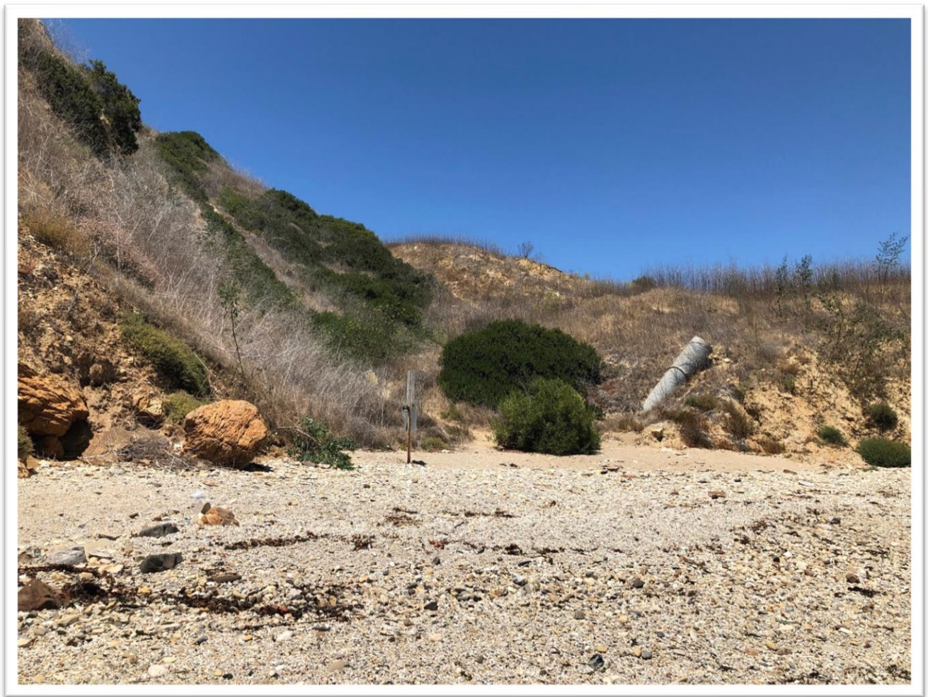
Photograph 5: Overview of proposed Hydrauger A6 location. View to north.
