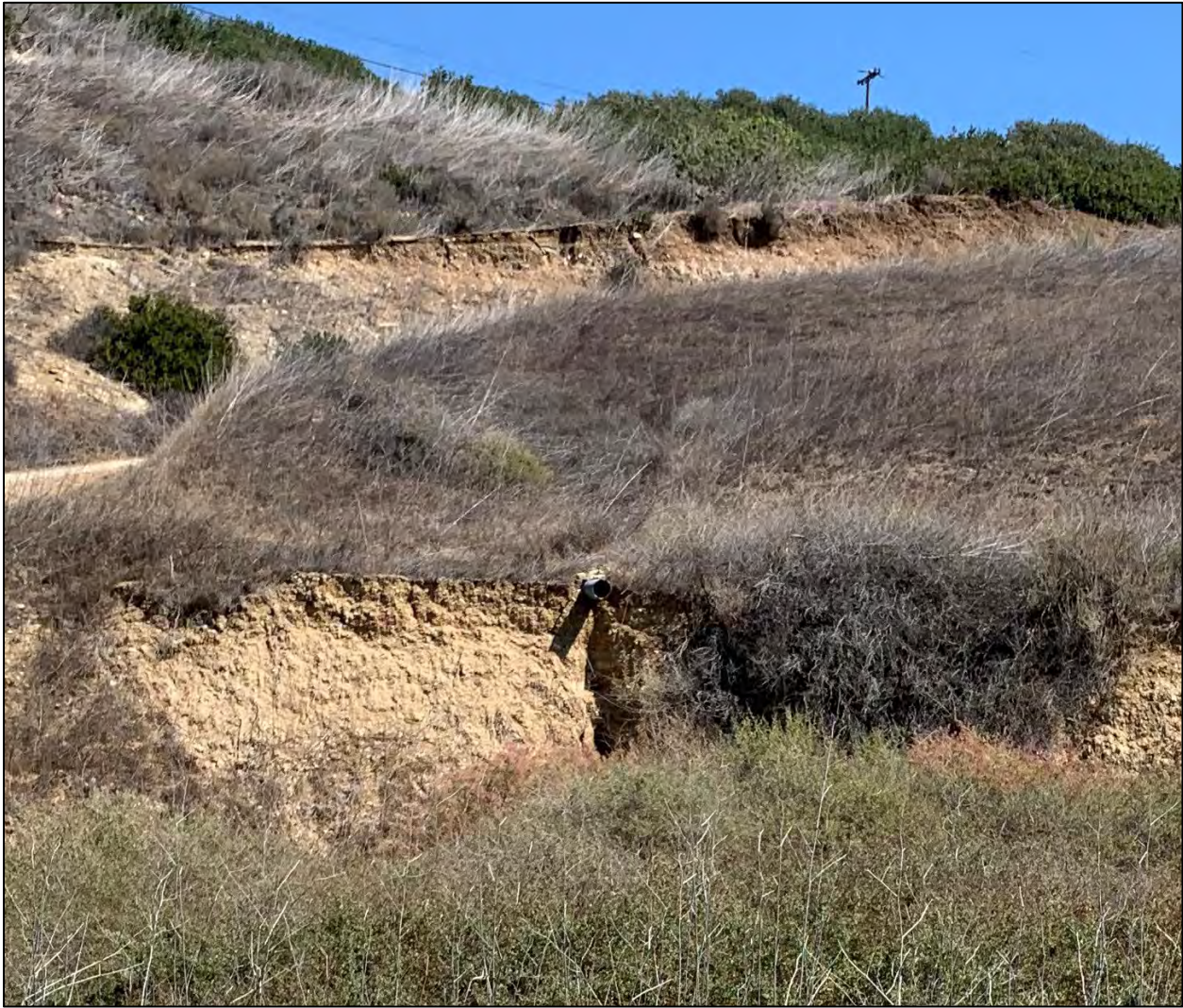
Figure H-2: Culvert or water conveyance along the north flank scarp draining into the Portuguese Bend Landslide.
