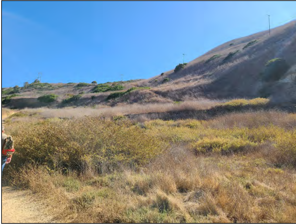
Photograph 3. View of the eastern portion of slide complex.
