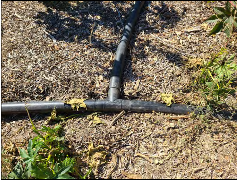
Photograph 5. Fused High-density Polyvinyl Ethylene (HDPE) pipe for dewatering well system.
