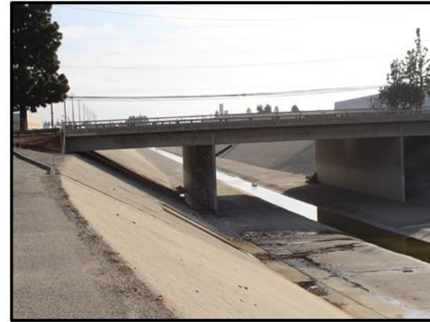
PHOTO 6: View looking east of the Valley View bridge over Coyote Creek.
