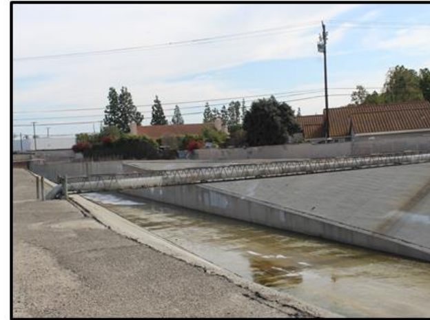
PHOTO 18: View looking northeast of a gas utility pipeline.
