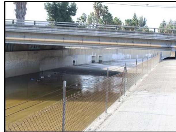
PHOTO 8: View looking south of the Artesia Boulevard bridge over Coyote Creek.
