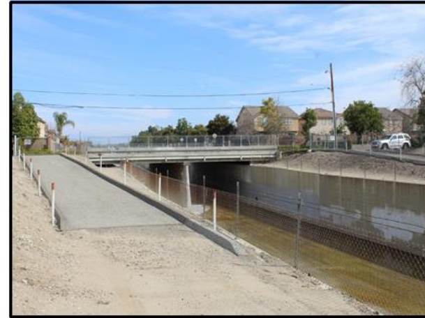
PHOTO 22: View looking northeast at La Mirada Boulevard.
