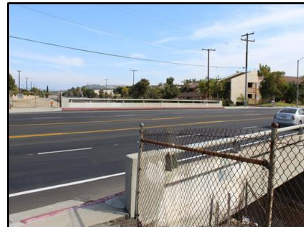
PHOTO 20: View looking northeast of Stage Road.
