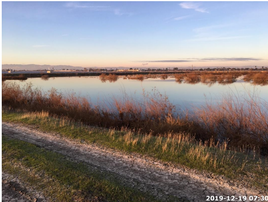
Photograph 15. Wastewater treatment pond northwest of site, looking northwest.
