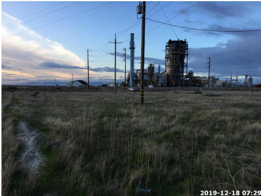
Photograph 2. Old power plant off southwest corner of site.
