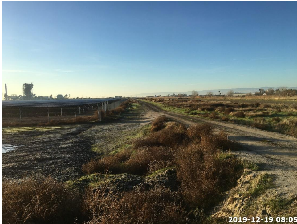
Photograph 17. Looking south along west side of solar farm.
