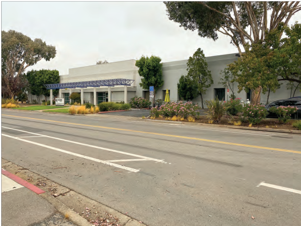
Photo 6: Light industrial building west of the project site, as seen from Jefferson Drive
