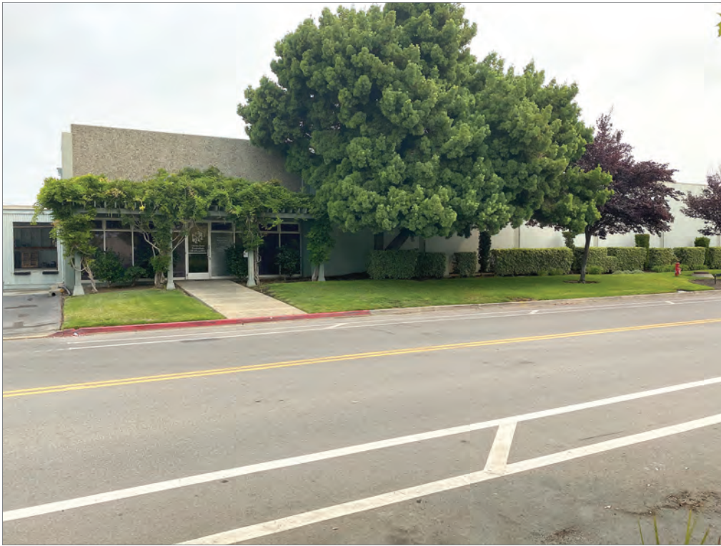
Photo 1: Existing building, as seen from Jefferson Drive
