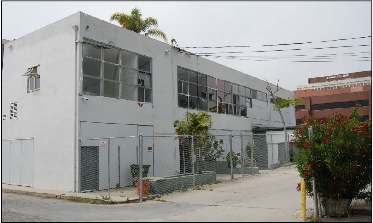
Barry Building, north façade, view looking southwest.
