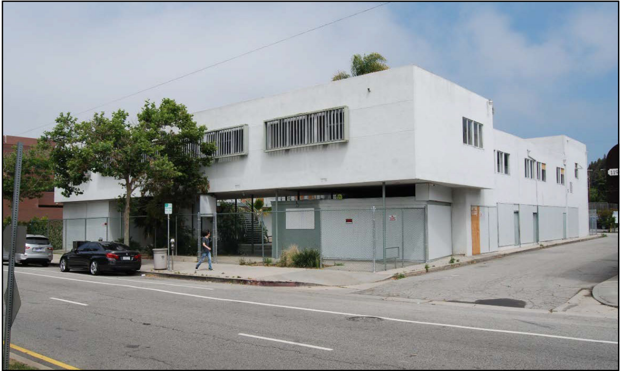
Barry Building, exterior, view of south and east façades looking northwest.
