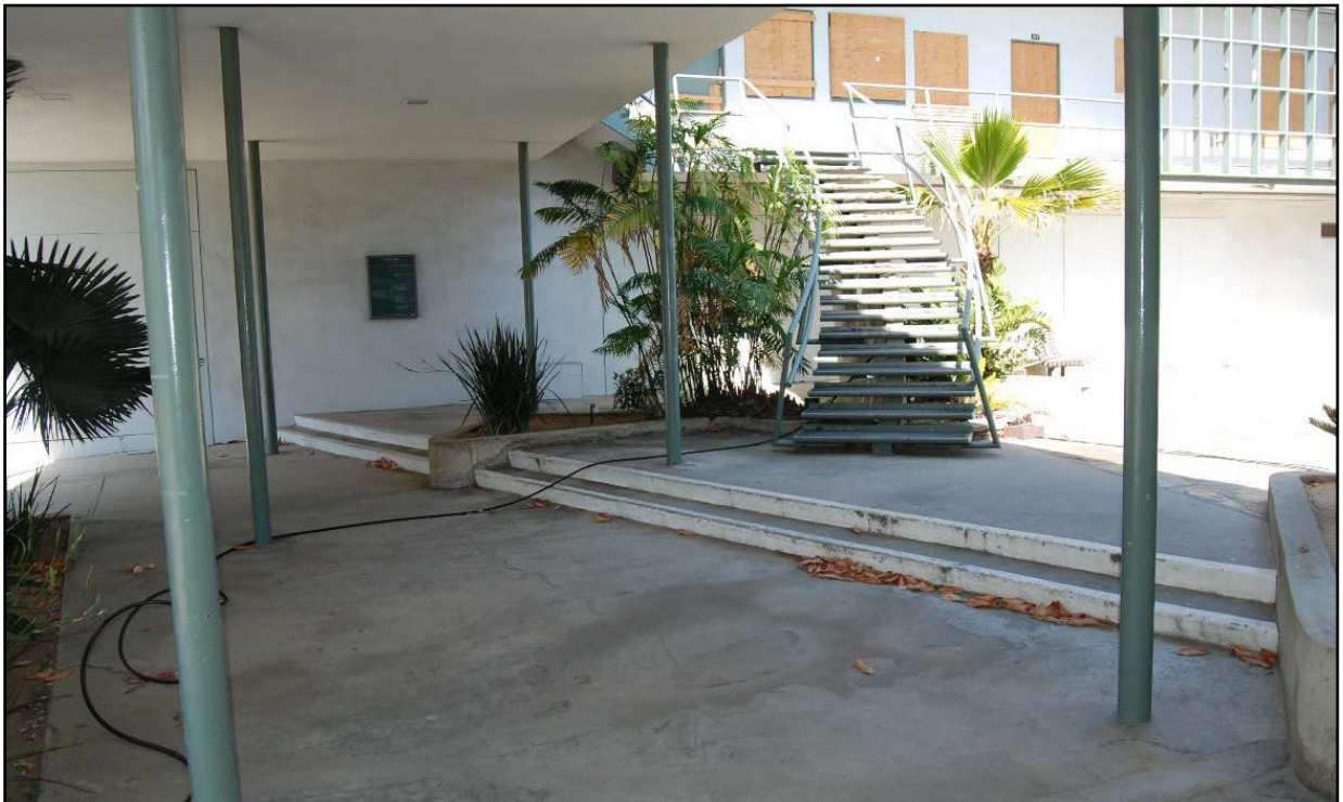
Barry Building, view looking northwest of courtyard entrance.
