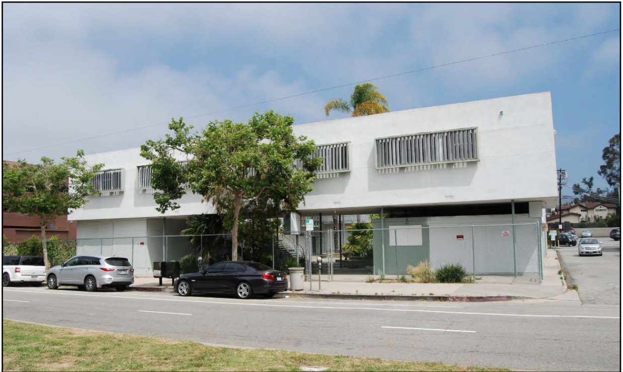
Barry Building, south façade, view looking northwest.
