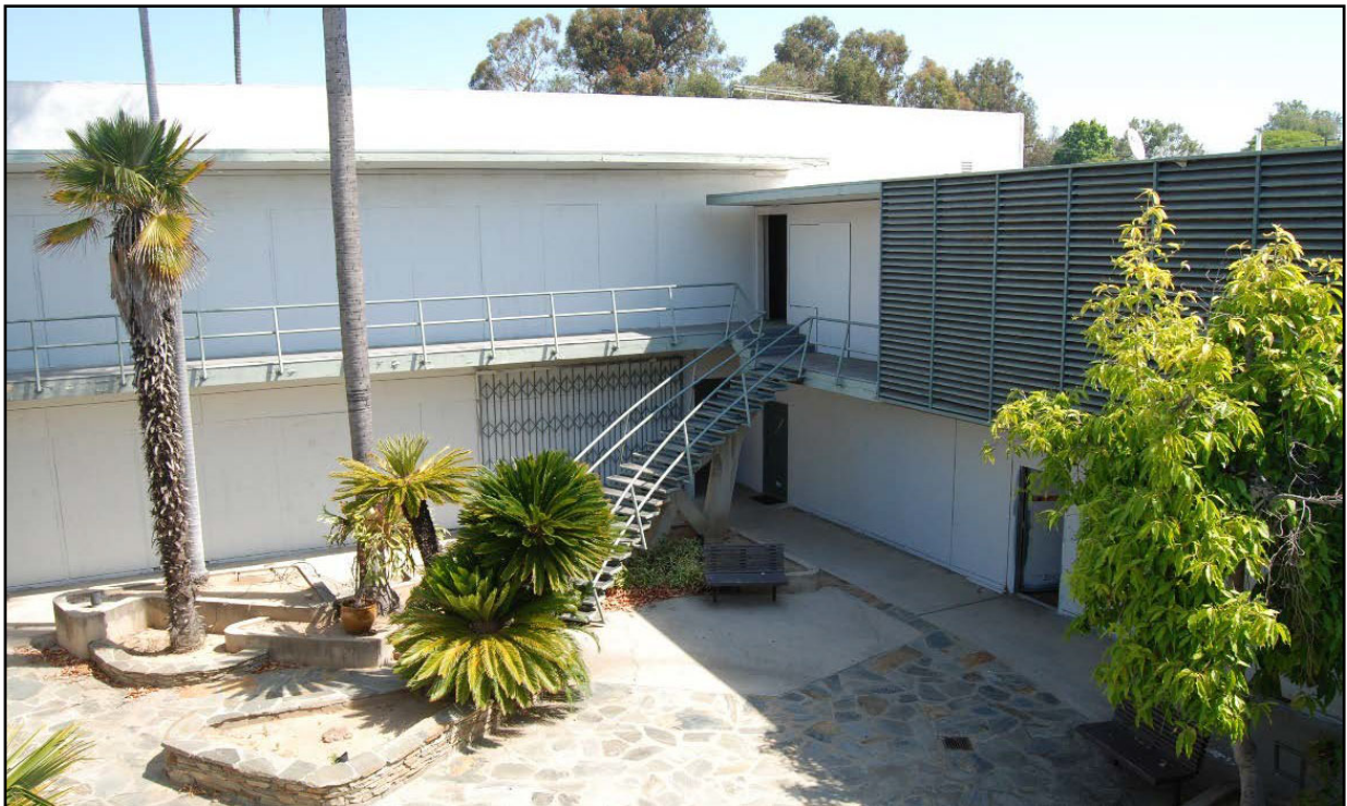
Barry Building, courtyard, view looking northeast.
