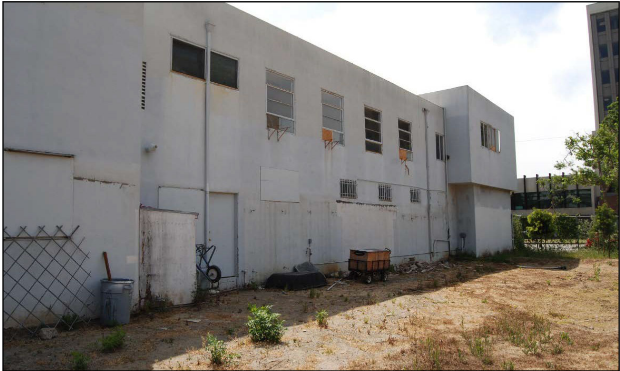
Barry Building, west façade, view looking southeast.
