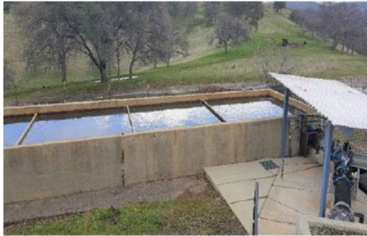
Photo 3 - Headworks (inlet pipe and flocculation basin)
