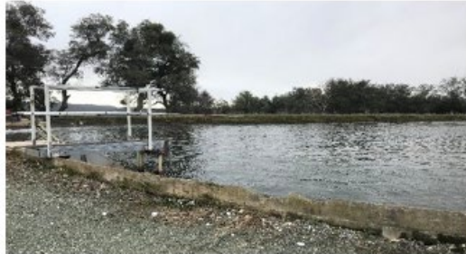
Photo 2 - Forebay Inlet to WTP Upper Plant
