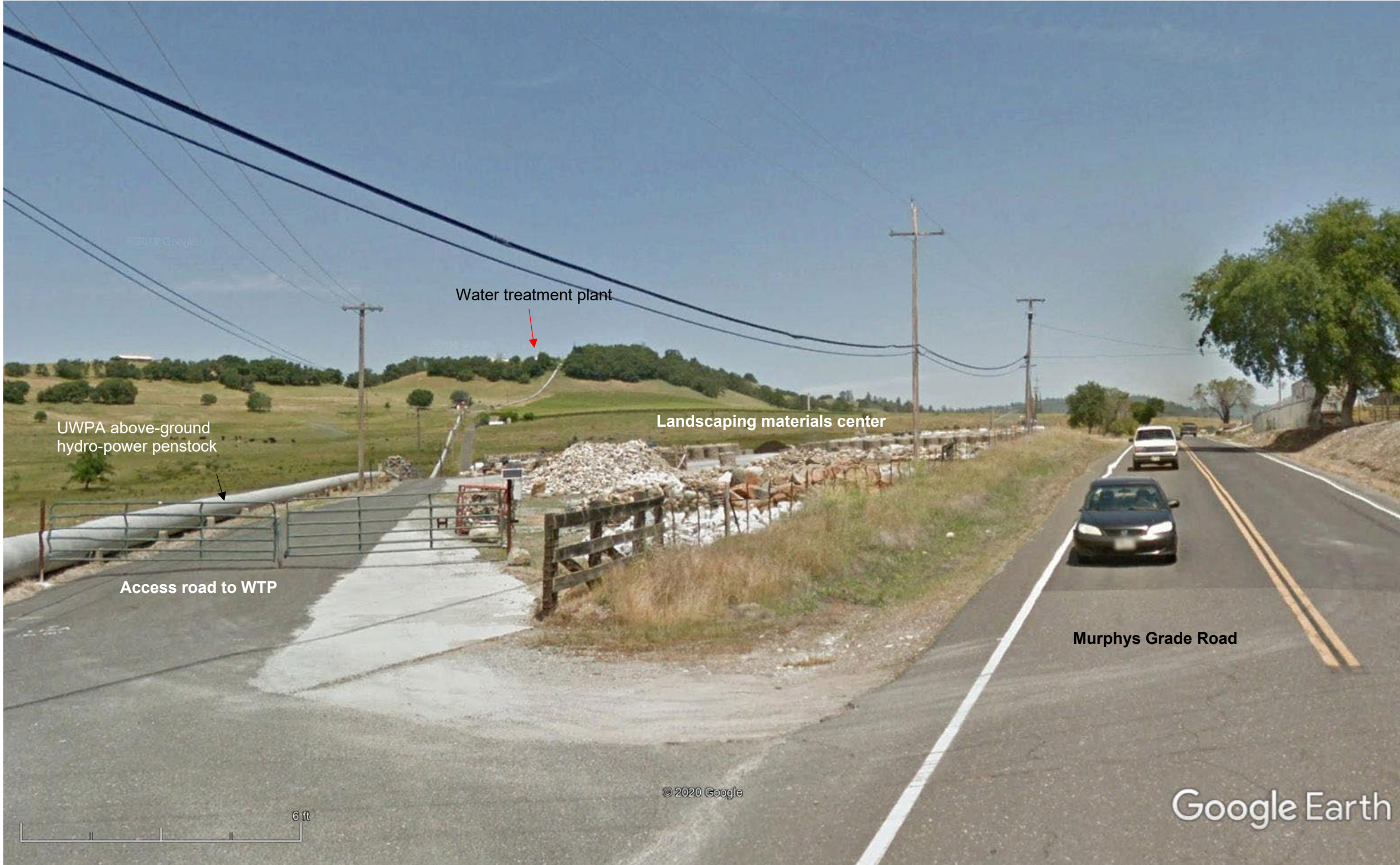
Figure 11: View of Water Treatment Plant from Murphys Grade Road Project Entrance
