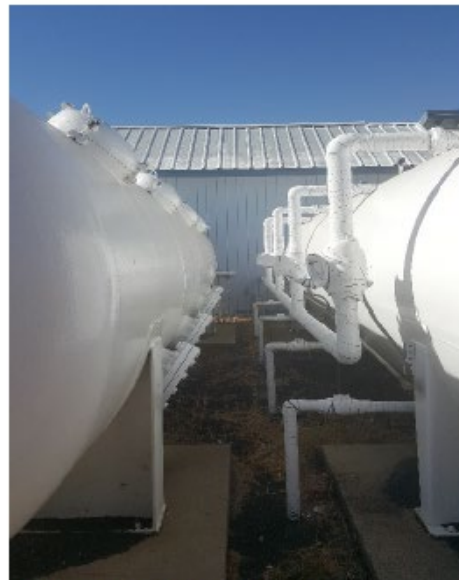
Photo 9 - Two of three filter vessels
