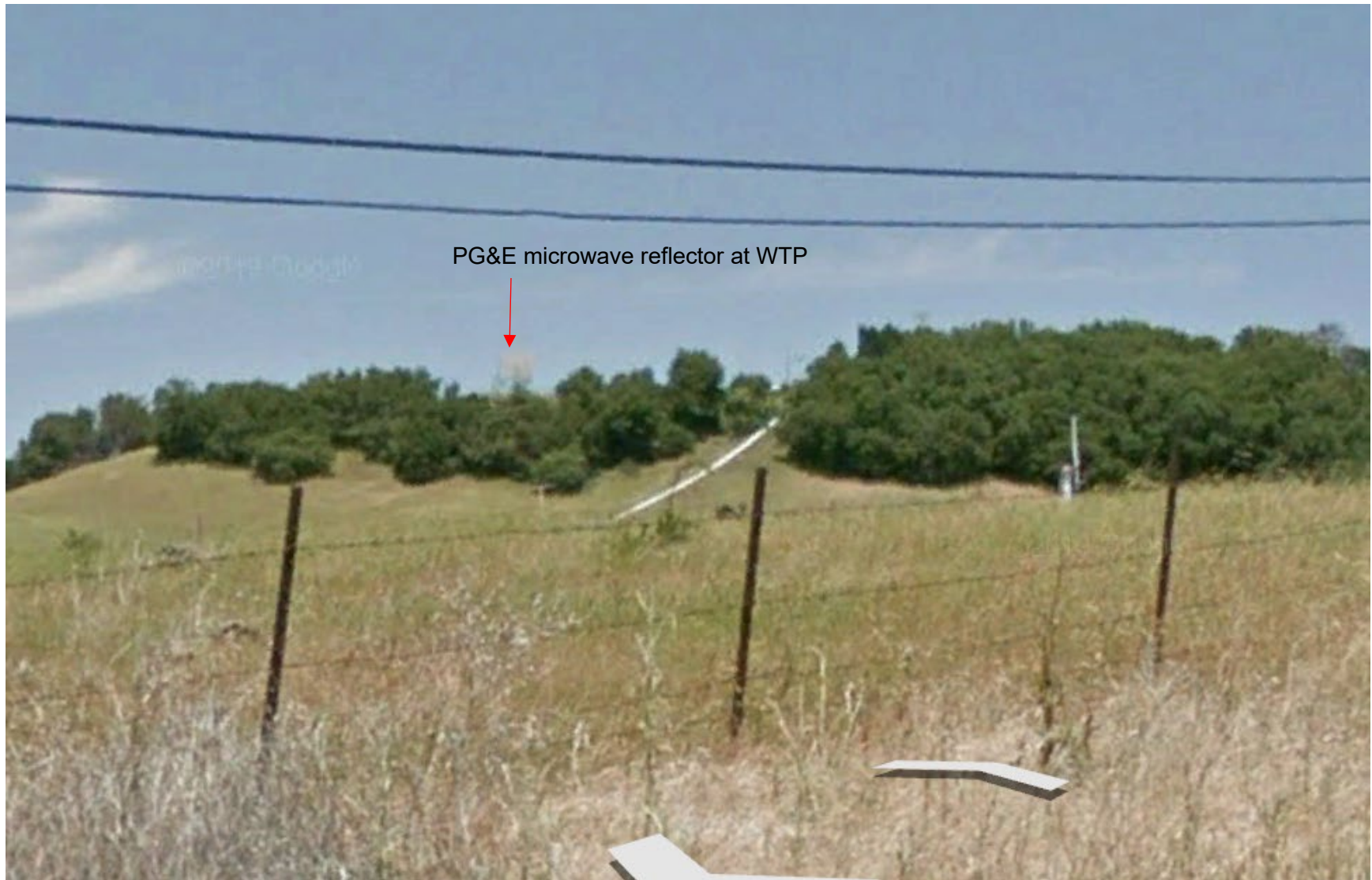
Figure 12: PG&E Microwave reflector at WTP visible from Murphys Grade Road
