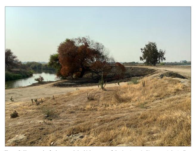
**Figure 6**. Photograph of a berm and the high terrace of the San Joaquin River near Lake Joallan (visible at far right), looking south, showing breaches in the berm that do not provide adequate flood protection for the City.
