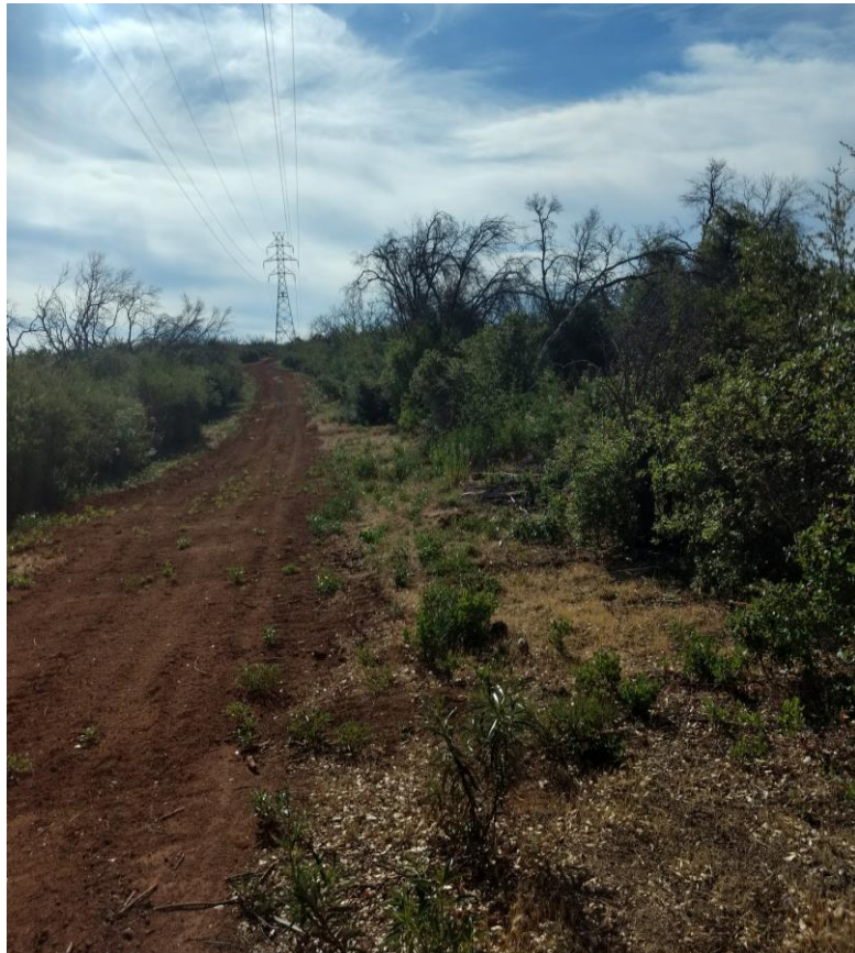
Figure 2. Proposed Tower Site, located 200 feet northeast of an existing 76 foot Electrical Tower
