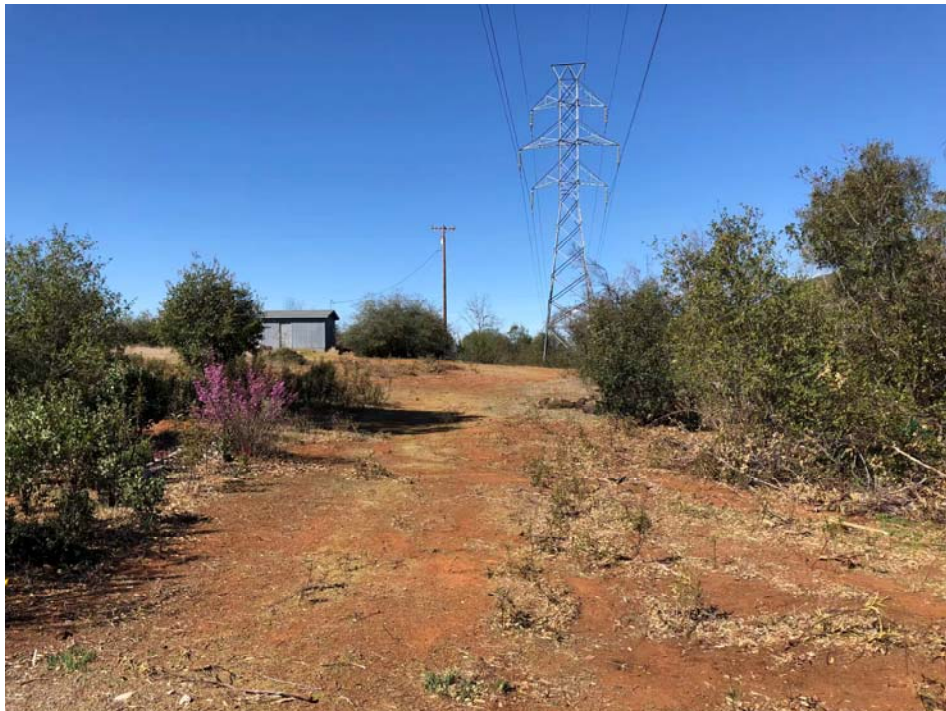
Existing access road and proposed route for power and fiber-optic cable. Proposed power and fiber-optic cable will be attached to existing wood pole in center of photo.
